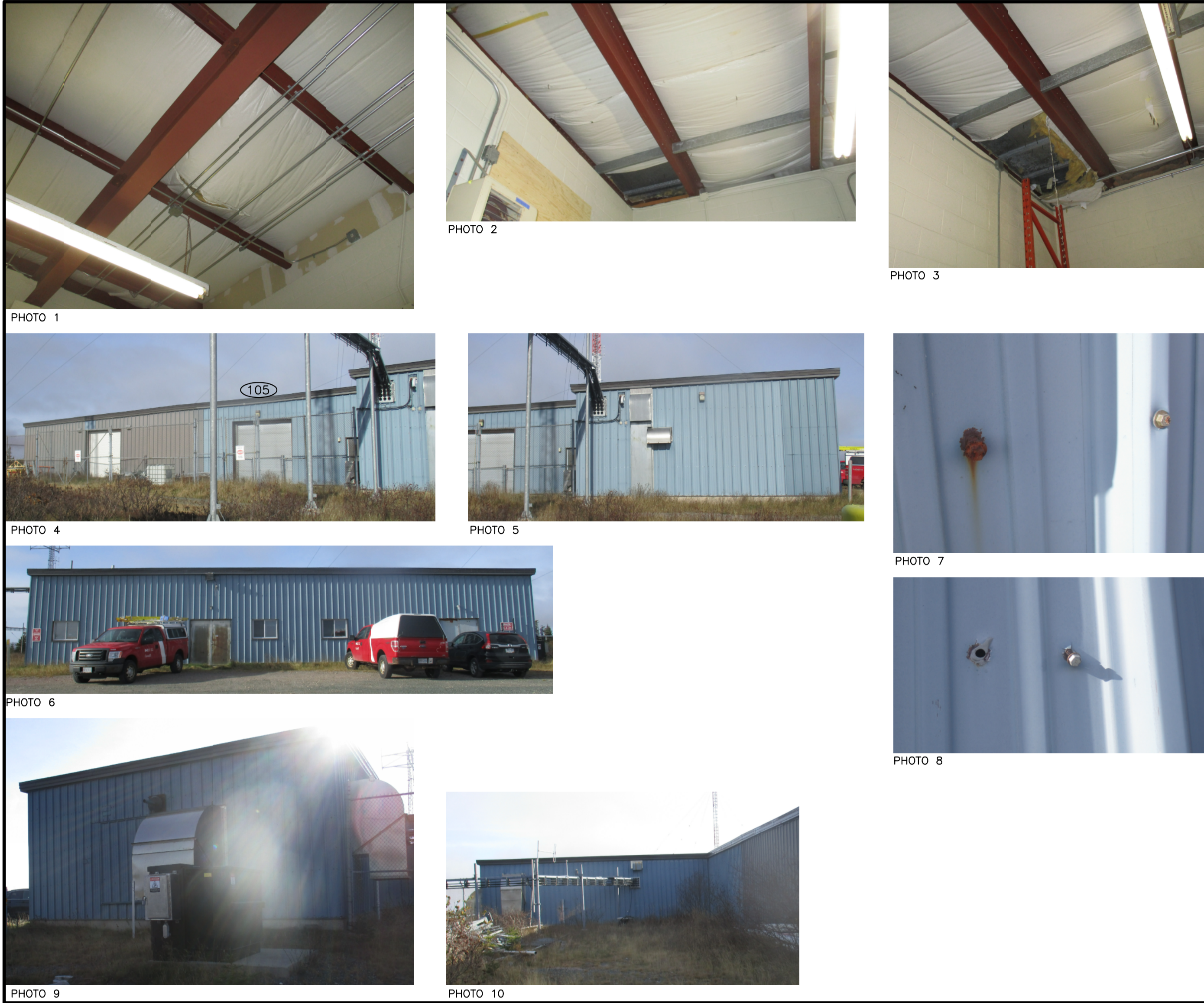
5 PHOTOS - EXISTING CONDITIONS
