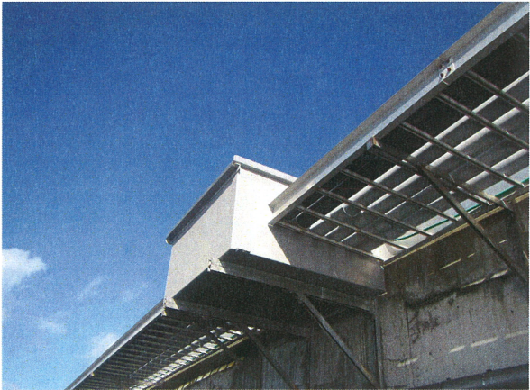
⑦ JUNCTION PULL BOX ALONG CABLE TRAY
