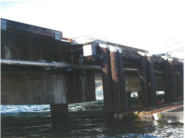
23 GLULAM WALE AND TIMBER FENDER PILE GROUPS AT BERTH Y3
