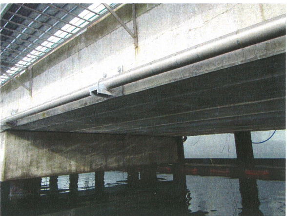
⑪ SEWER FORCE MAIN TYPICAL PIPE SUPPORT
