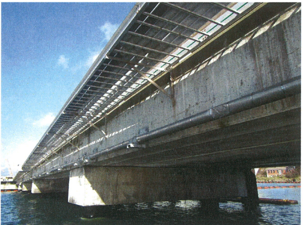
20 ELECTRICAL CABLE TRAY AND SEWER FORCE MAIN
