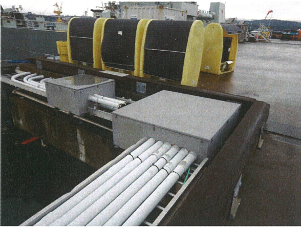
⑤ PULLBOXES AT JETTY TRESTLE INTERFACE WITH WHARF HEAD
