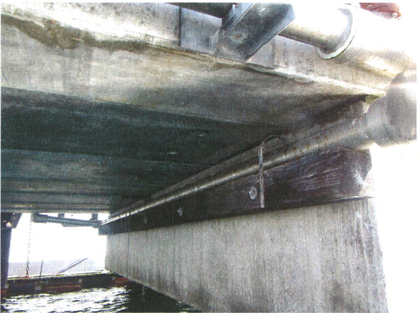
24 UNDER PIER UTILITY SUPPORT AND HANGING ANODE STRING
