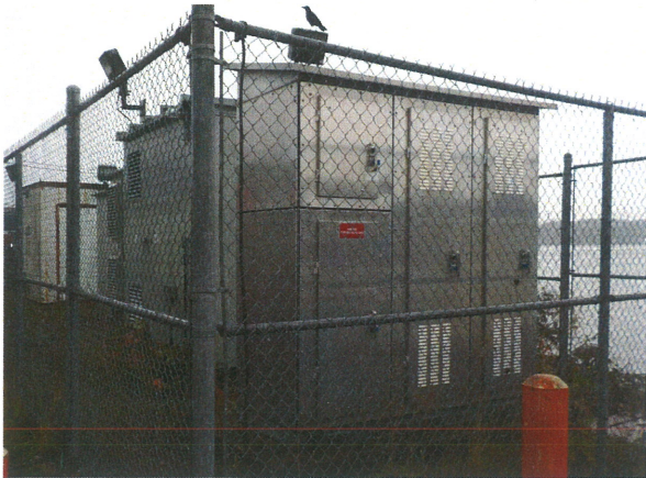
① 12.47 kV / 480 V UNIT SUBSTATION
