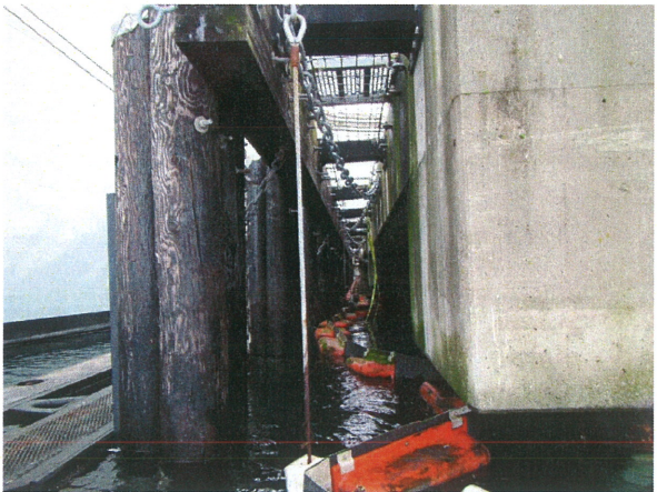
16 TYPICAL FENDER PILE GROUP, GLULAM WALE AND BARRIER BOOM
