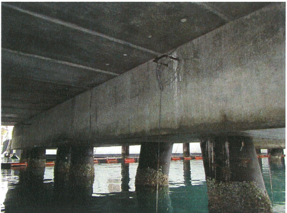
19 CATHODIC PROTECTION ANODES HANGING FROM WHARF HEAD PILE CAP
