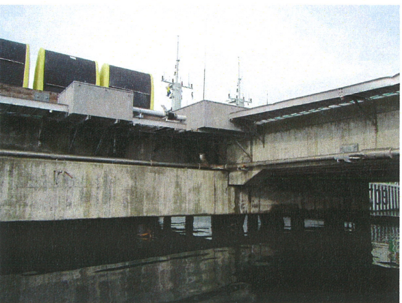
⑫ PULLBOXES AT JETTY TRESTLE INTERFACE WITH WHARF HEAD - FROM WATER
