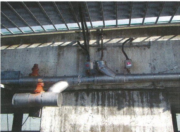
⑩ HEAT TRACE SYSTEM FOR WATER PIPES
