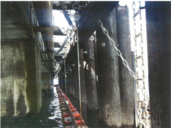
21 TYPICAL BERTH Y1 FENDER SYSTEM AND UTILITIES
