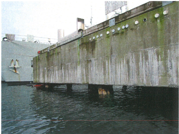
14 EMBEDDED CONDUITS CAPPED AT WHARF HEAD
