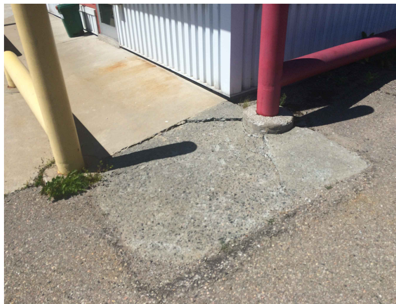
7 AREA OF CONCRETE REPAIR A-B01/ APPROXIMATELY 3M 2 AREA
