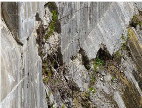
Vegetation growing in wall, very severe spalling, and alkali-aggregate reaction on north downstream weir wall.
