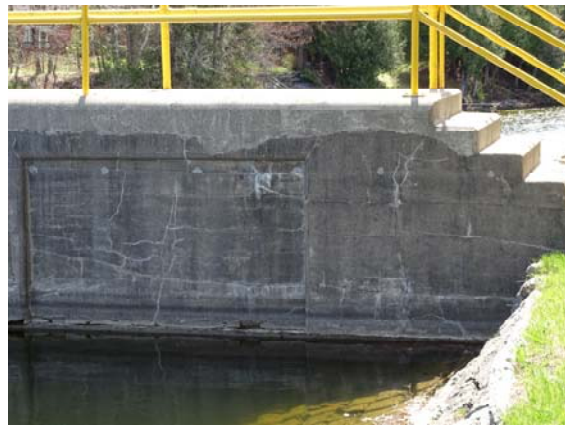
Alkali-aggregate reaction on north abutment.
