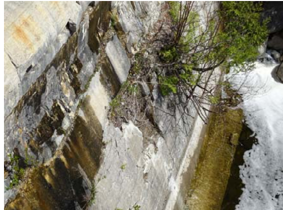
Tree growing out of downstream face of South Weir and water stains from seepage through wall.
