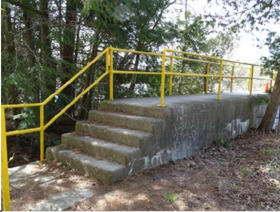
Alkali-aggregate reaction at South Abutment.
