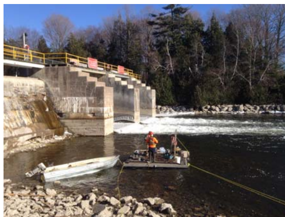
Portable coring on raft.
