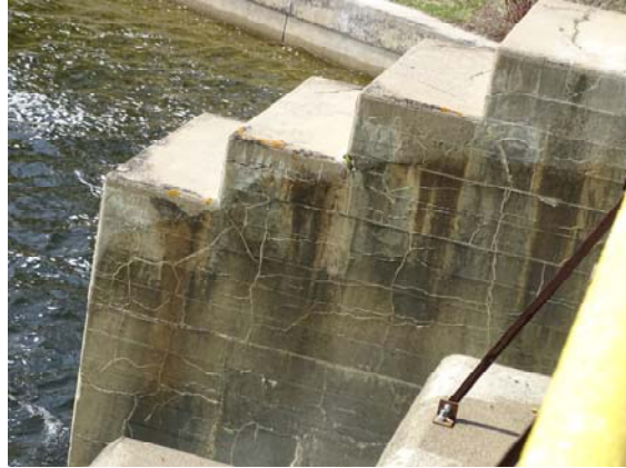
Severe alkali-aggregate reaction.
