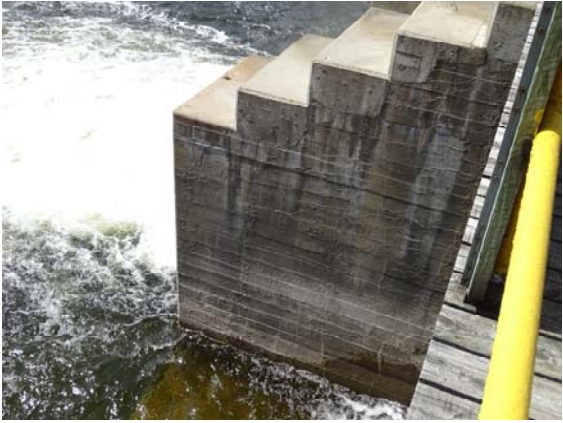
Downstream middle pier showing alkali-aggregate reaction.
