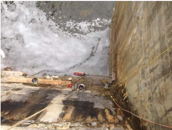
Horizontal coring of downstream pier.
