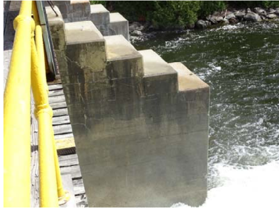
Downstream middle pier showing alkali-aggregate reaction.
