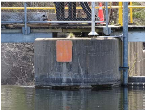
Upstream face of north pier with cracking and spalling at waterline.
