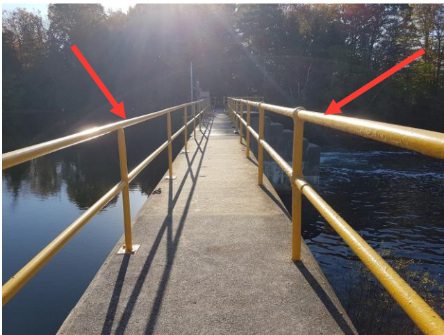
Photo #3: View of lead-containing yellow paint on railings throughout the subject area.
