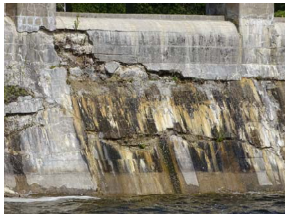
Water seepage, very severe spalling, wide cracks and alkali-aggregate reaction on north downstream weir wall.
