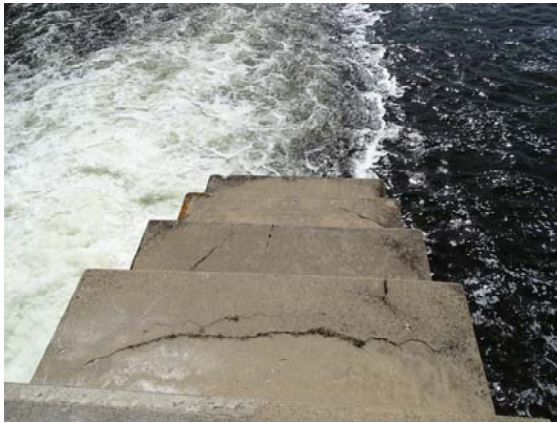
Wide grass filled crack at top of downstream face.
