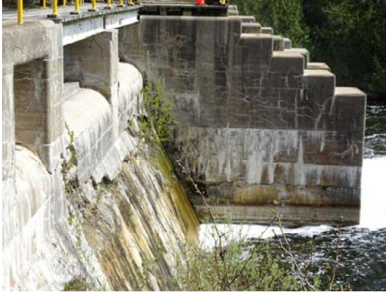
Severe alkali-aggregate reaction.
