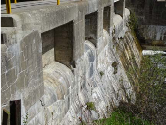
Alkali-aggregate downstream face of north weir wall and tree growing out of wall.
