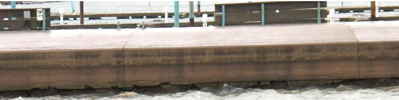
Small Craft Harbours, Fisheries and Oceans Canada, Central and Arctic Region Photo 42, Concrete Coping Above Water, See photo 32 Station 0+420 to 0+400 Port Dalhousie - East Pier (Channel Side) December 2014
