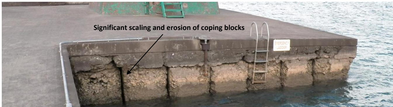
Small Craft Harbours, Fisheries and Oceans Canada, Central and Arctic Region Photo 47, Concrete Coping Above Water Station 0+665 Port Dalhousie - East Pier (Lake Side) December 2014
