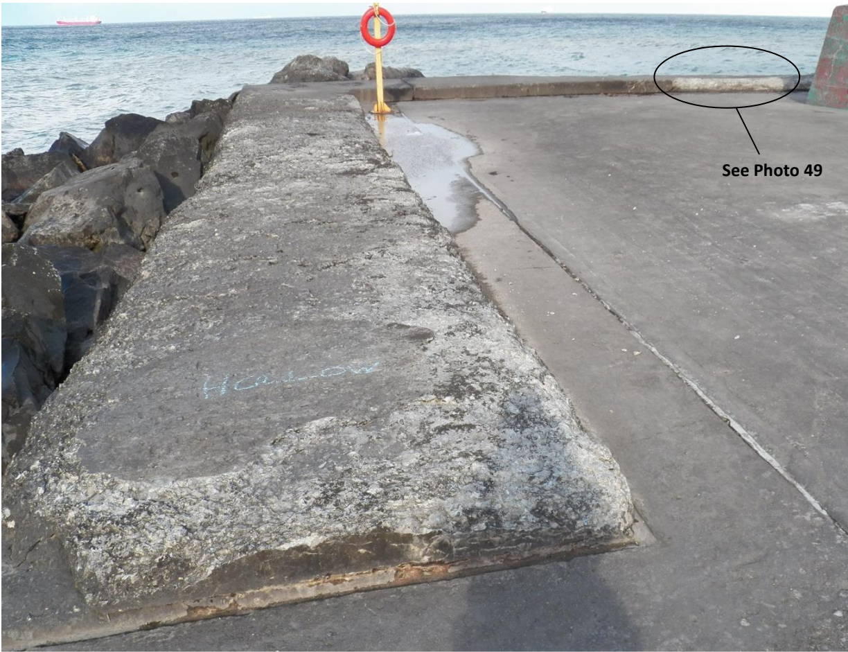
Small Craft Harbours, Fisheries and Oceans Canada, Central and Arctic Region Photo 48, Delaminated Surface, Concrete Deck Station 0+665 Port Dalhousie - East Pier December 2014
