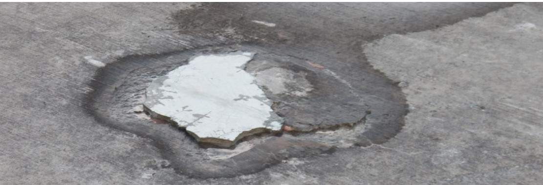
Small Craft Harbours, Fisheries and Oceans Canada, Central and Arctic Region Photo 44, Delaminated Surface, Concrete Deck Station 0+235 Port Dalhousie - East Pier December 2014
