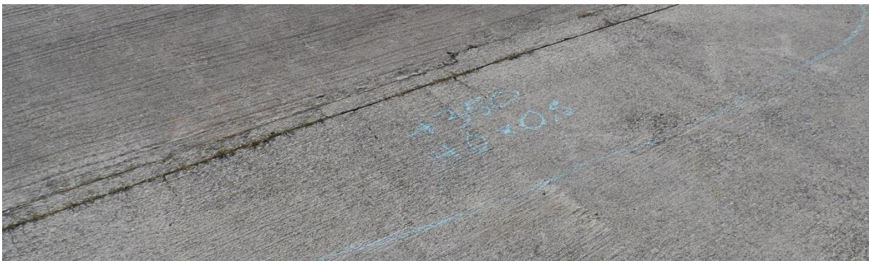
Small Craft Harbours, Fisheries and Oceans Canada, Central and Arctic Region Photo 45, Delaminated Surface, Concrete Deck Station 0+350 Port Dalhousie - East Pier December 2014
