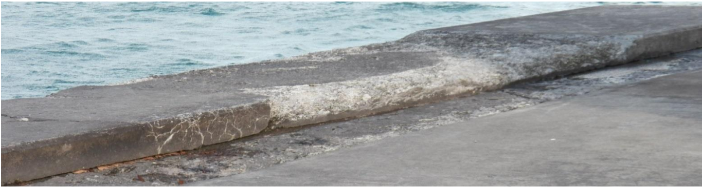
Small Craft Harbours, Fisheries and Oceans Canada, Central and Arctic Region Photo 49, Delaminated Surface, Concrete Deck Station 0+681 Port Dalhousie - East Pier December 2014
