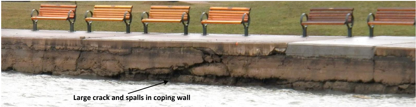
Small Craft Harbours, Fisheries and Oceans Canada, Central and Arctic Region Photo 43, Concrete Coping Above Water, See photo 36 Station 0+240 to 0+230 Port Dalhousie -East Pier (Channel Side) December 2014
