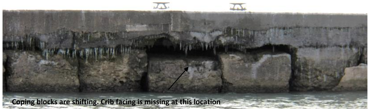
Small Craft Harbours, Fisheries and Oceans Canada, Central and Arctic Region Station 0+520 Photo 20, Close up – See Photo 4 Port Dalhousie - West Pier (Channel Side) December 2014
