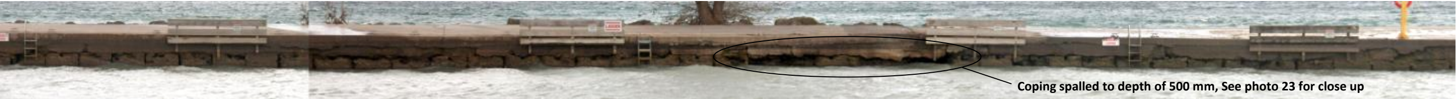
Small Craft Harbours, Fisheries and Oceans Canada, Central and Arctic Region Station 0+315 to 0+365 Photo 8, Concrete Coping Above Water Port Dalhousie, ON - West Pier (Channel Side) December 2014
