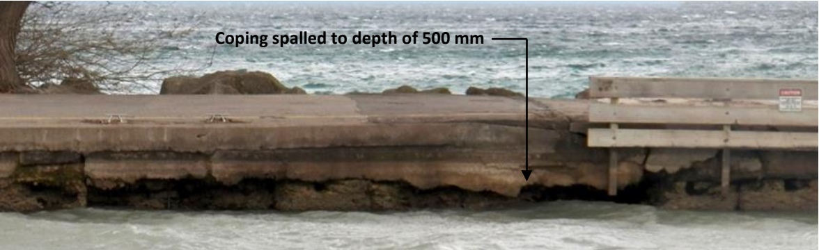
Small Craft Harbours, Fisheries and Oceans Canada, Central and Arctic Region Station 0+335 Photo 23, Concrete Coping – See Photo 8 Port Dalhousie - West Pier (Channel Side) December 2014
