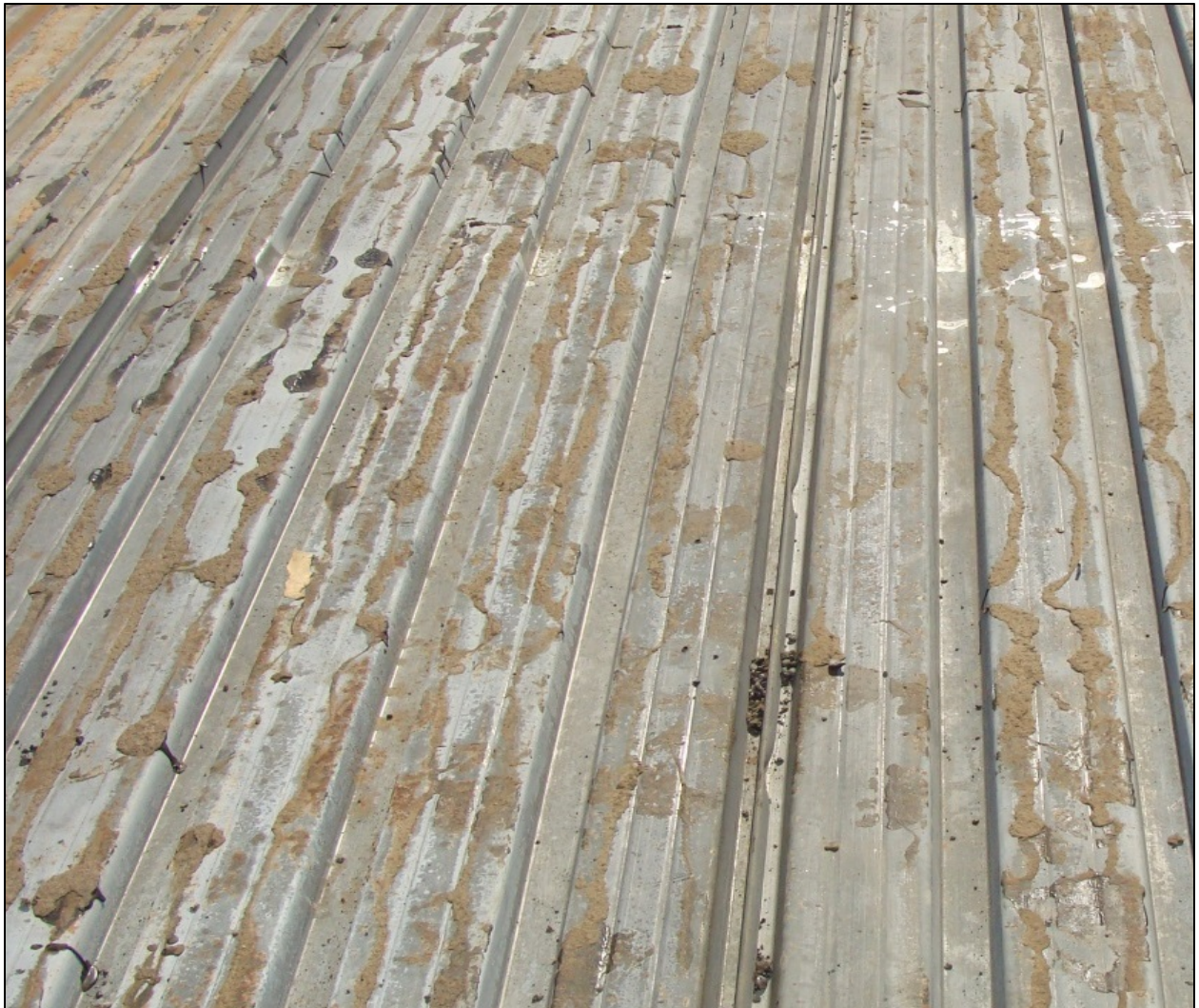
Photo of Level 1: No Visible Corrosion
