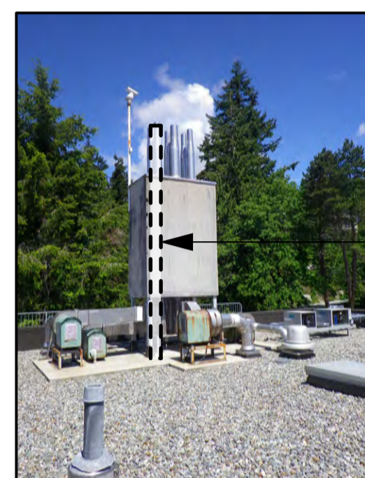
NEW EXHAUST SECURED TO EXTERIOR OF (E) TOWER
