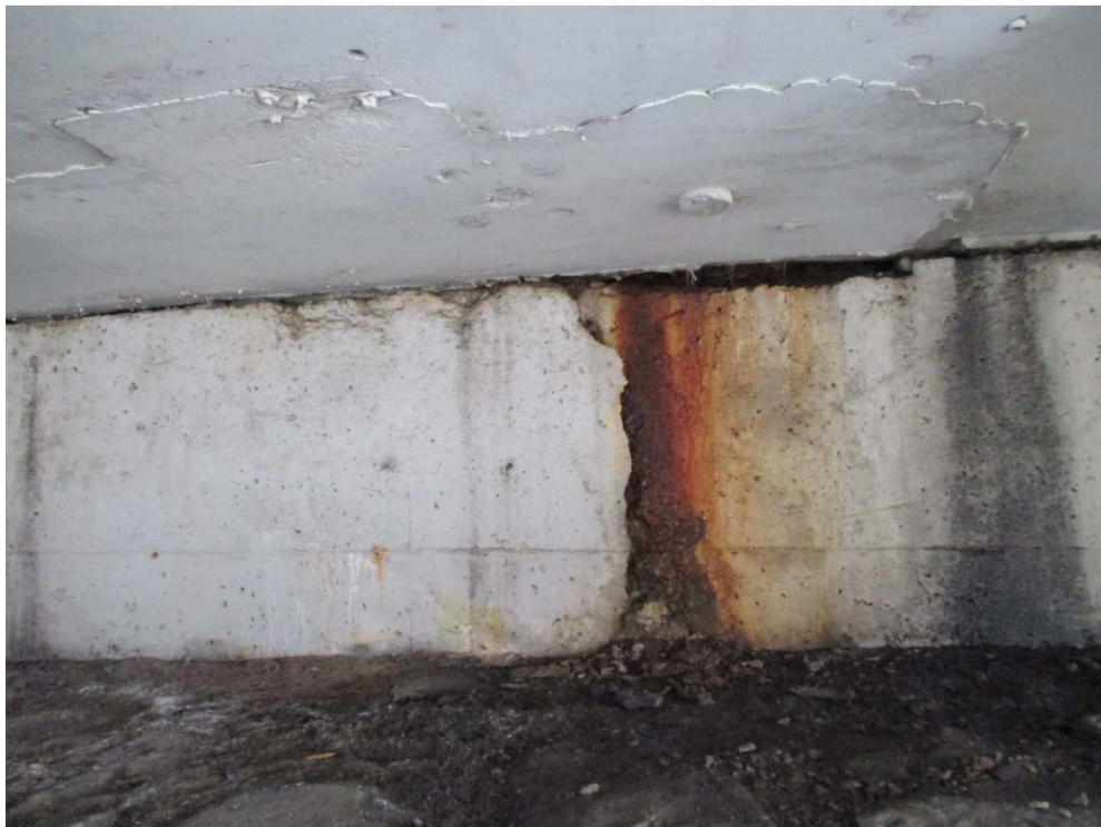
Photo 6: Delamination in the east abutment
