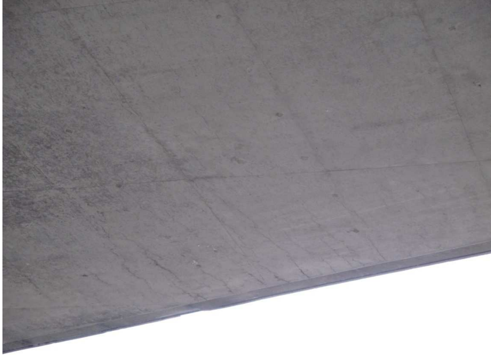
Photo 3: Light cracks in the soffit of bridge deck
