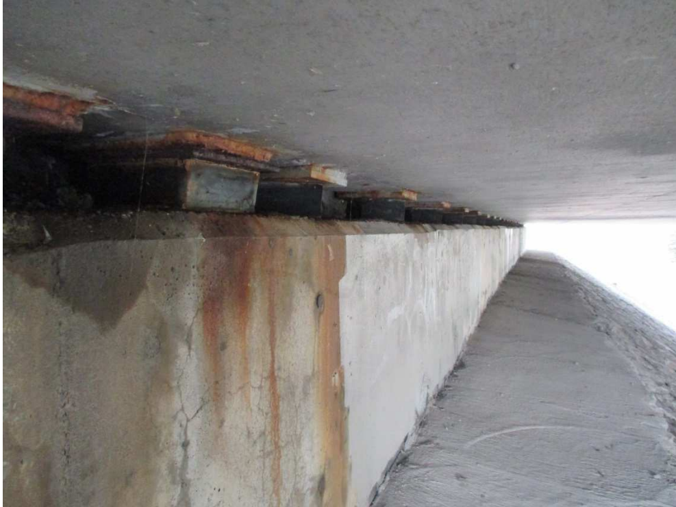
Photo 7: leaking water and rusted steel plates
