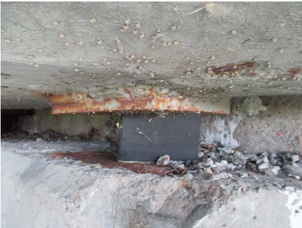
Photo 8: Horizontal cracks in elastomeric in bearing
