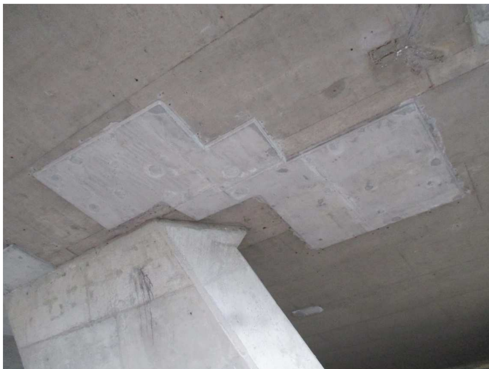
Photo 6: Overbuilt patches in the bridge deck
