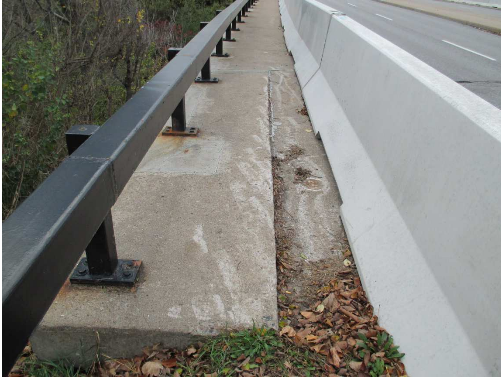
Photo 13: Settlement of approach slab
