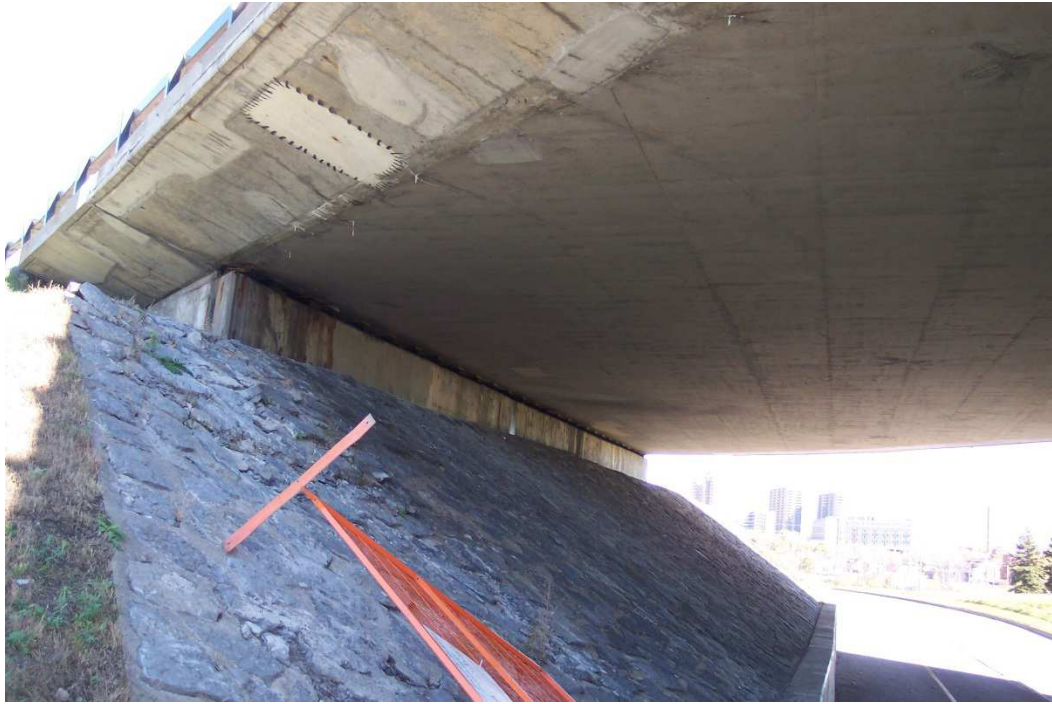
Photo 15: Loose stones in embankment
