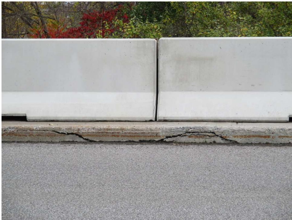
Photo 10: Cracks in curb
