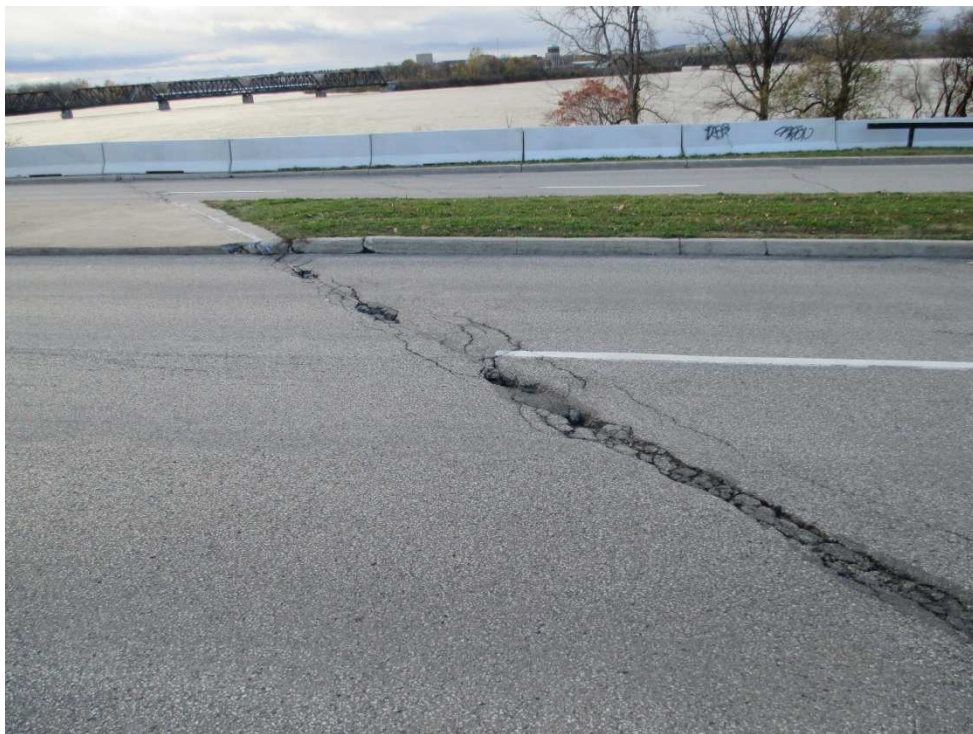
Photo 12: Severe cracks in asphalt at expansion joint
