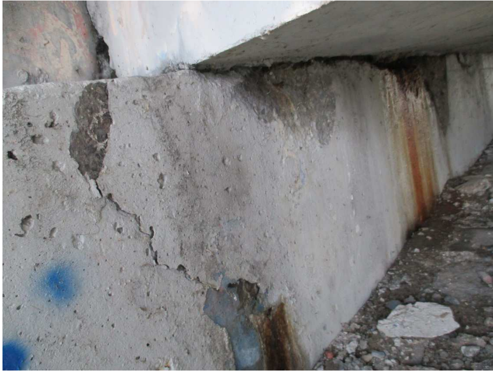
Photo 5: Delamination in the east abutment
