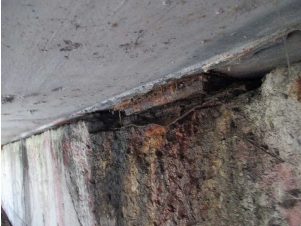
Photo 7: Spalling and leaking in west abutment
