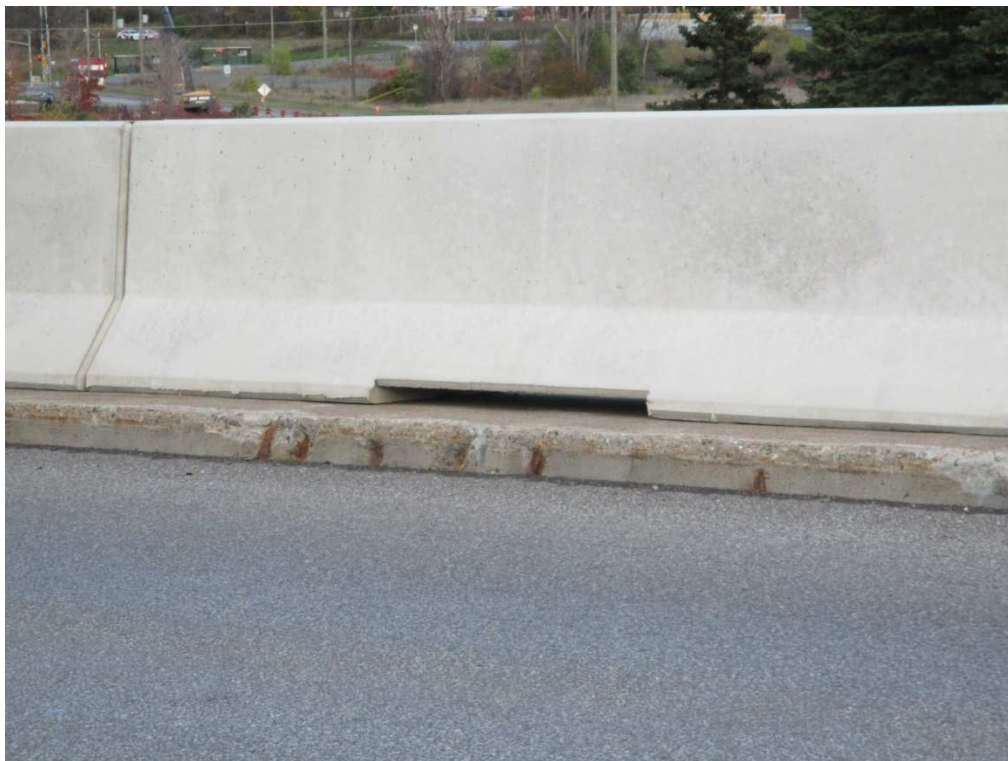
Photo 10: Spalling in curb
