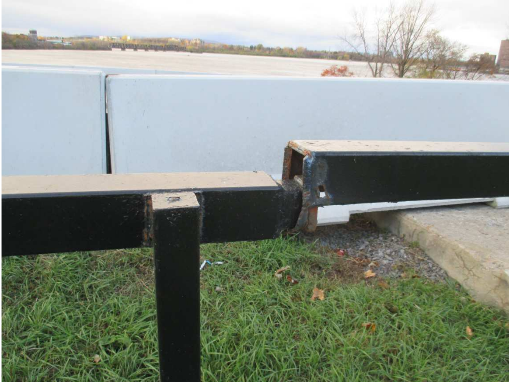
Photo 11: Corrosion and missing connection in railing
