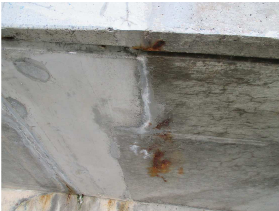
Photo 5: Corrosion of reinforcement in cantilever
