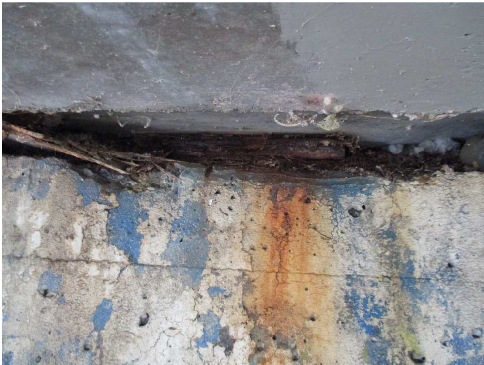
Photo 8: Severe corrosion in bearing
