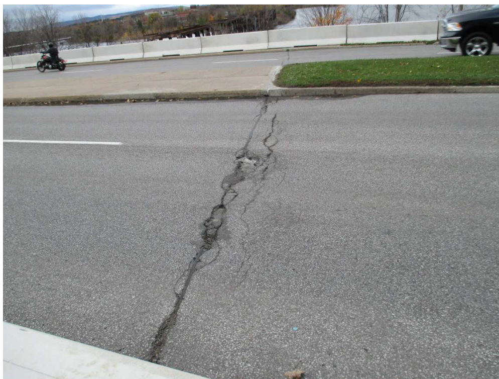
Photo 12: Severe cracks in asphalt at expansion joint
