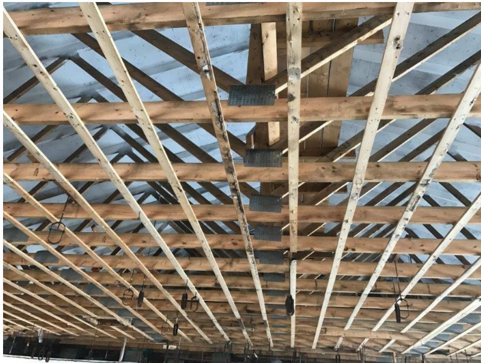
3 –View of Roof Structure
