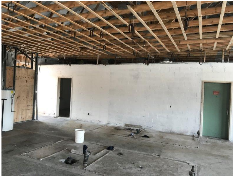
1 – Interior - View Towards Cell Block Area
