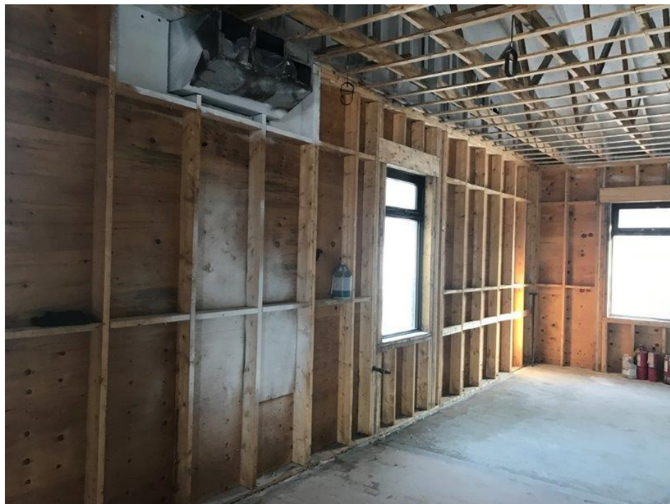
2 – Interior - View of Exterior Wall
