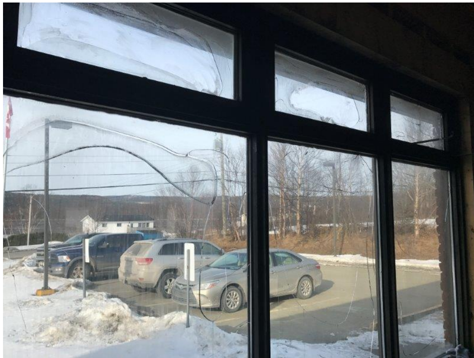
6 - Interior - View of Window
