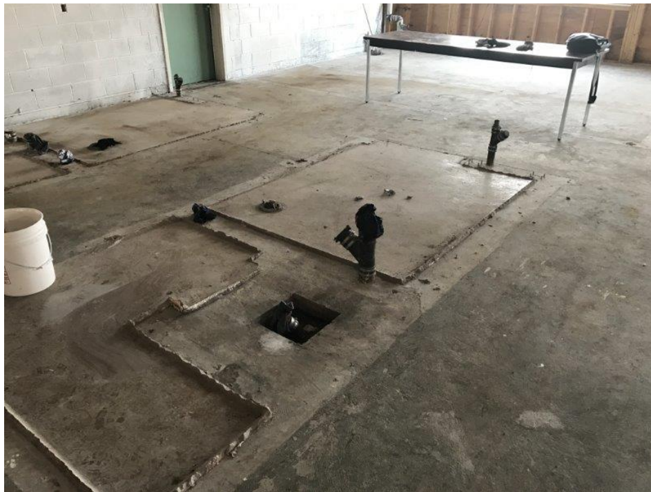
4–View of Floor Slab in Office Area
