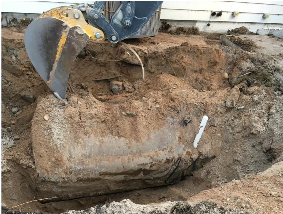
PHOTOGRAPH 5: Excavating around the UST to remove.
