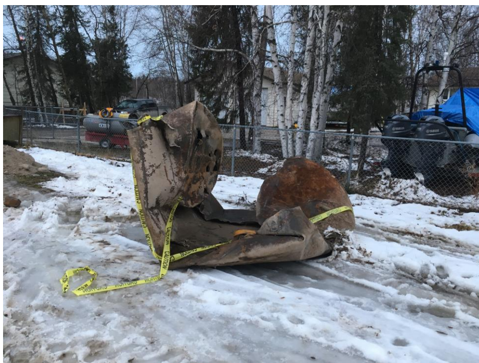
PHOTOGRAPH 8: Crushed UST waiting to be hauled to local landfill.
