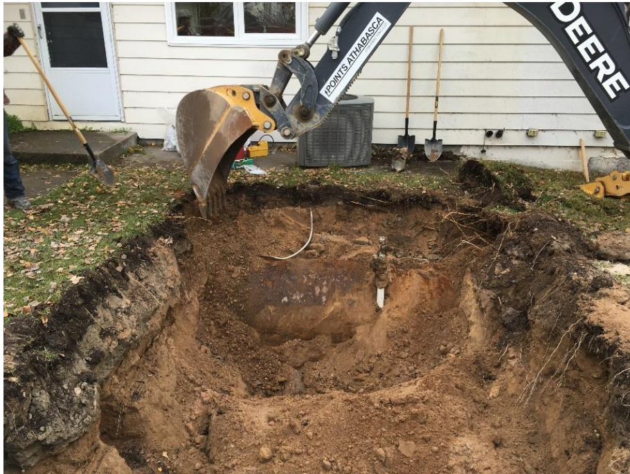
PHOTOGRAPH 3: Uncovering the UST during the initial excavation facing south.
