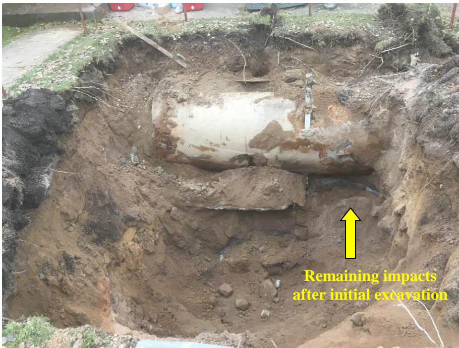
PHOTOGRAPH 4: View south at the exposed tank and concrete pad.
