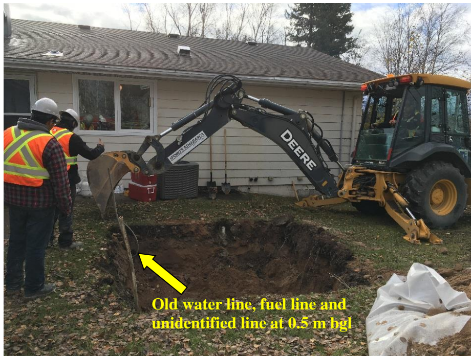
PHOTOGRAPH 2: Uncovering abandoned lines along the east wall of the excavation facing south.
