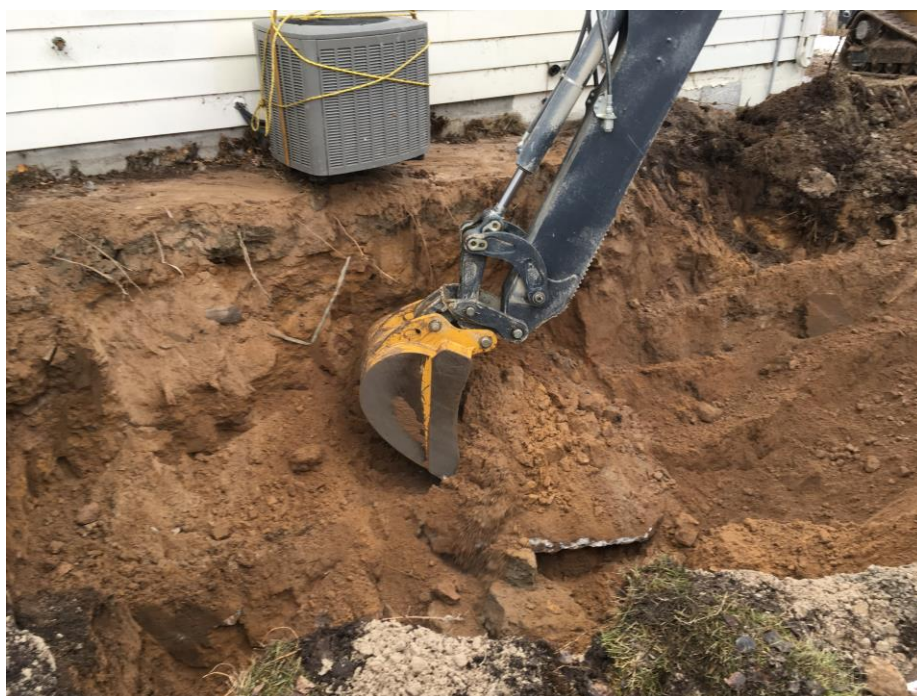
PHOTOGRAPH 7: Removing concrete pad the UST was situated on.
