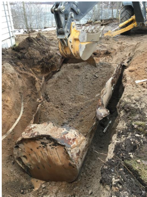
PHOTOGRAPH 6: Excavating soil out of the UST placed during the initial excavation.
