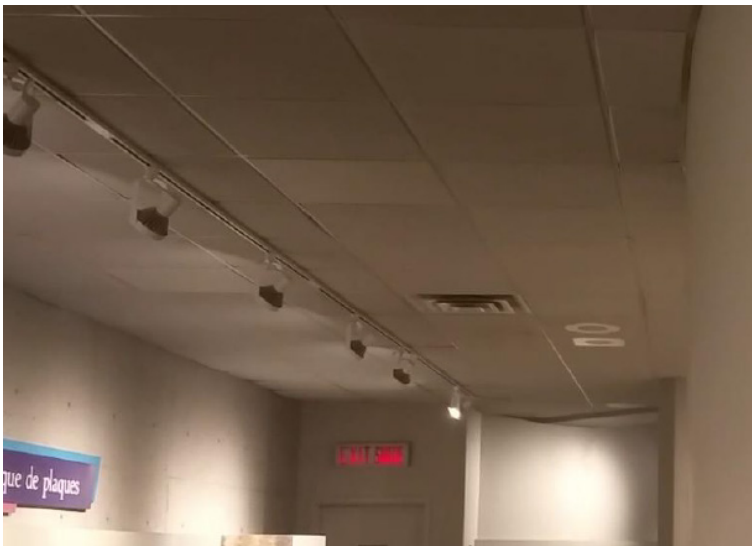
Air Supply grille in T-bar ceiling
