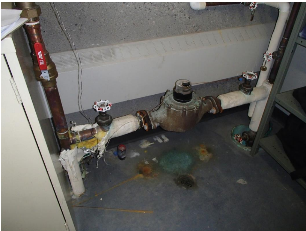
Photograph 25: Water Staining on Floor by Water Meter – Storage Room 1
