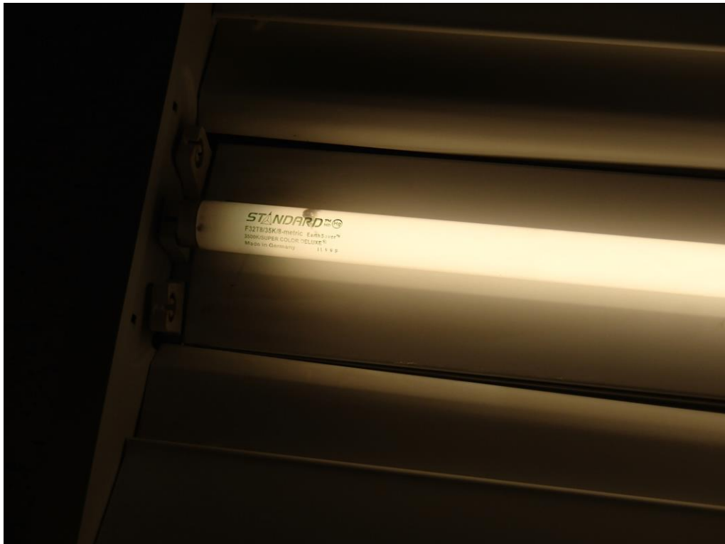
Photograph 12: Fluorescent Light Tube Observed Containing Mercury
