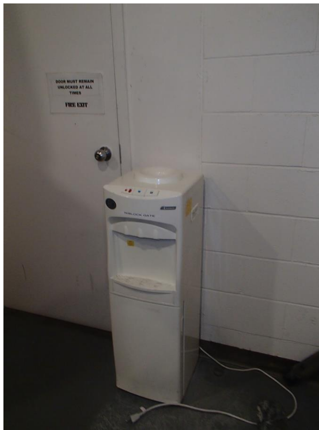
Photograph 19: Water Cooler Containing R-134a Located in the Corridor by the Mechanical Room
