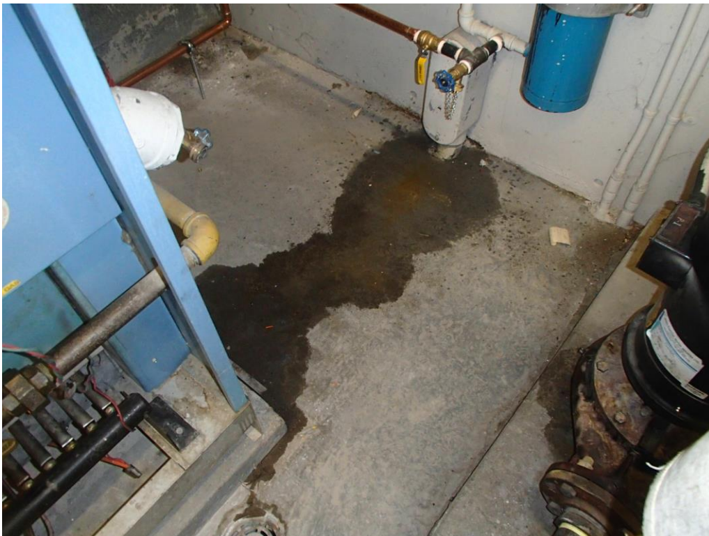
Photograph 23: Water Staining on the Floor – Mechanical Room
