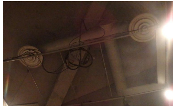
Exposed duct with Air grilles in the Theater
