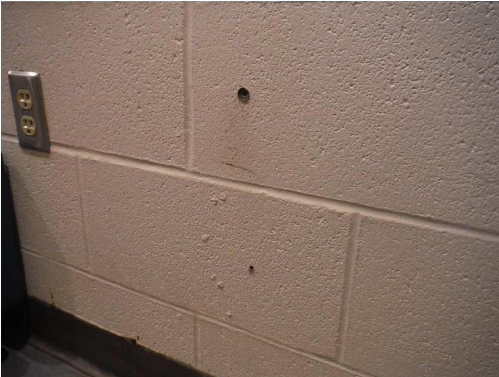
Photograph 05: Attempt to Drill into Cinderblock Wall for Vermiculite
