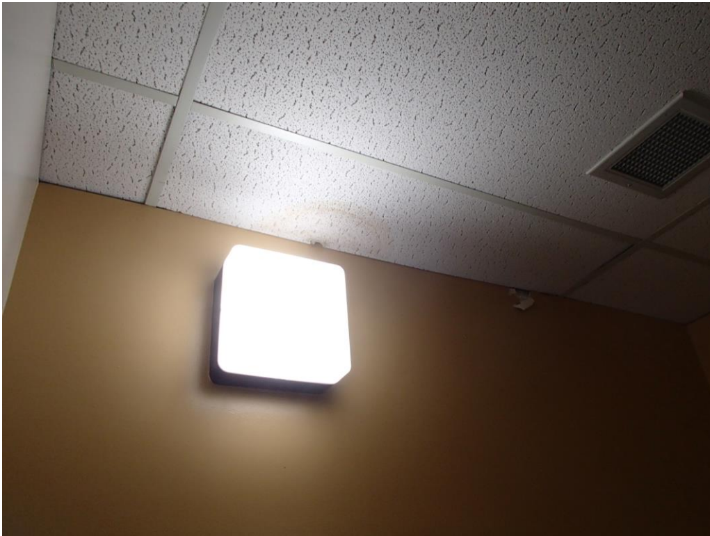
Photograph 26: Water Damage on Ceiling Tile in Washroom next to Kitchen
