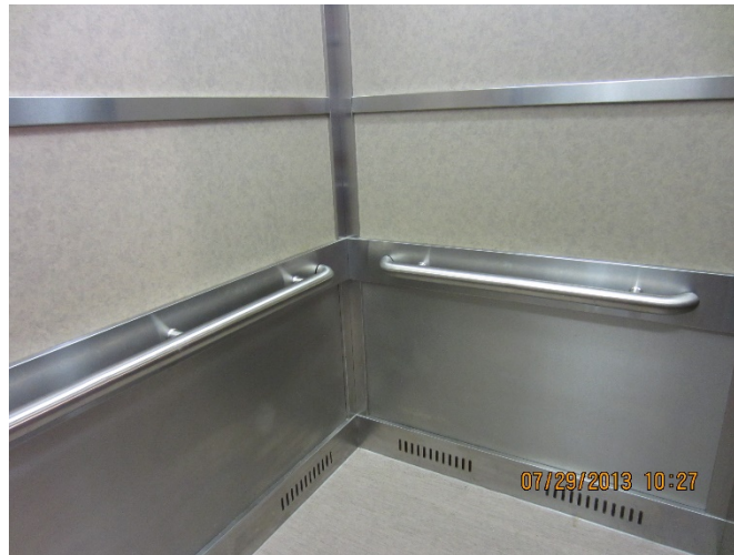
Typical Modernized Wall Panel Layout (with recessed base)
