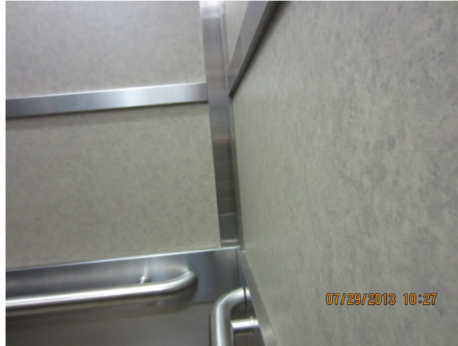
Typical Modernized Raised Stainless Steel Trim Detail
