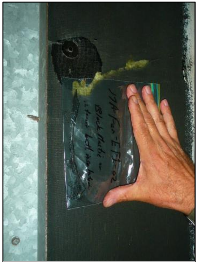
The White and Black Mastics on Interior Batt Insulation as observed and sampled within the Exhaust Fan EFl in the Main Fan Room was found to be None Detected for asbestos.
