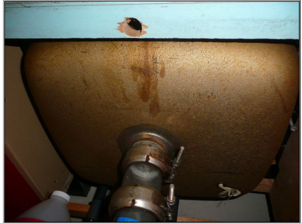
Sinks with Bronzy Silver and/or Greenish Silver Undercoating as sampled in Rooms 107b and 110 and similarly as observed to be present in Rooms 107a, 110b, 125, 127a, 127b, 127c, were determined to be Asbestos-Containing .
