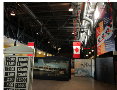
windows shown here in existing space
