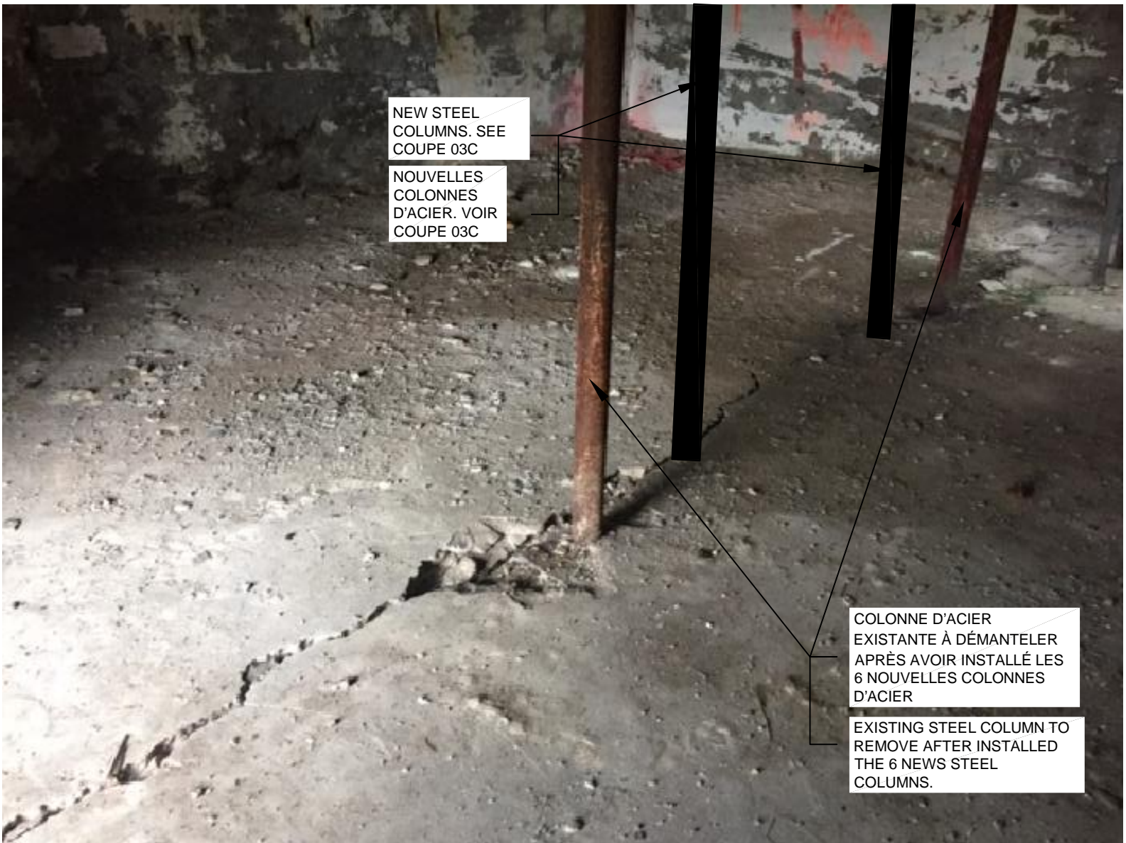
PHOTO 7 - COLONNES EXISTANTES / EXISTING COLUMNS
