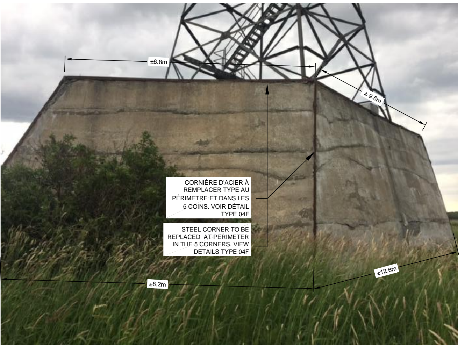
PHOTO 9 - DIMENSION GÉNÉRALES DU PILIER COIN "SUD-OUEST" / GENERAL PILLAR DIMENSION "SOUTH-WEST" CORNER
