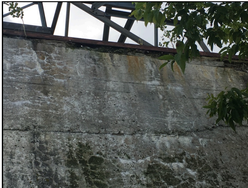
Typical cracking caused by the alkali-aggregate reactivity (AAR)
