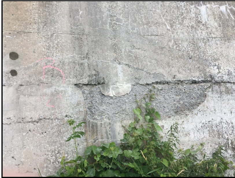
Delaminated concrete and location of additional cores
