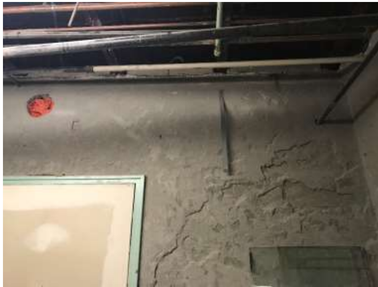
Asbestos Masonry Block Wall Coating (Sample S0004), 4-002 (Location:41)
