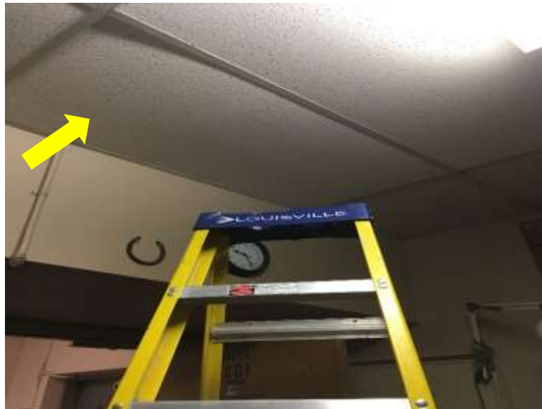
Non-asbestos Lay-In Ceiling Tiles, Pinholes and Random Flakes (Sample S0020), 4-215 (Location:62)
