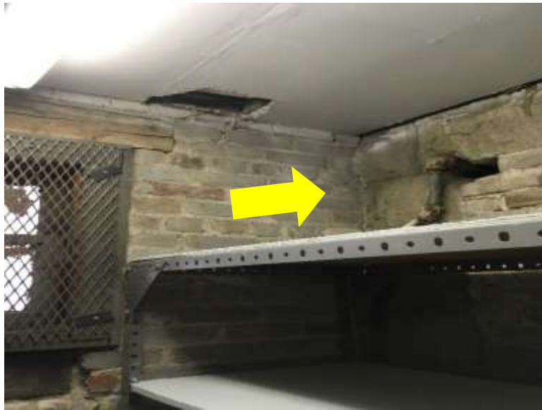
Non-asbestos visually similar Grey Brick and Mortar (Samples S0010 and S0011), 3-211 (Location:12)
