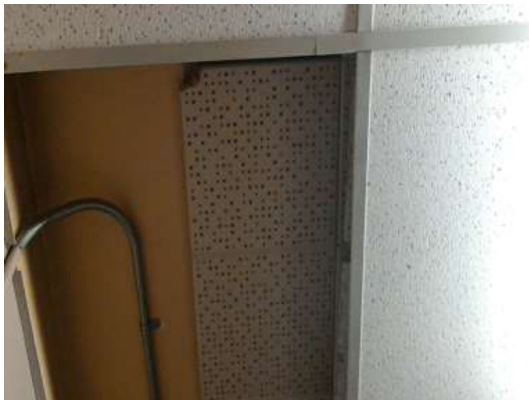
Non-asbestos Glued-on Ceiling Tiles, 1x1 large holes, Ref G-4-203-118, (Sample S0012A), 4-202 (Location:52)
