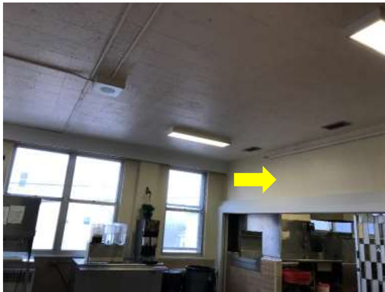
Asbestos Drywall and Joint Compound (Sample S0002), 4-135 (Location:13)
