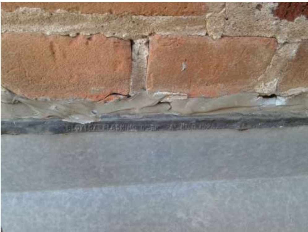
Mastic, Grey mastic at roof flashing , (Sample S0021), Roof (Location:43)
