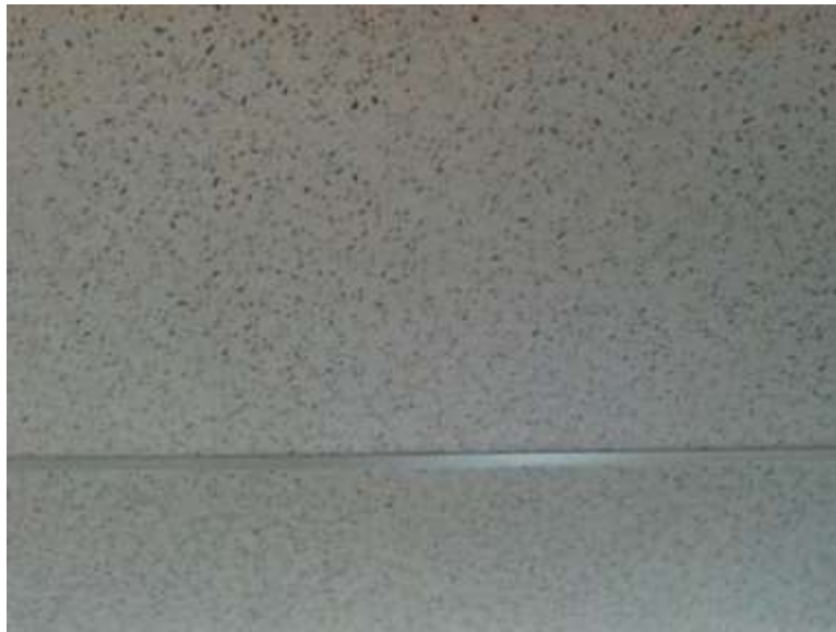
Non-asbestos Lay-in Ceiling Tiles, 2x4 pinholes and small flakes, (Sample S0001B), 1-002-5 (Location:10)
