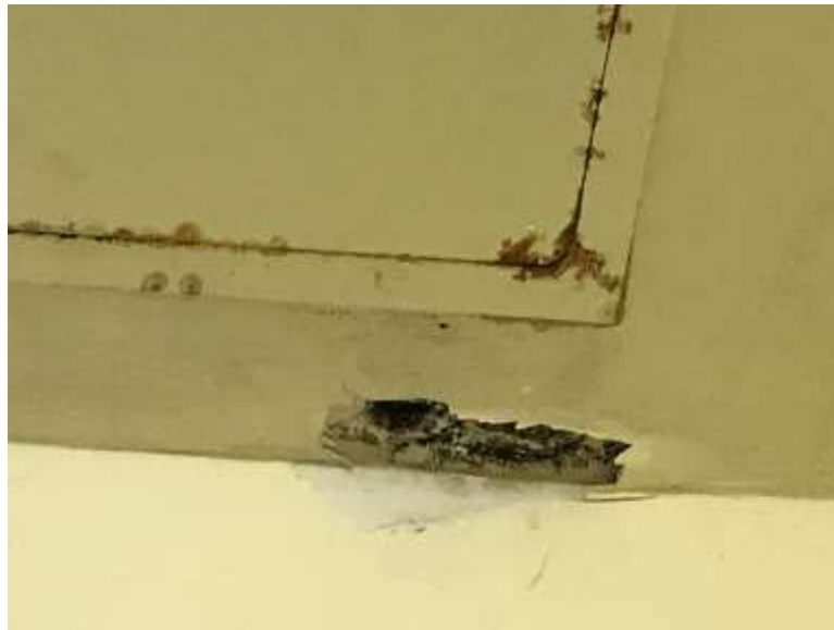
Mould impacted Plaster ceiling, 4-124 (Location:10)
