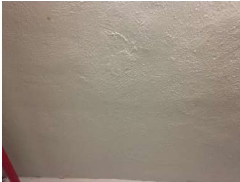
Non-asbestos Plaster texture, Ref 1-007-112 (Sample S0007), 1-007 (Location:5)
