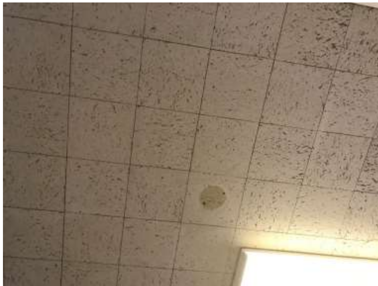
Non-asbestos Glued-on Ceiling Tiles 1X1 With Fissures and Brown Mastic, Ref G-4-132-153 (Sample S0005 and S0006), 4- 131 (Location:20)
