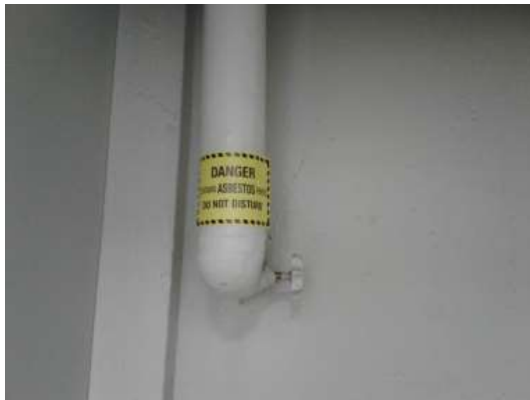
Parging Cement Insulation, Asbestos labelling, (Sample V9000), 4-029 (Location:45)
