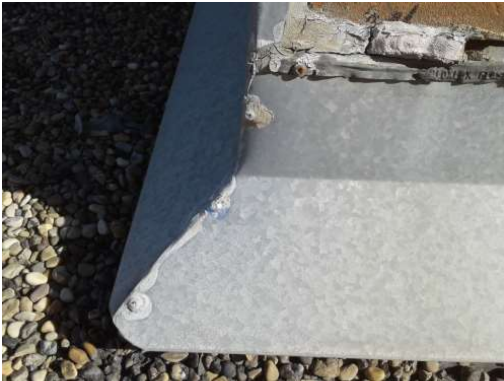
Mastic, White mastic on flashing , (Sample S0024), Roof (Location:43)
