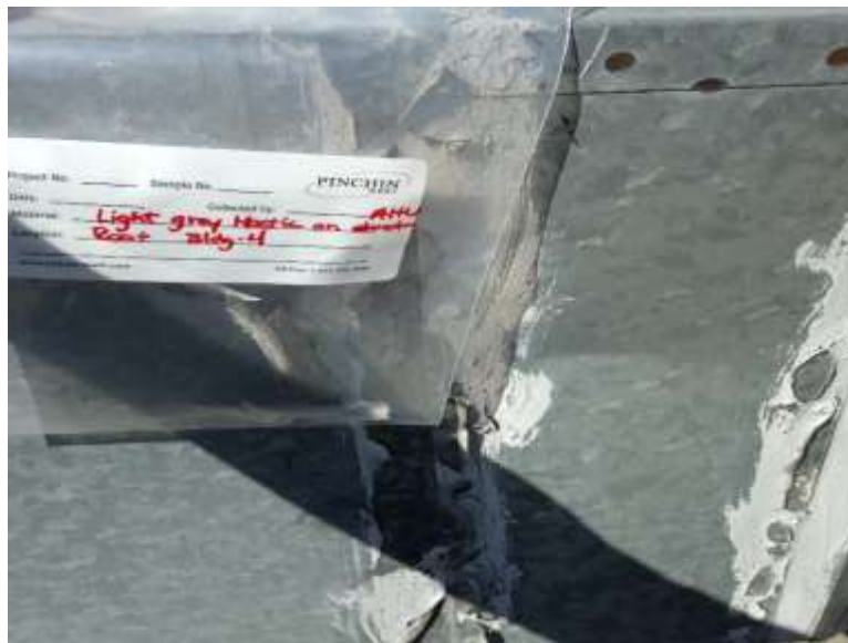
Asbestos-containing light grey mastic on Air Handling Unit, Roof (Location:79)
