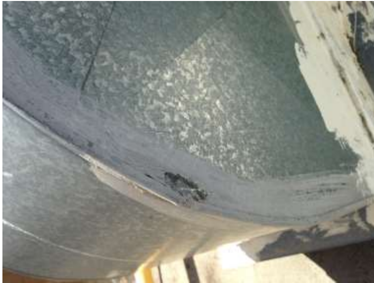
Non-asbestos light grey mastic on Air Handling Unit. Roof (Location:79)
