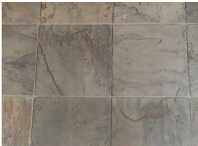
Non-asbestos Vinyl Sheet Flooring, Squares, (Sample S0015), 1-242 (Location:26)
