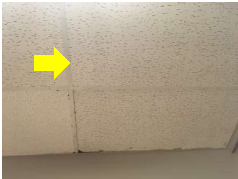
Non-asbestos Lay-In Ceiling Tiles, Pinholes and Long Directional (Sample S0019), 4-206 (Location:53)
