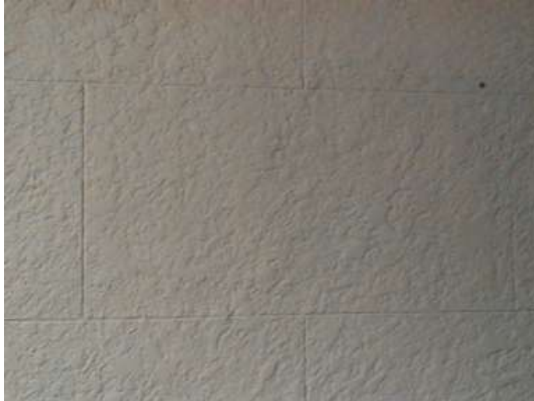
Non-asbestos Texture Finish ( Texture Coat),Ref G-1-119-138, (Sample S0012C), 1-119 (Location:19)
