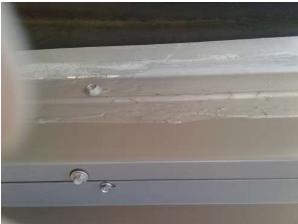
Mastic, Silver mastic on duct, (Sample S0020), Roof (Location:43)
