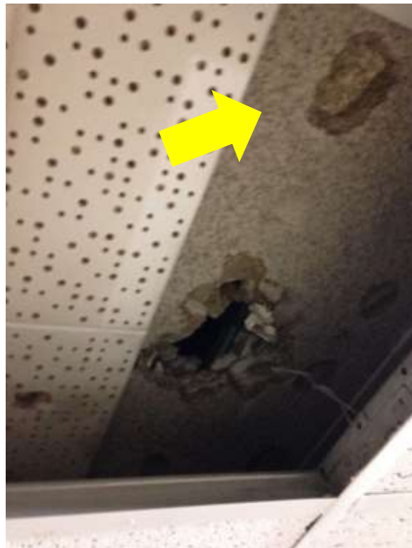
Asbestos Mastic behind Ceiling Tiles (Sample S0014), 4-202 (Location:52)
