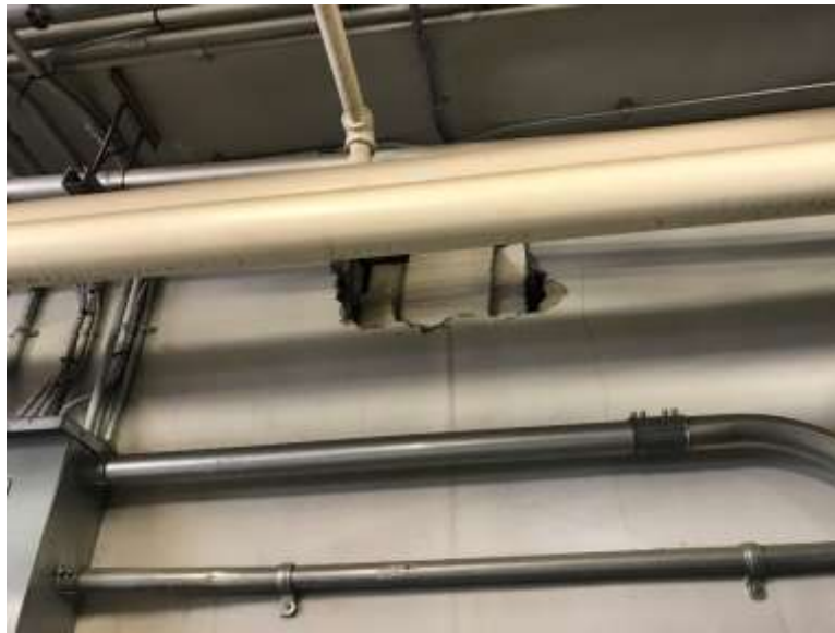
Asbestos Plaster (Sample S0011), 4-025 (Location:46)
