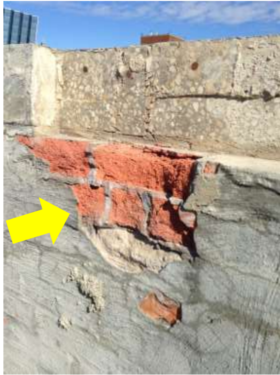
Non-asbestos Stucco and Brick (Samples S0016 and S0017), Roof (Location:36)
