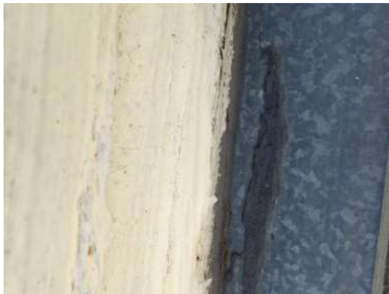
Non-asbestos white mastic on dark grey, Roof (Location:79)
