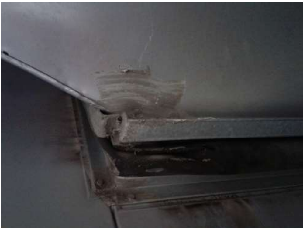
Mastic, Grey mastic on duct, (Sample S0026), 1-016 (Location:15)
