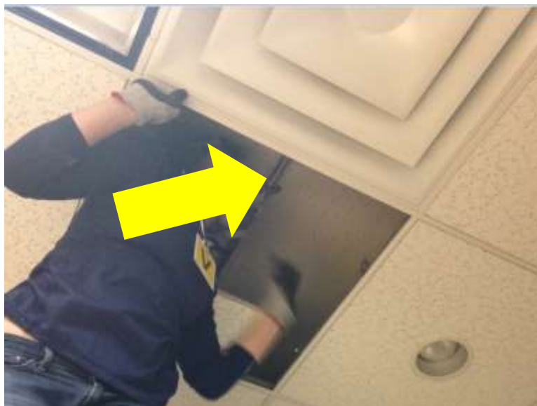
Non-asbestos Glued on Ceiling Tiles 1X1, Ref G-1-102-140, (Sample S002), 1-110 (Location:1)
