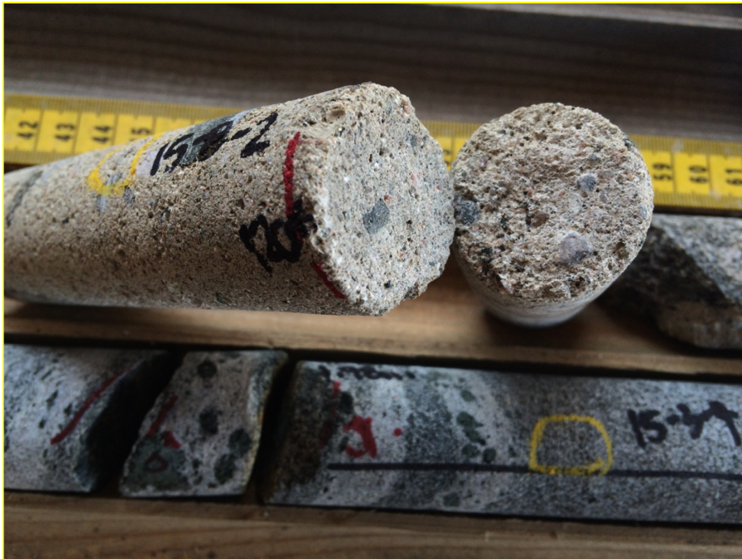
DH15-8 detail showing concrete cold joint within concrete core at 0.51 m from collar.
