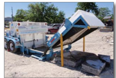
Figure 17. Delivering hardened concrete to a recycler
