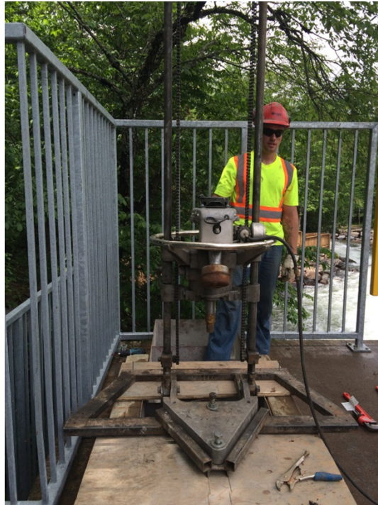
Winkie Drill set up on DH15-1 looking downstream.
