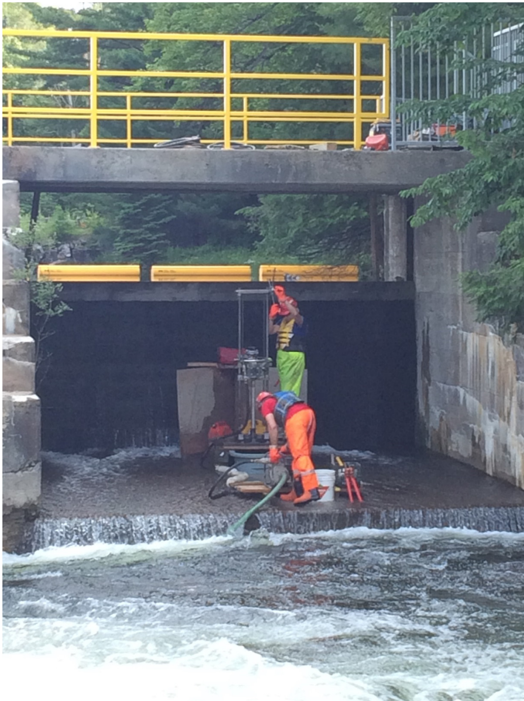
Detail of set up and drilling on DH15-5 on July 3, 2015.
