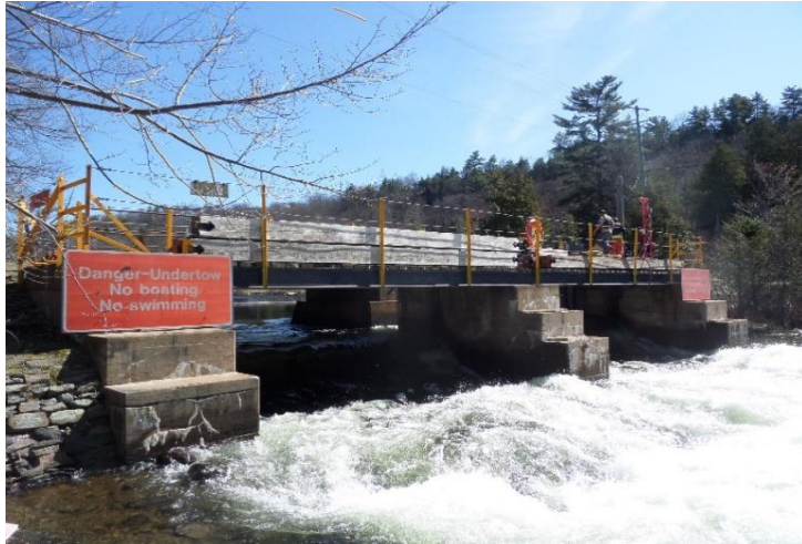
PHOTOGRAPH 1: Downstream Dam View
