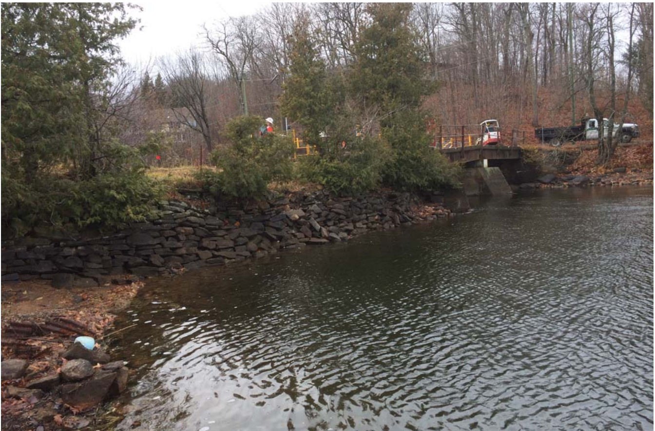
Photograph 4: Facing south on the north side of the dam.
