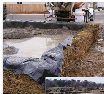
Figure 9. Hay bale and plastic washout pit
