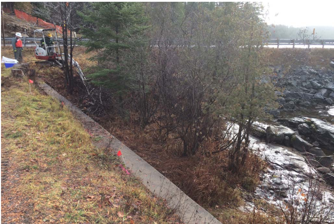
Photograph 2: Minimal tree and soil cover over bedrock, facing east side of the dam bridge.
