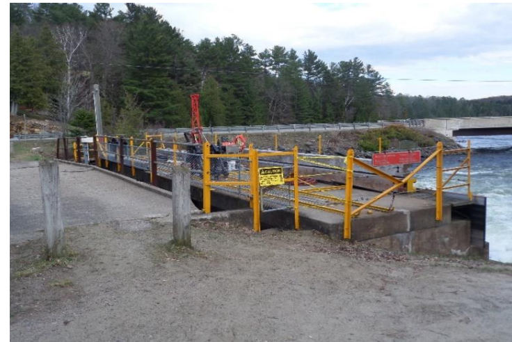
PHOTOGRAPH 2: Drilling Equipment on Dam
