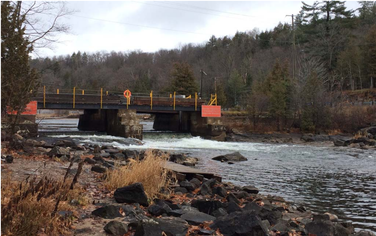
Photograph 1: Twelve Mile Dam, south side of structure, facing north.
