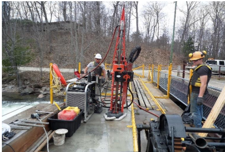
PHOTOGRAPH 3: Borehole TWM-03 Location
