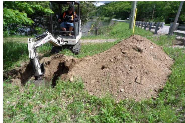
PHOTOGRAPH 4: Test Pit Excavation
