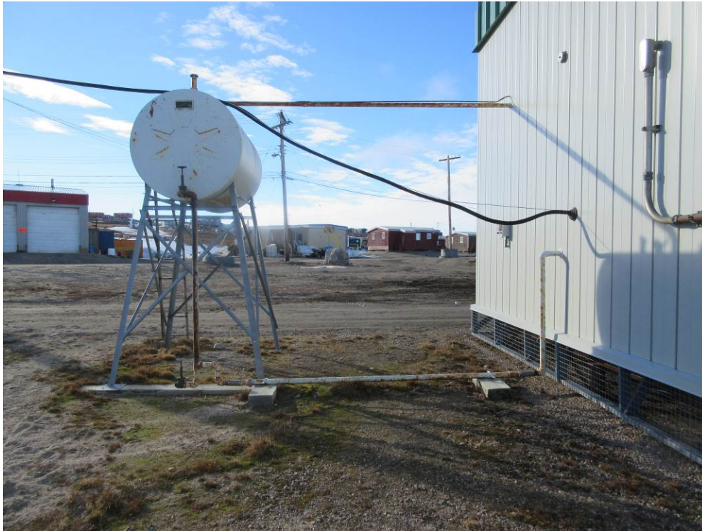
Photo 11 Exterior Tank Elevation
