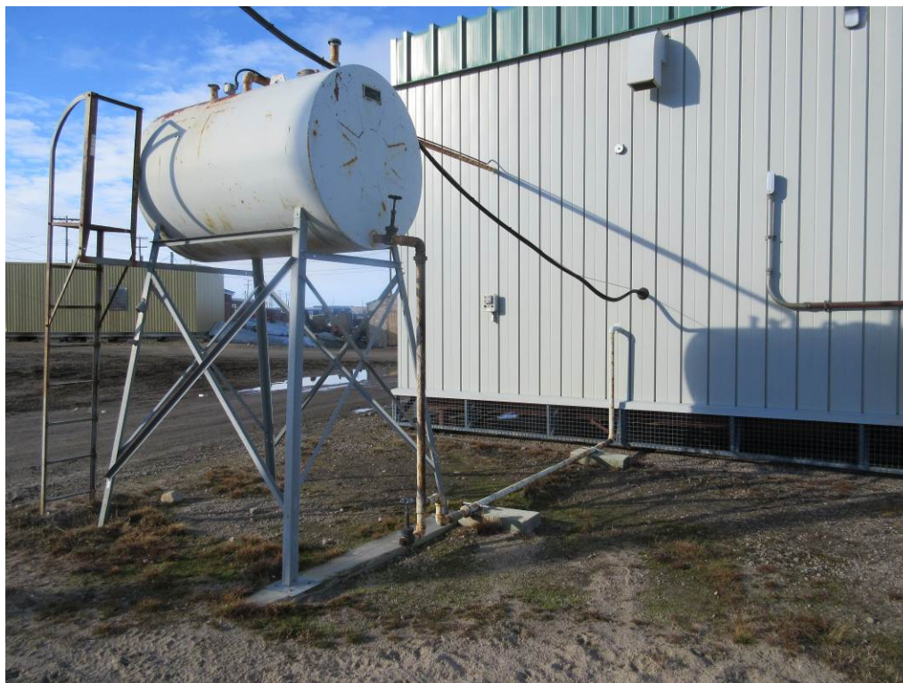
Photo 10 Exterior Tank Elevation
