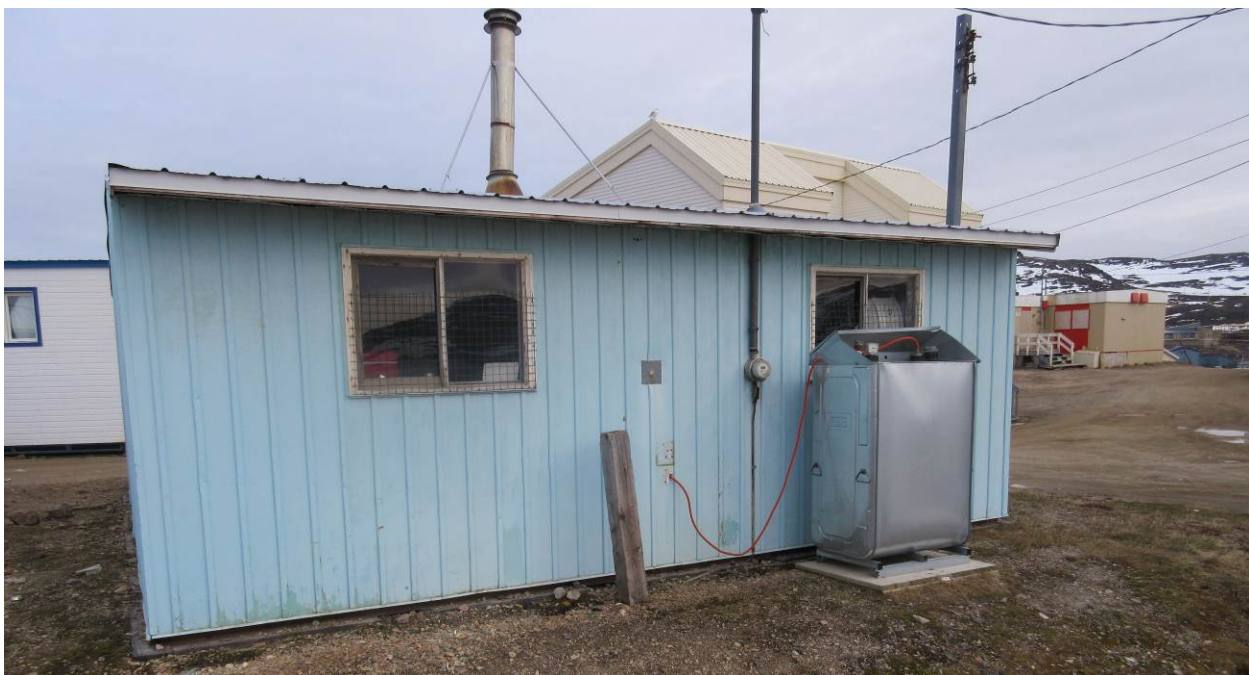
Photo 6 Rear Elevation of Fuel Tank
