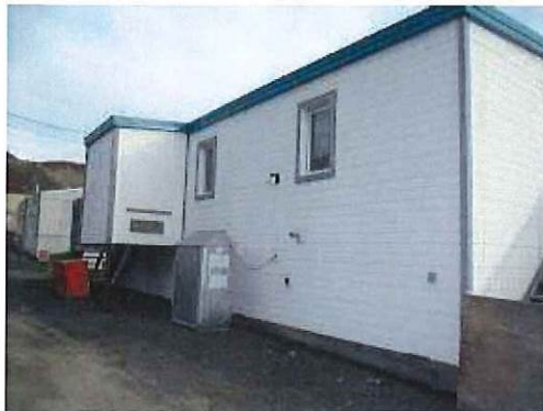
Photo 1: Outdoor above ground fuel tank
