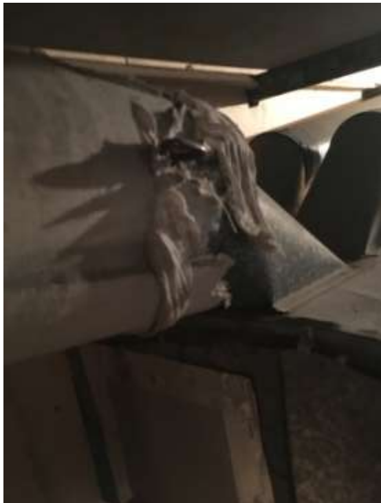
Figure 2: Pipe Wrap in Basement (NL3512-L07)
