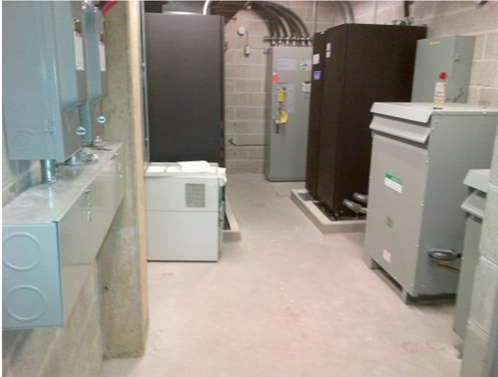
Figure 3: Elec Rm 010 – black cabinets are UPS.
