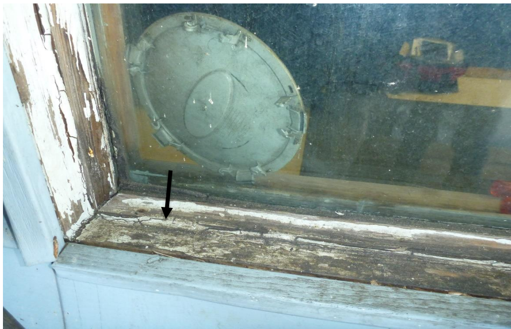
Photo 2: Exterior window caulking, along the northwest side of the control house, presumed to be asbestos-containing. Approximately 20 linear feet of this material was observed to be in fair condition.
