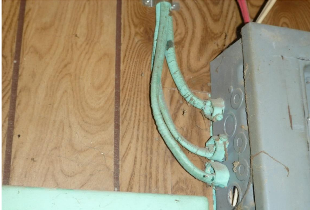
Photo 11: Wire sheathing protruding from the storage room electrical box, presumed to be asbestos-containing.
