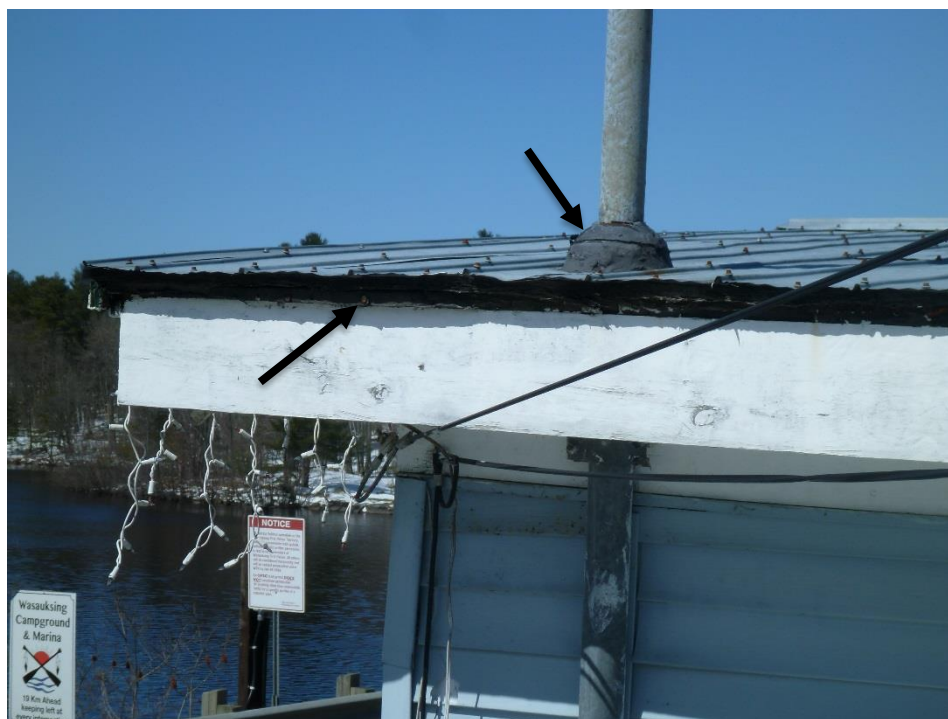
Photo 3: Roofing materials present under metal sheeting and as caulking presumed to be asbestos-containing.
