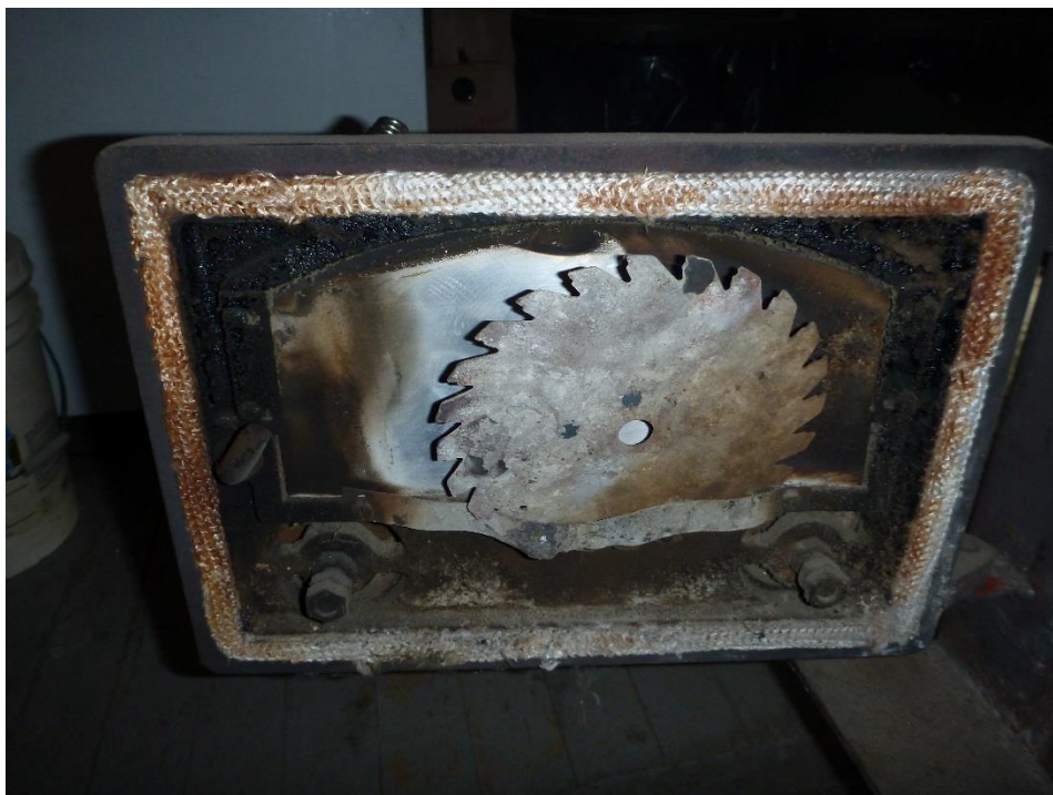
Photo 14: Gasket associated with the wood fireplace, presumed to be asbestos-containing (not sampled to avoid compromising heat source seal).
