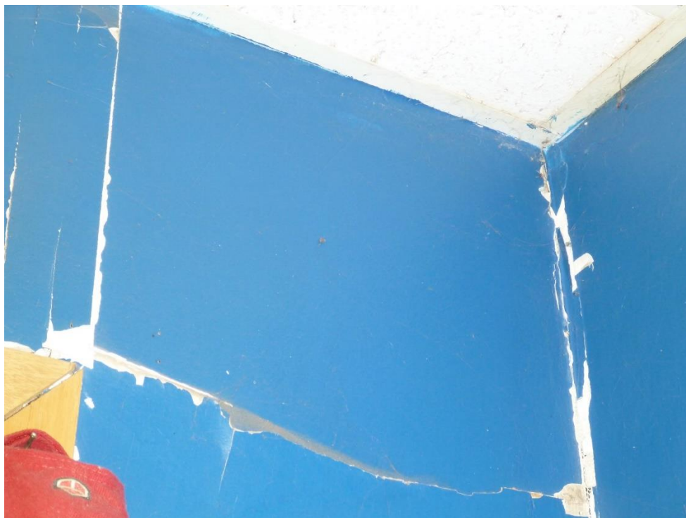
Photo 7: Drywall joint compound located in the control room and kitchen, determined to be non-asbestos.
