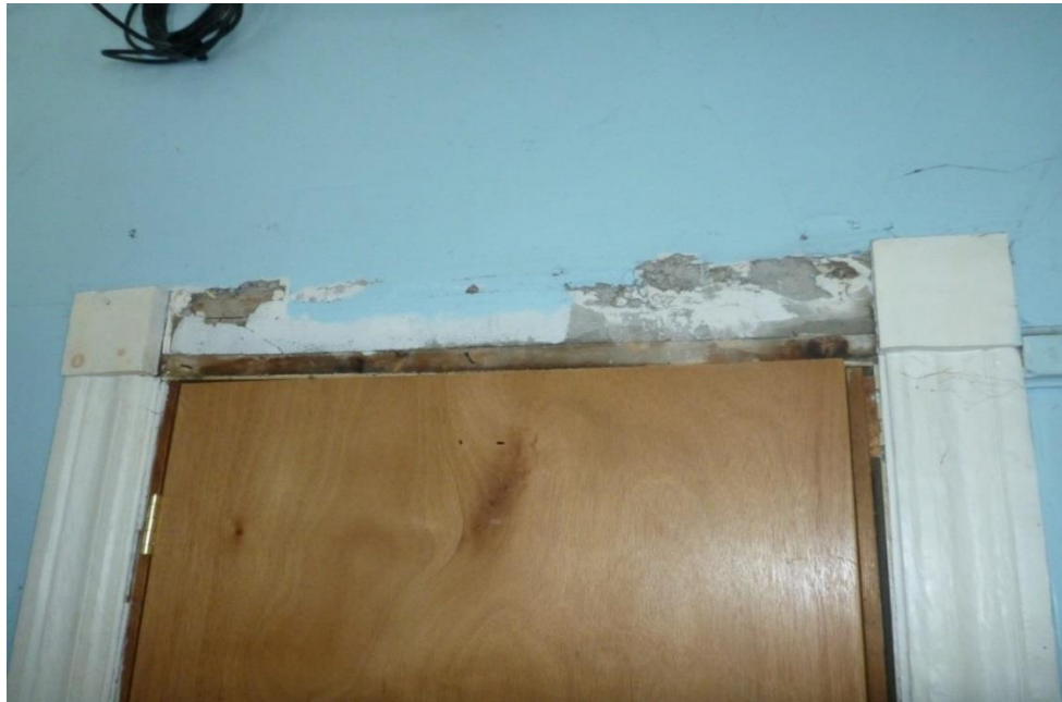
Photo 9: Plaster wall material determined to be non-asbestos, as well as light blue paint determined to contain trace amount of lead (320 ppm).
