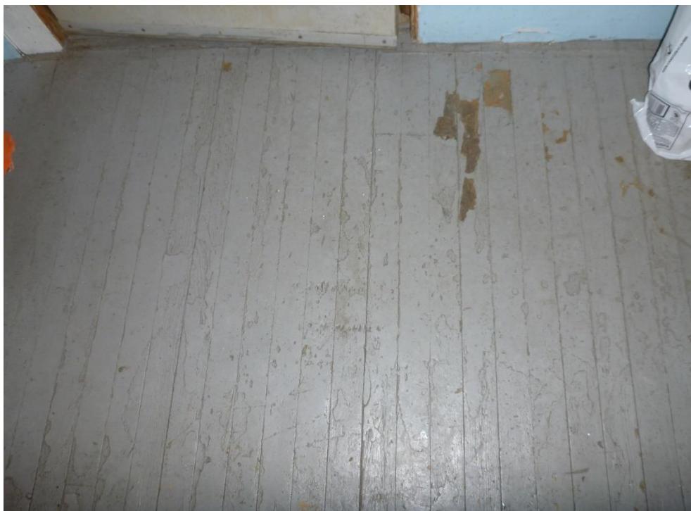
Photo 10: Grey paint on hardwood flooring in the kitchen and storage room, determined to be lead-based (25,000 ppm).
