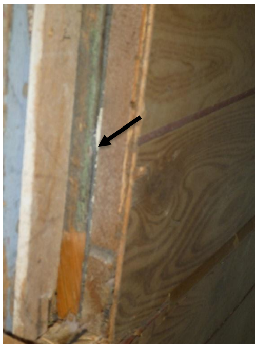
Photo 15: Tar paper present behind vinyl siding on the exterior and behind wood paneling in the storage room, sampled and determined to be non-asbestos.
