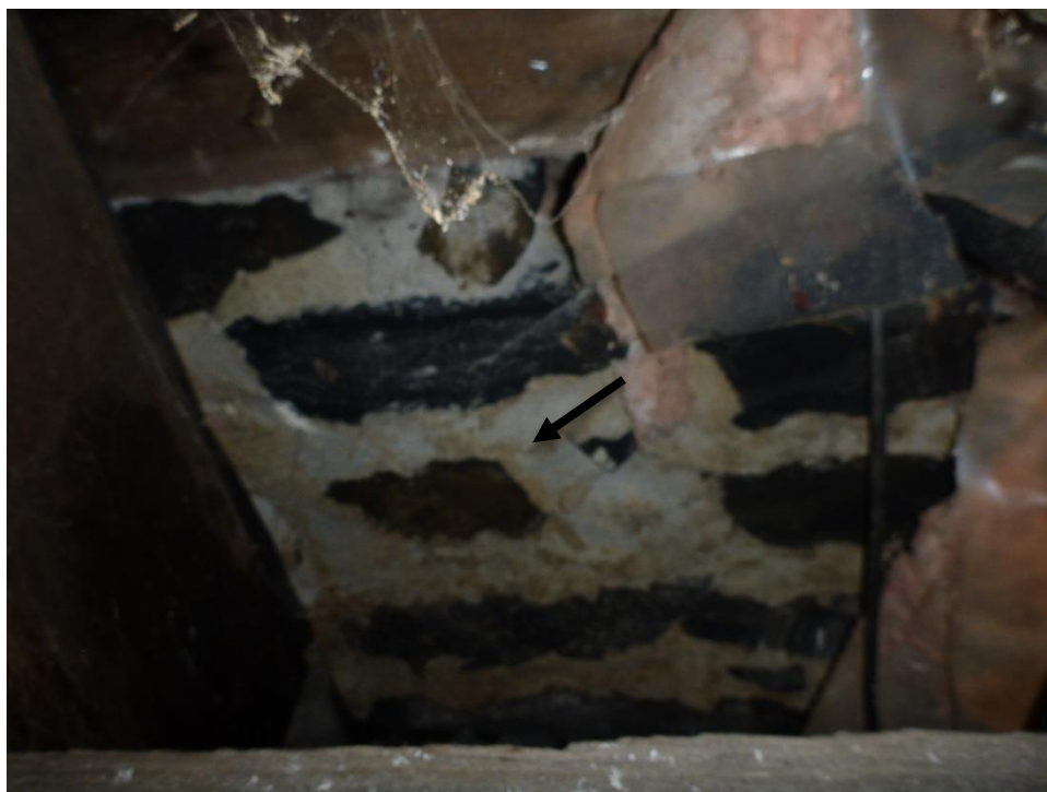
Photo 16: Stone and mortar foundation, with the mortar presumed to contain silica.
