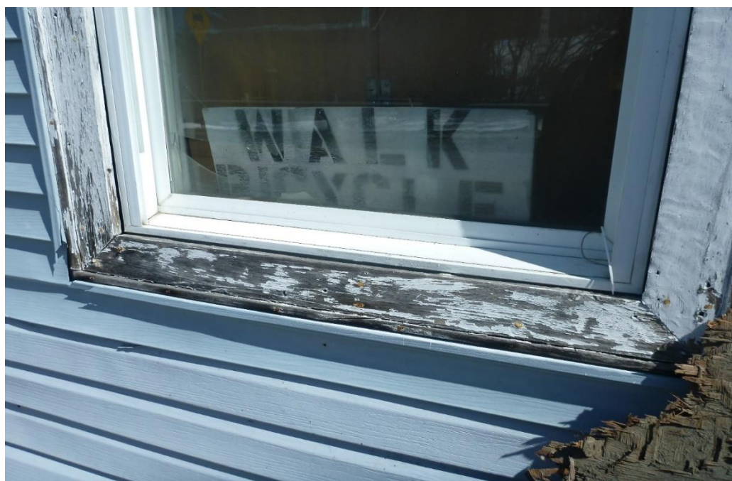
Photo 4: Exterior wooden window frame with white paint determined to contain trace amounts of lead (140 ppm).
