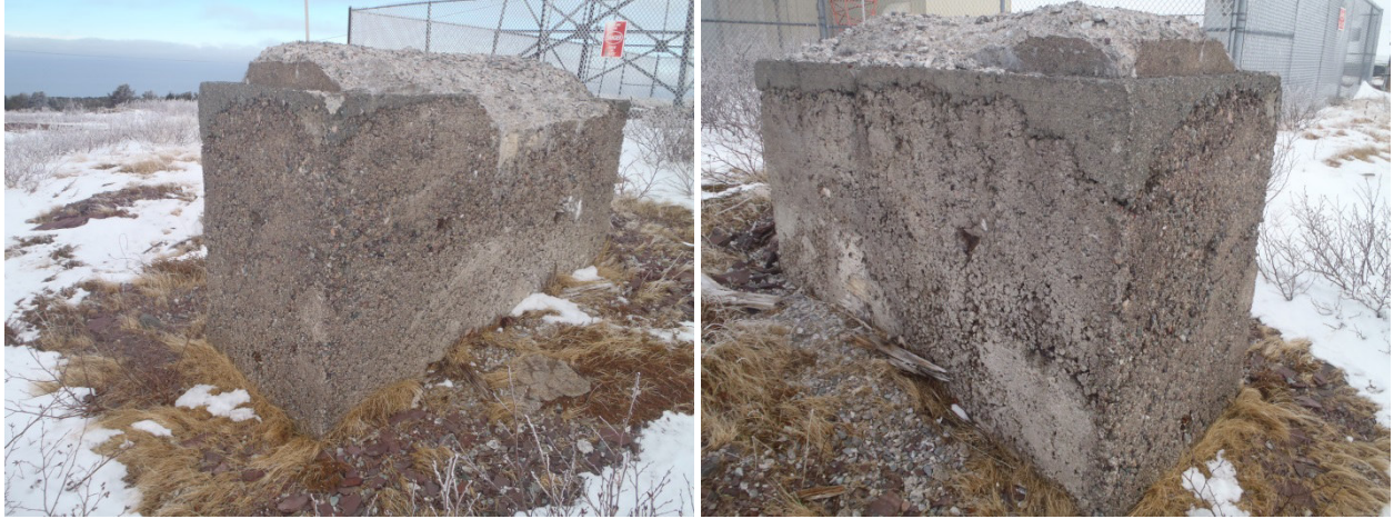
Cuslett – Existing Foundation for Removal
