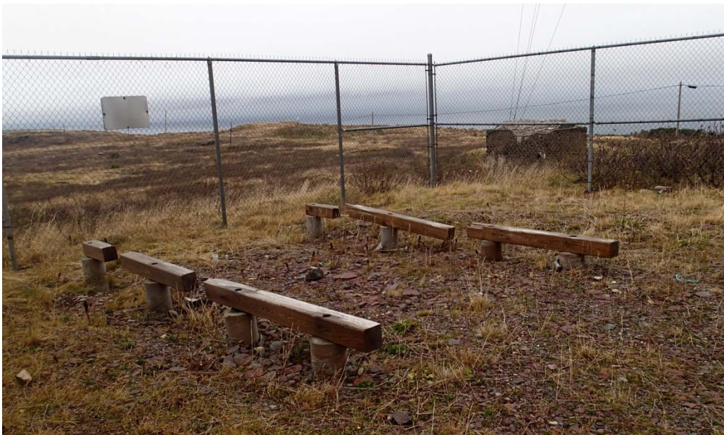
Cuslett – Existing Footings for Removal
