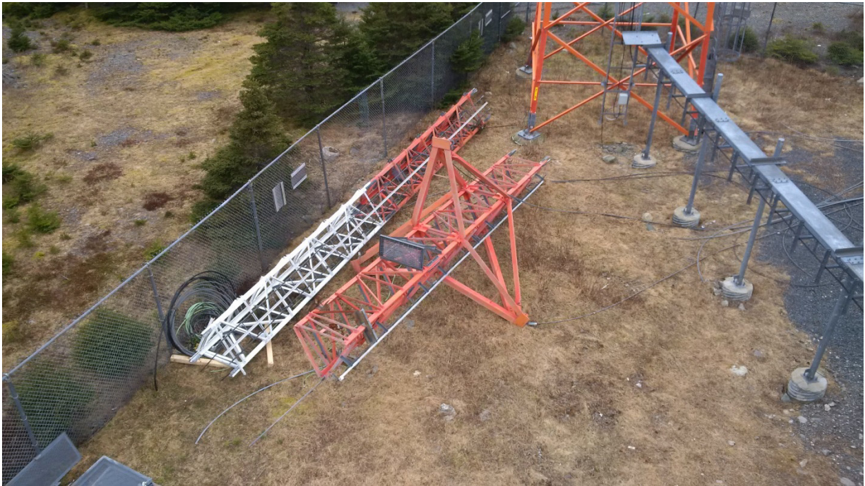
Pearce Peak – VHF Tower Existing Condition
