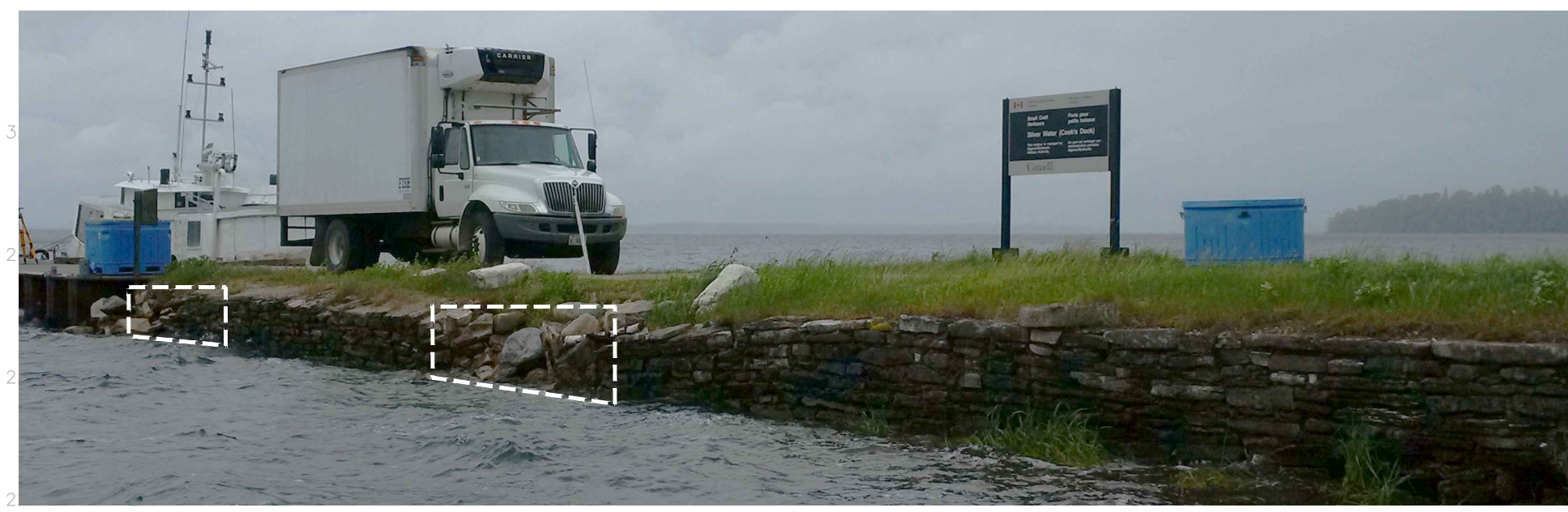
FAILED SECTIONS OF WEST STONE WALL SCALE: NTS
