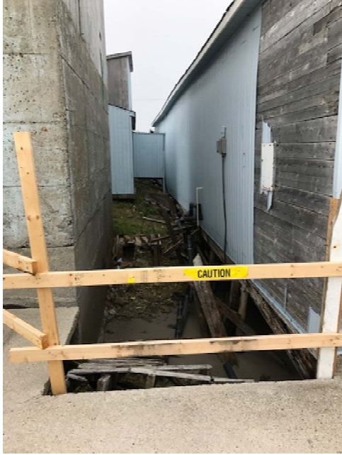
Back of fish plant (west side)
