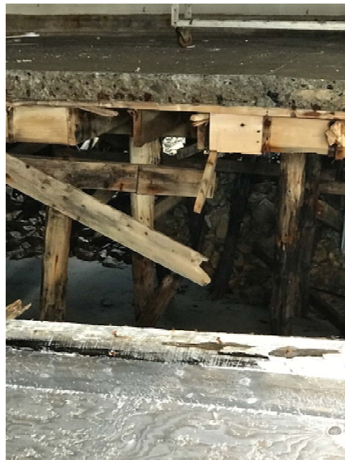
General view – piling foundation of fish plant
