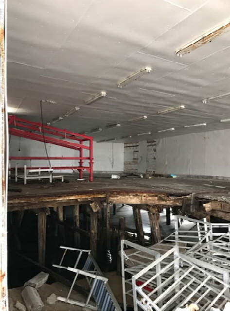
General view – interior of fish plant
