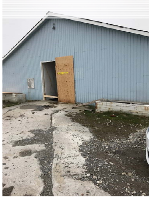
North side – fish plant
