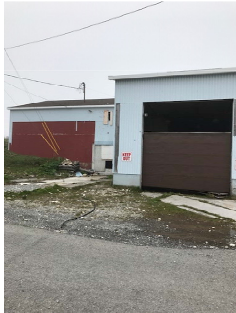
General view – storage building (south side)
