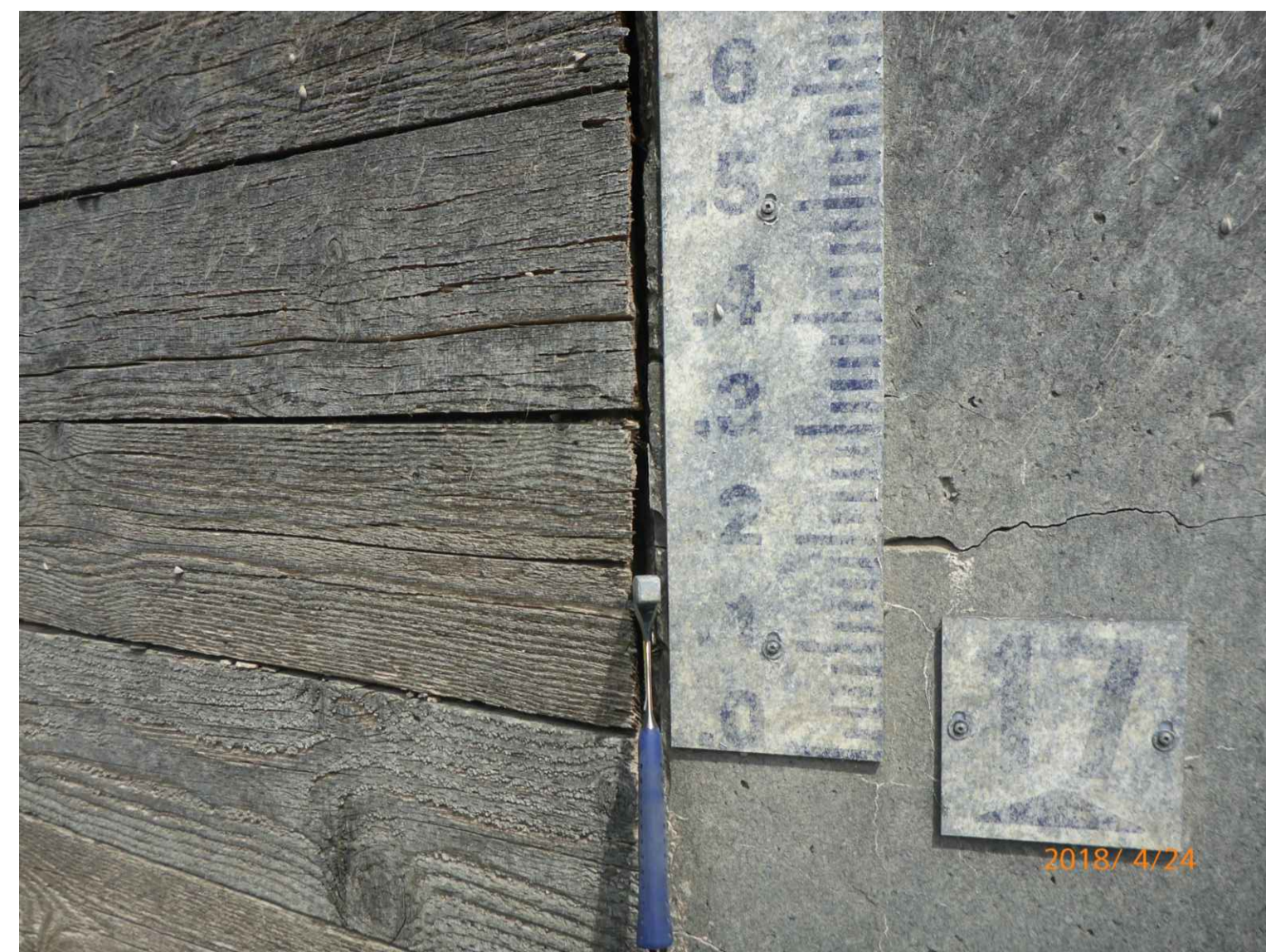
PHOTO 13-1020948 MUR DROIT - AMONT PICTURE RIGHT WALL - UPSTREAM
