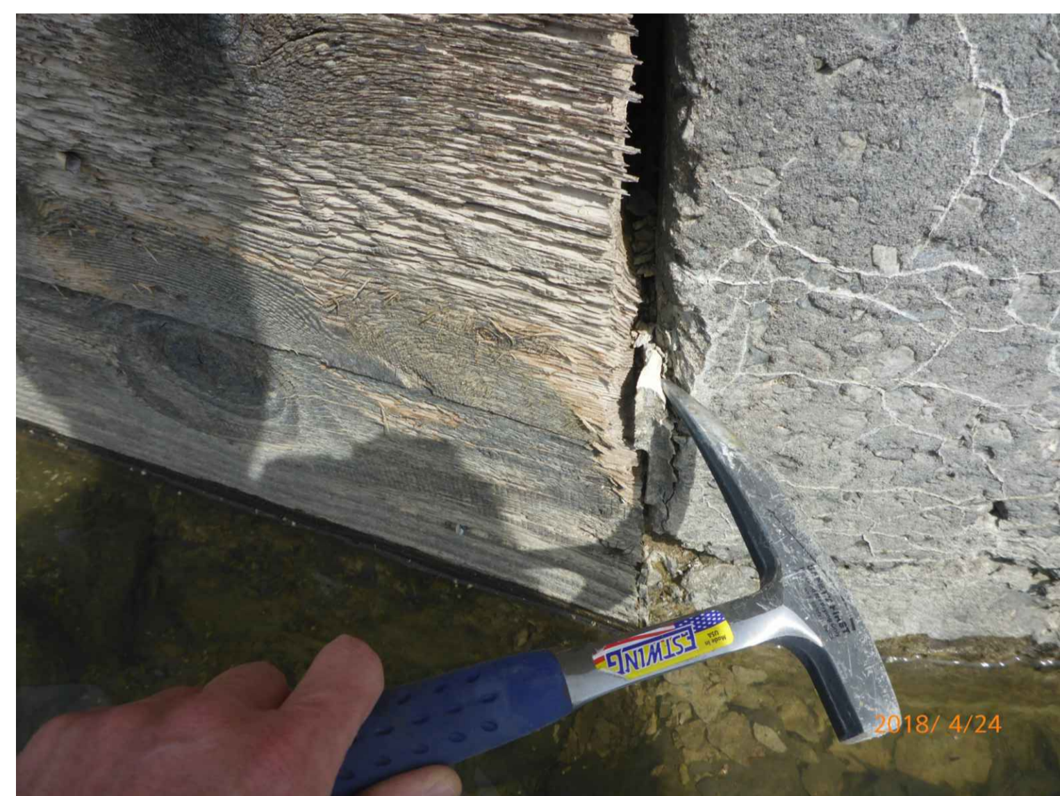
PHOTO 13-1020950 MUR DROIT - AMONT PICTURE RIGHT WALL - UPSTREAM
