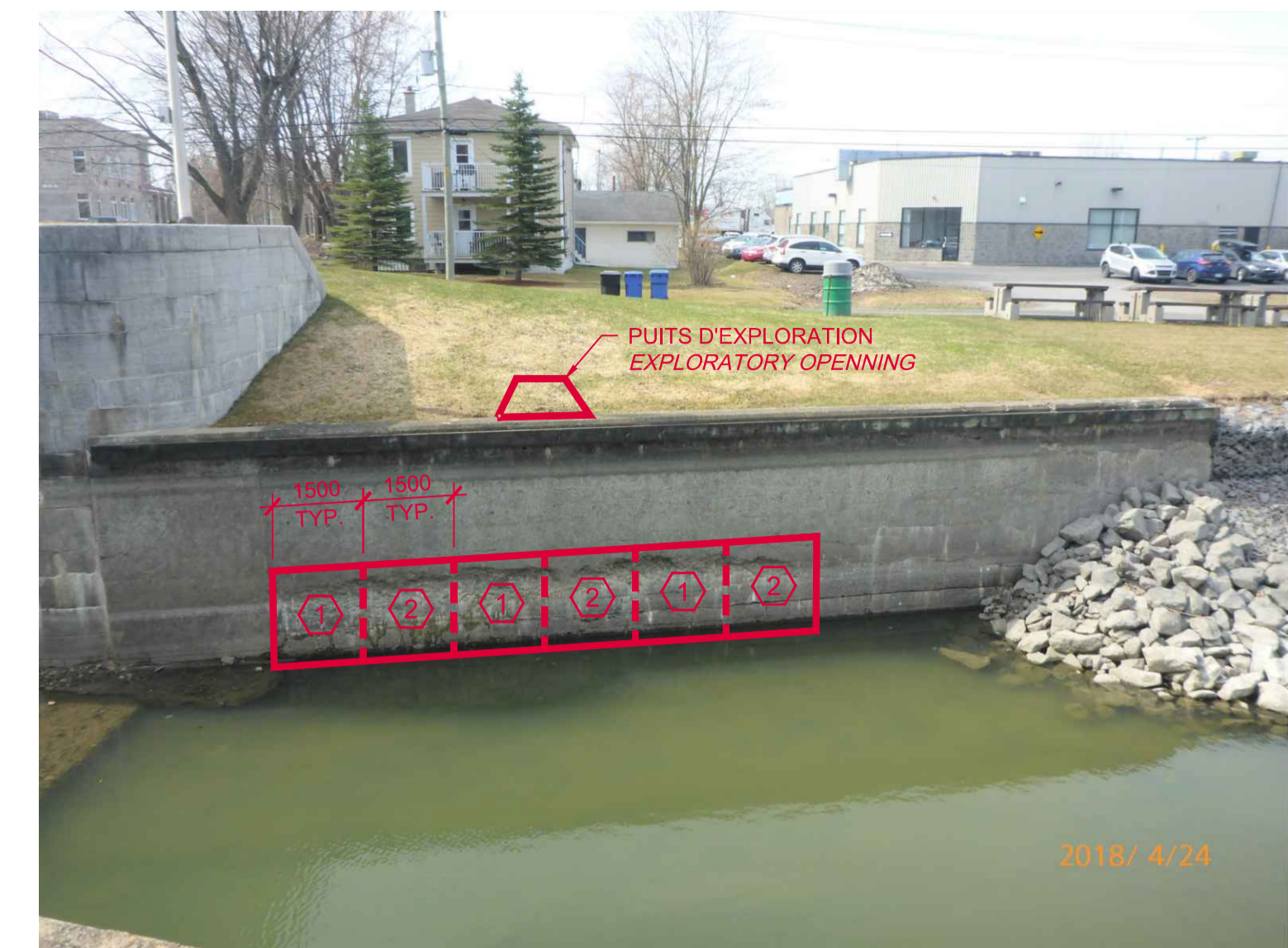
PHOTO 12-1020918 MUR GAUCHE - AVAL PICTURE LEFT WALL - DOWNSTREAM
