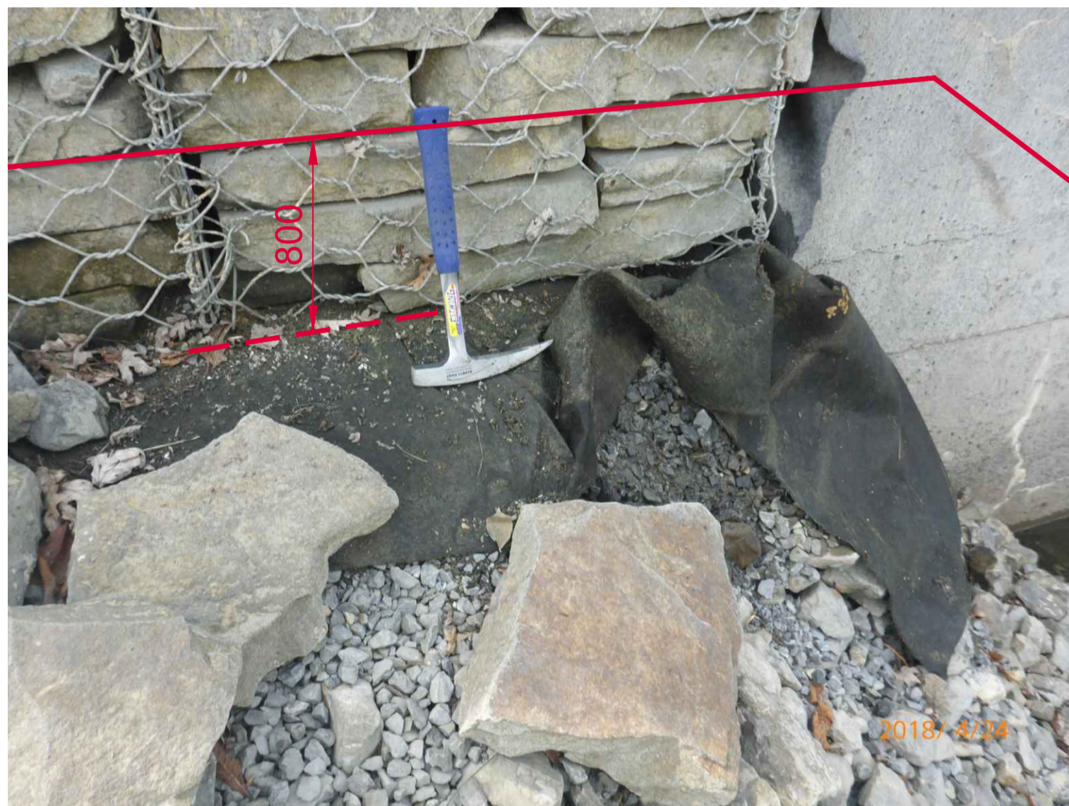
PHOTO 14-1020977 MUR GAUCHE - AMONT PICTURE LEFT WALL - UPSTREAM
