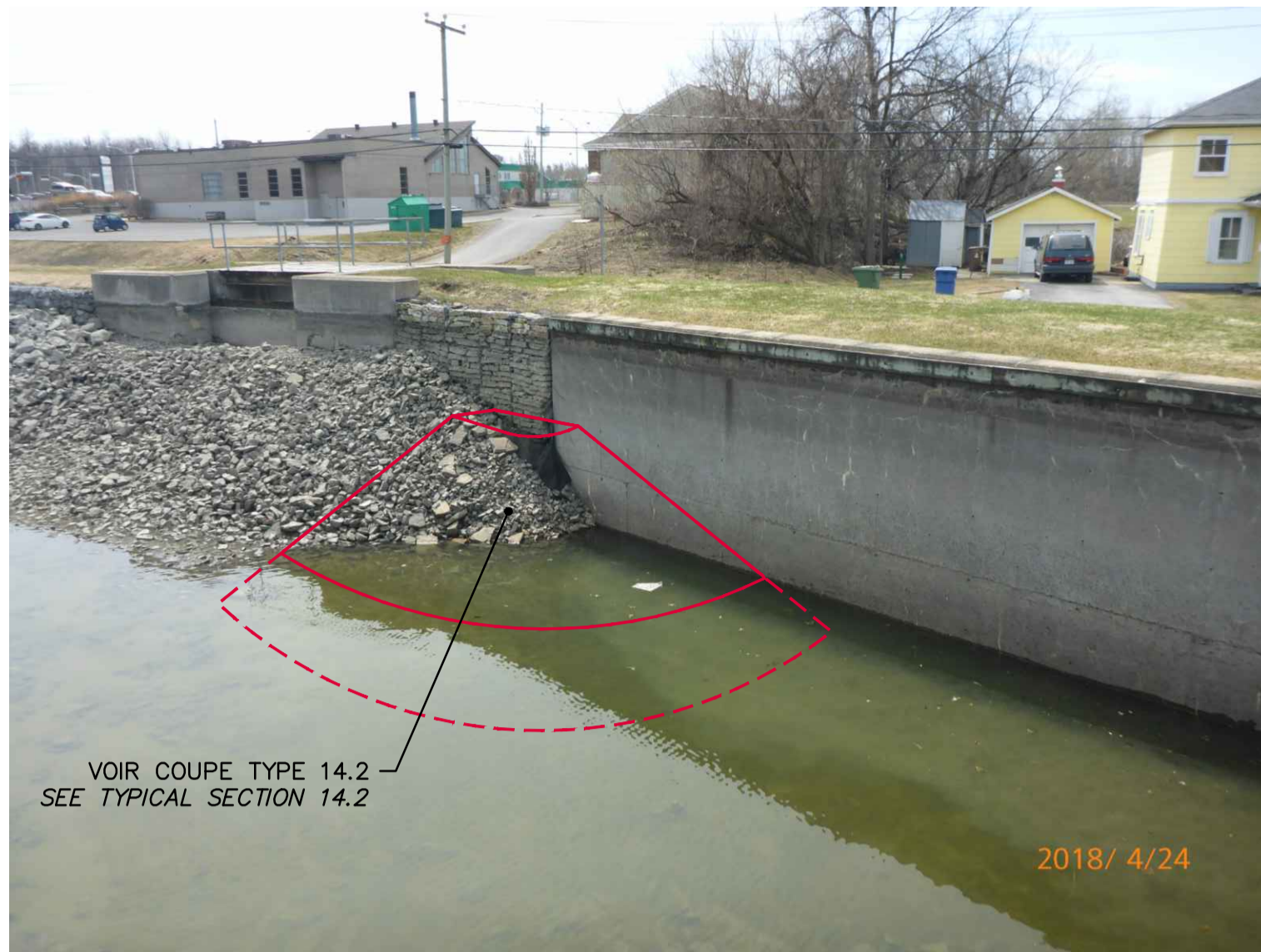
PHOTO 14-1020962 MUR GAUCHE - AMONT PICTURE LEFT WALL - UPSTREAM
