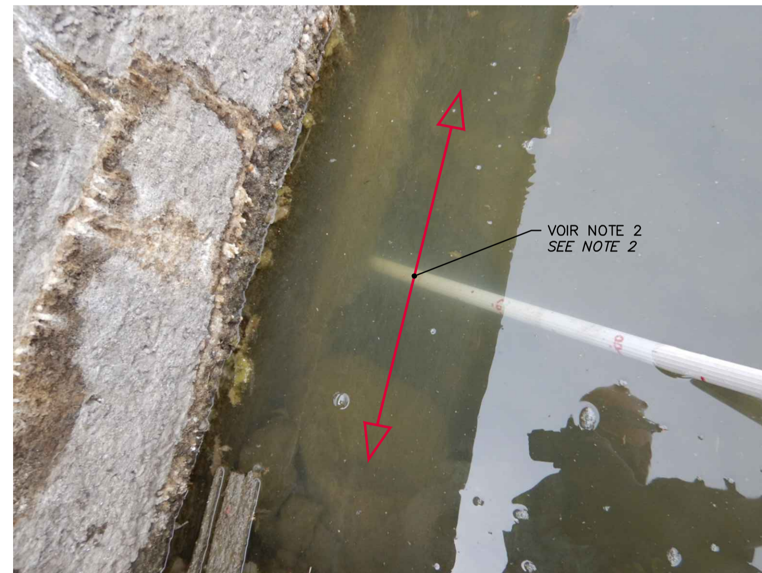
PHOTO 14-9024 MUR GAUCHE - AVAL PICTURE LEFT WALL - DOWNSTREAM
