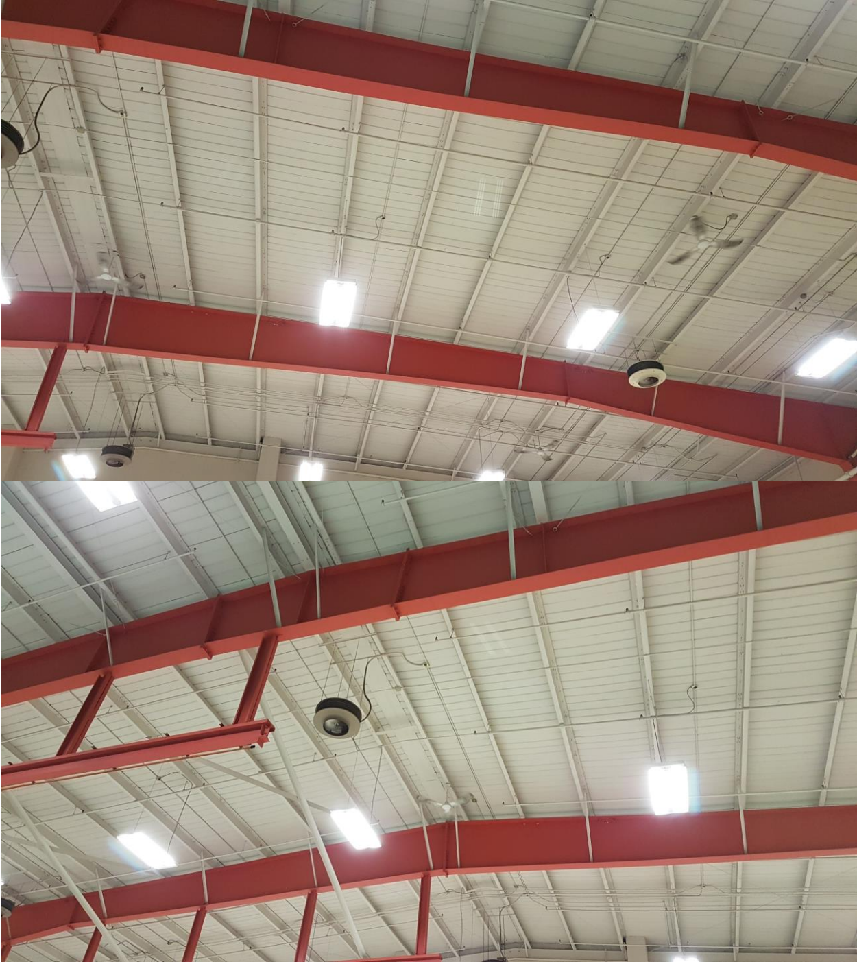
General Aviation Services Building
