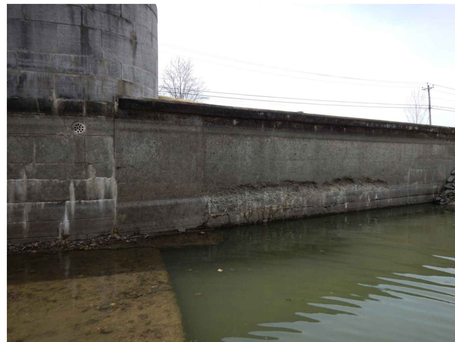
PHOTO 15-9005 MUR GAUCHE - AVAL PICTURE LEFT WALL - DOWNSTREAM
