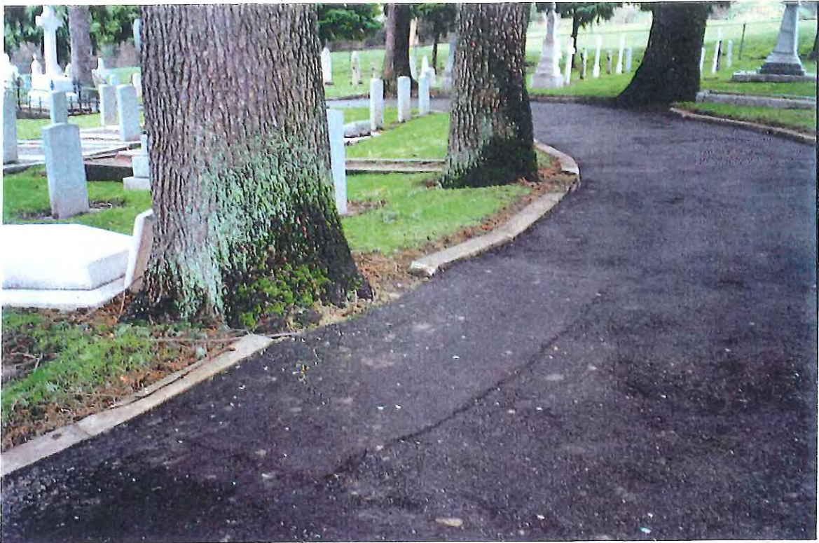
6. Trees Growing into Roadway
