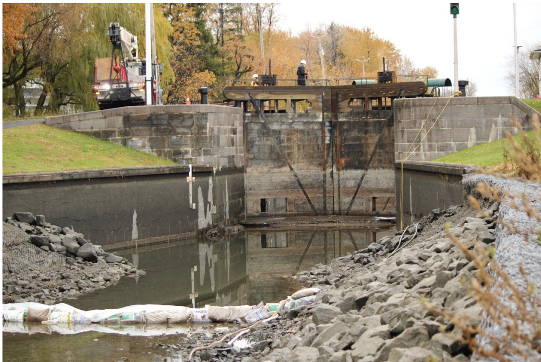
Photo #2 : Lock #4 –PCA downstream cofferdam, upstream view
