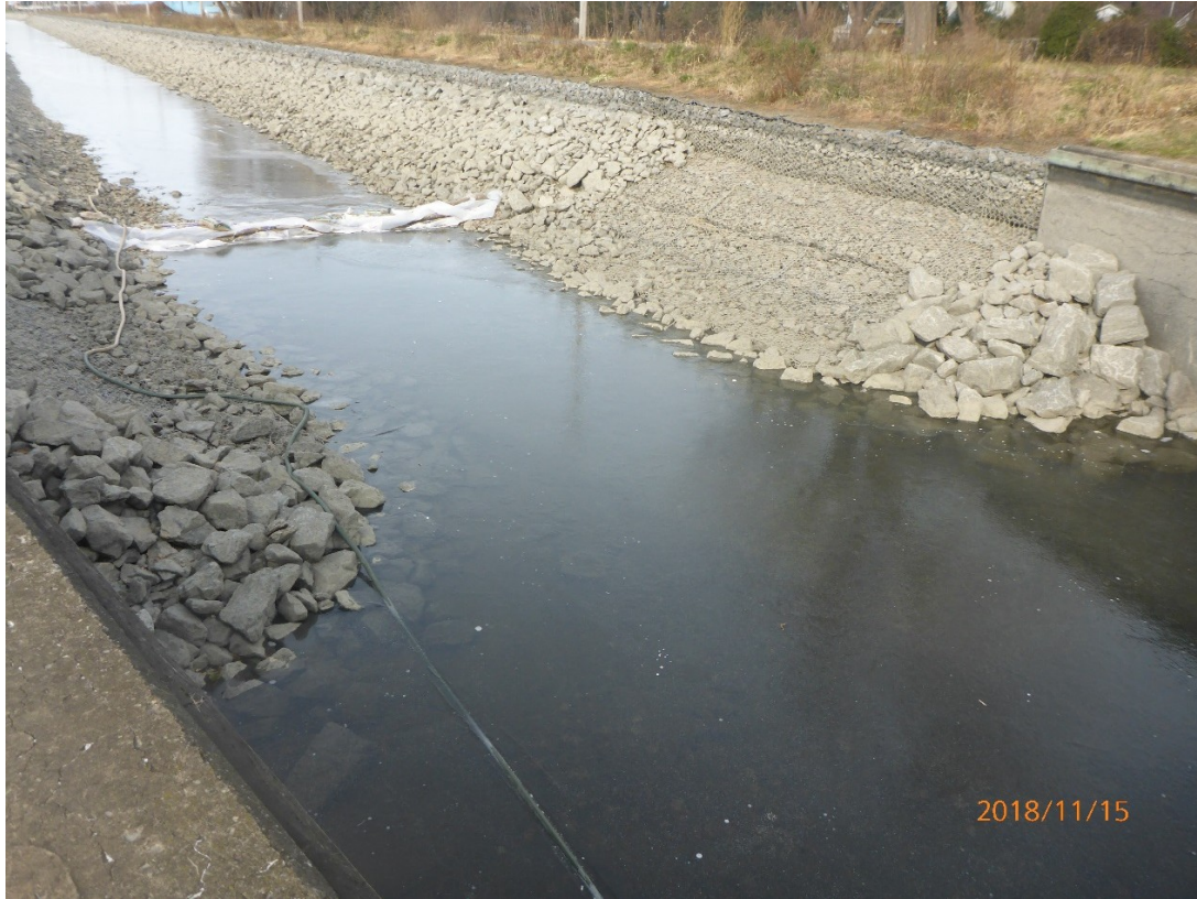
Photo #3 : Lock #4 – PCA downstream cofferdam, downstream view
