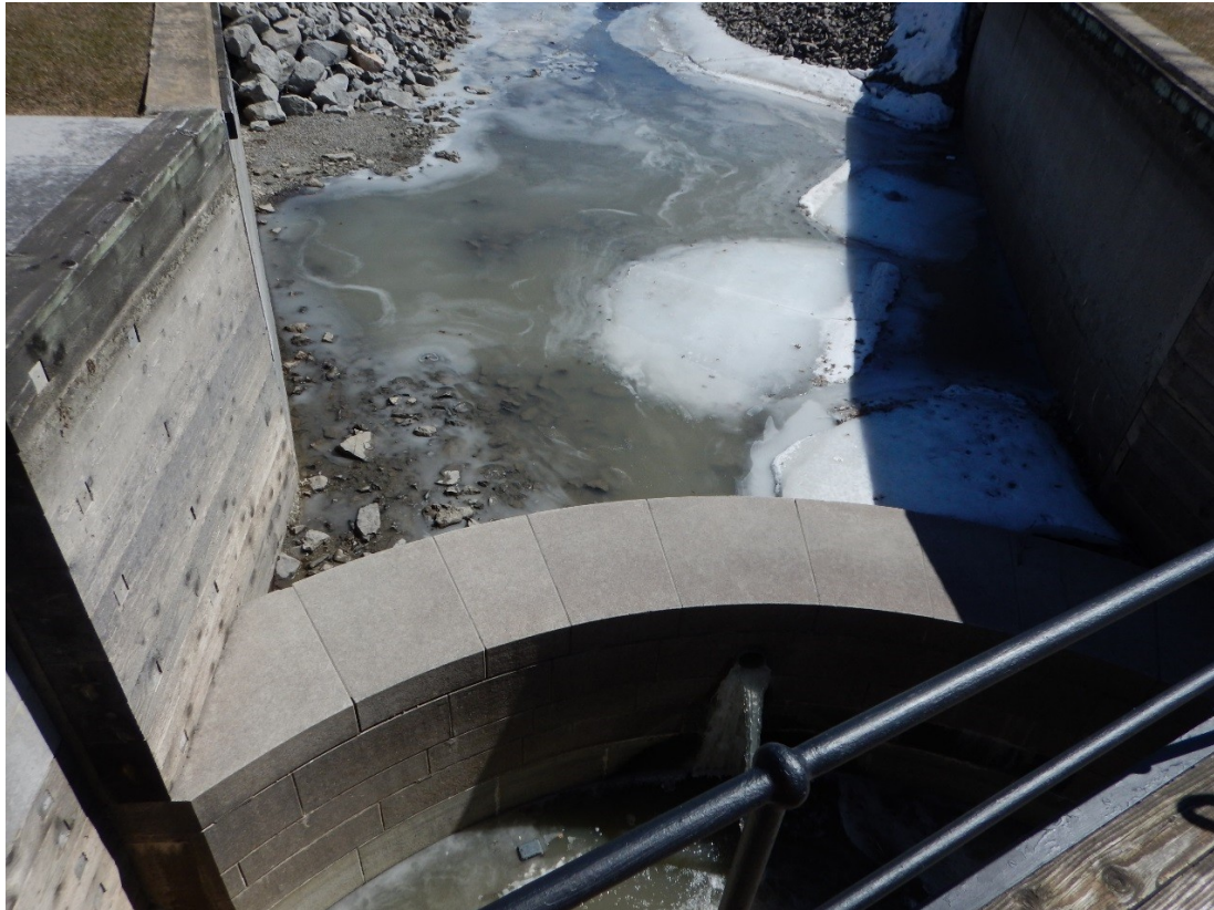
Photo #1 : Lock #4 – upstream fall wall, upstream view
