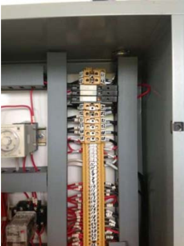
Gate #3 – Control Panel – blown fuse
