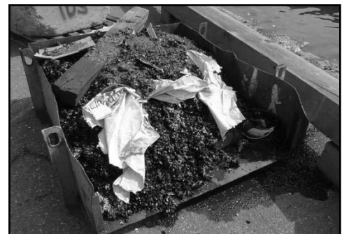
INADEQUATE containment of odorous waste.
