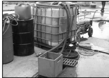
The trench drain is blocked and a sump pump is installed to collect wash water into a tote.
