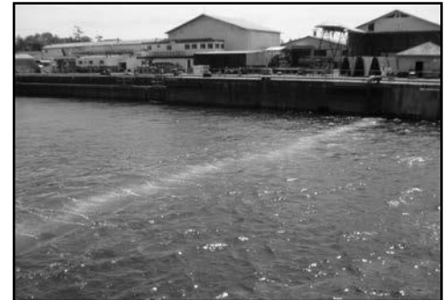
Bubble curtain employed during vessel transfer.
