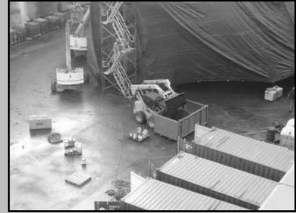
Remove waste grit from work areas as soon as possible to prevent migration of contaminants throughout the drydock floor.
