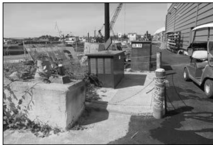
AUTHORIZED Sanitary Sewer Discharge point, Lift Station #11.
