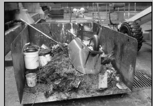
INADEQUATE waste grit storage.
