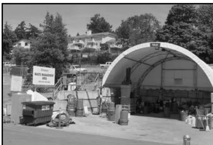
The EGD is located in close proximity to residential areas.
