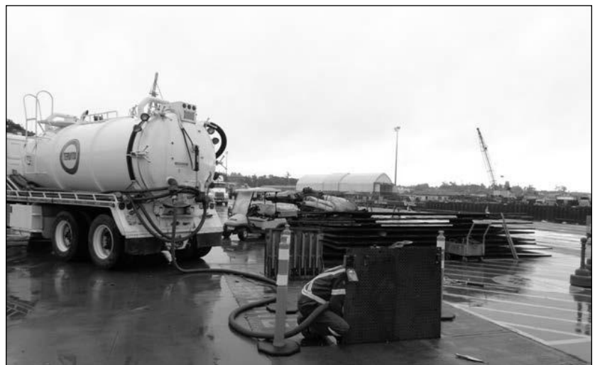
Lift Station Maintenance.
