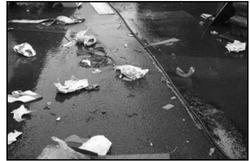
INADEQUATE: Keep work areas neat & orderly.
