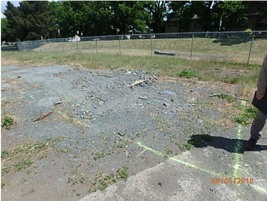
Photo 1: Proposed building site location at 25 Huron Street, Victoria, BC. Photo taken at southwest corner of building lot looking north. Note: The spray-painted lines designate the approximate location of the proposed Project.
