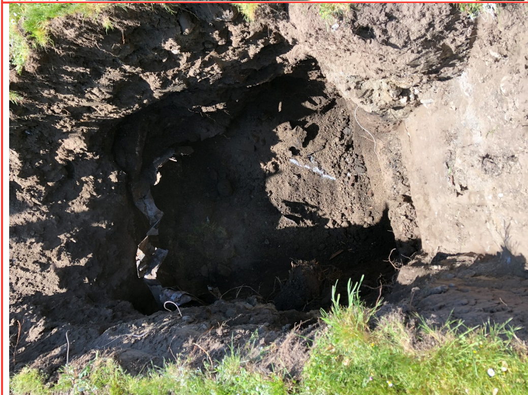
Photo 6: TP18-04 terminated at 2.3m in bedrock
