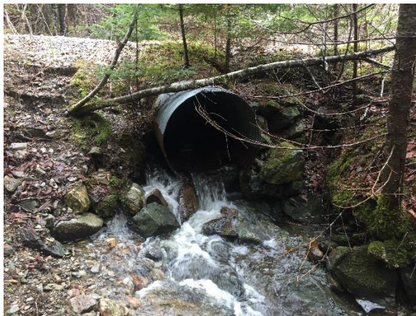
Figure 13: One of the Culverts to be Replaced along the Goose River Trail & Drainage Swale Design
