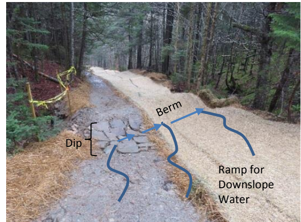
Figure 14: Design and Example of Rolling Grade Dip (Grade Reversal)
