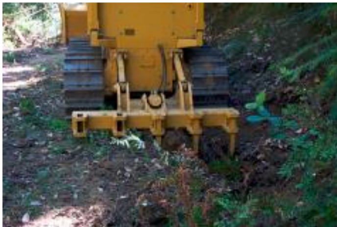
Figure 16: Root Rake Used to Scarify Road Surface
