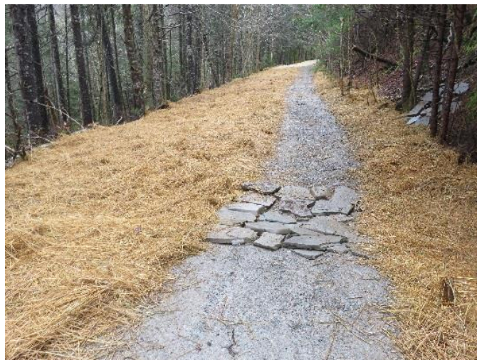
Figure 17: Exposed Area Covered with Straw Mulch
