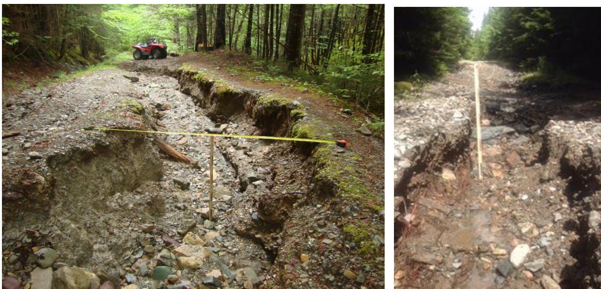
Figure 4: Erosion Just West of Second Mile Brook Bridge, 2015
