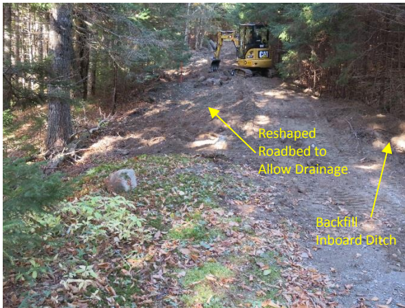
Figure 12: Backfill Inboard Ditch and Reshape Slope to Restored Natural Drainage Pattern
