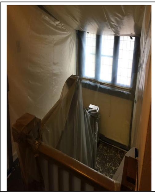
Figure 20: Stairway Containment Set Up
