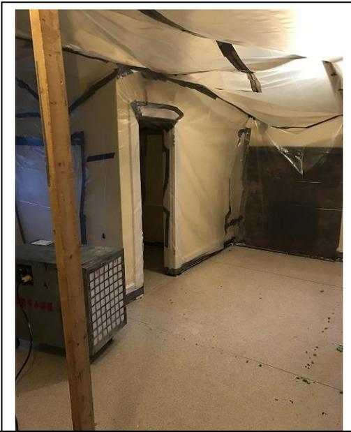
Figure 24: Rec Room Containment Set Up
