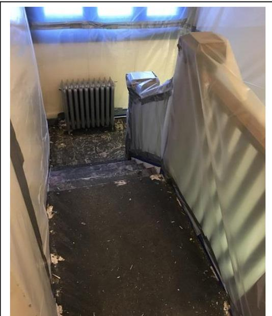
Figure 19: Stairway Containment Set Up
