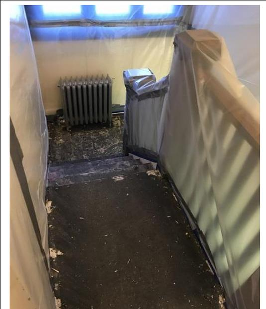
Figure 19: Stairway Containment Set Up
