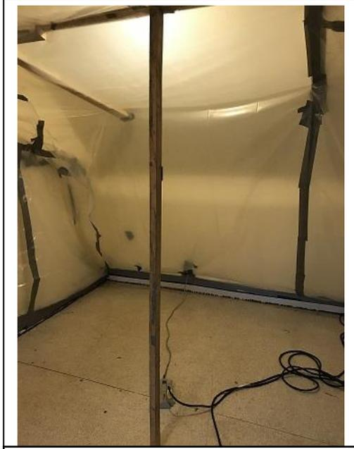
Figure 22: Rec Room Containment Set Up
