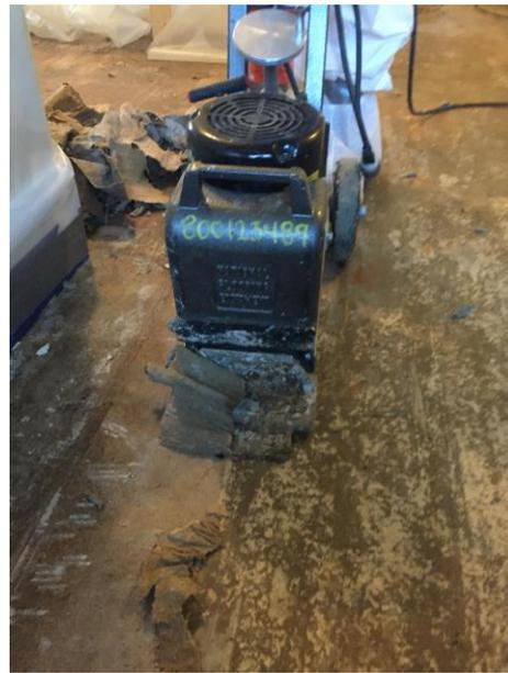
Figure 26: Removal of Paper Backing
