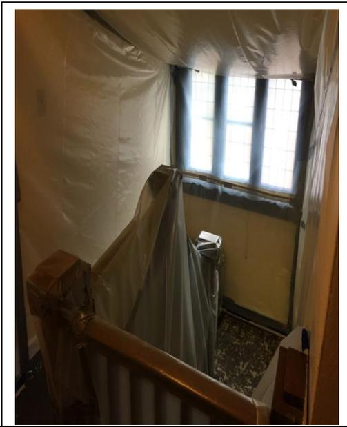
Figure 20: Stairway Containment Set Up
