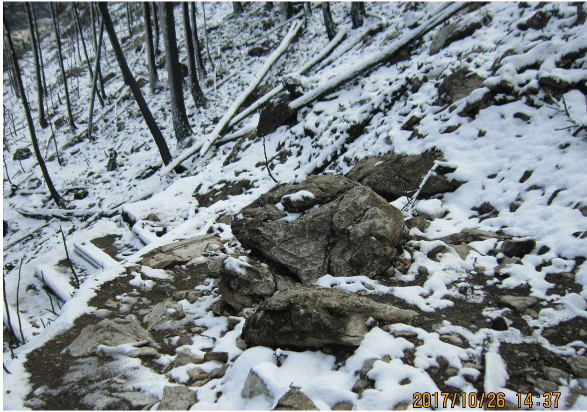
SWITCHBACK WITH A LARGE ROCK OUTCROP WITHIN THE UPPER AREA OF SWITCHBACK. ROCK SHALL REMAIN AS IS AND BE INCORPORATED WITHIN THE NEW LEVEL SURFACE AREA OF SWITCHBACK
