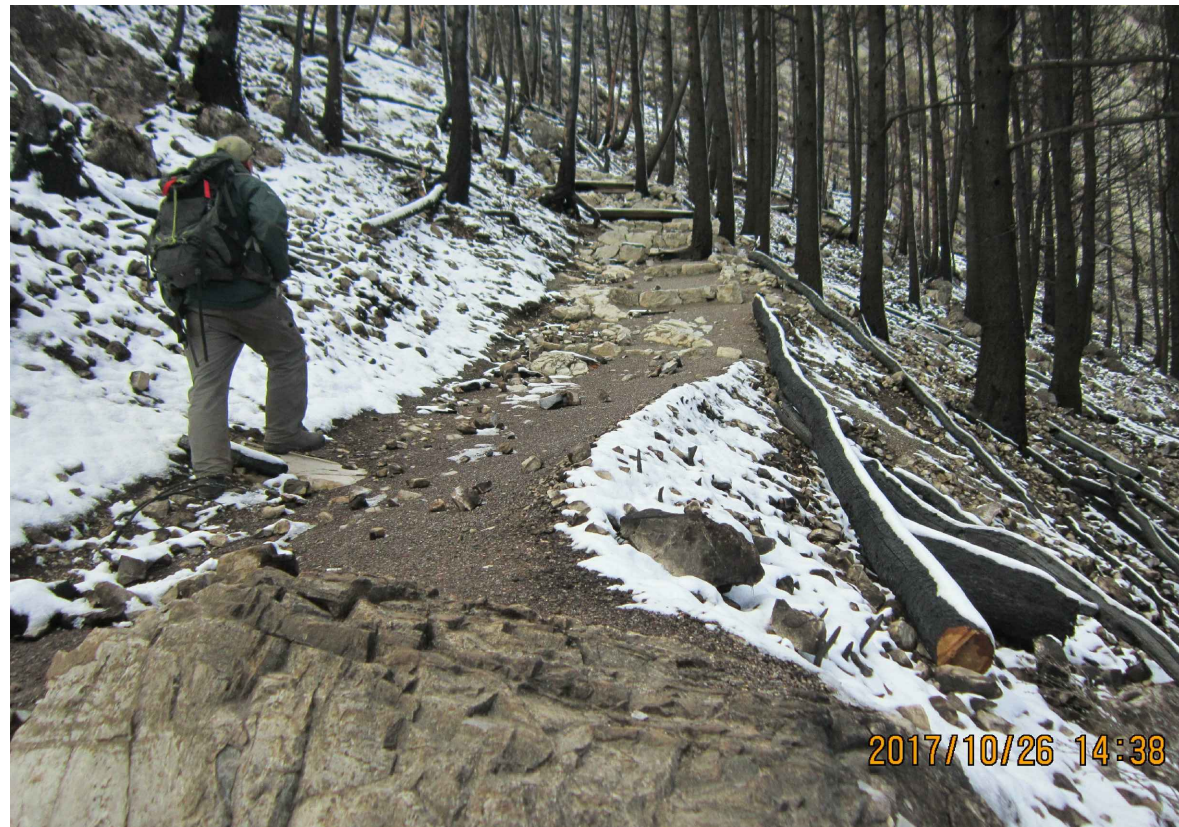
TRAIL LOOKING UPHILL AT THE SITE OF THE EXISTING LARGE ROCK IN TRAIL. INSTALL A NEW DRAINAGE SWALE BESIDE THE ROCK OUTCROP AND IMPROVE TRAIL
