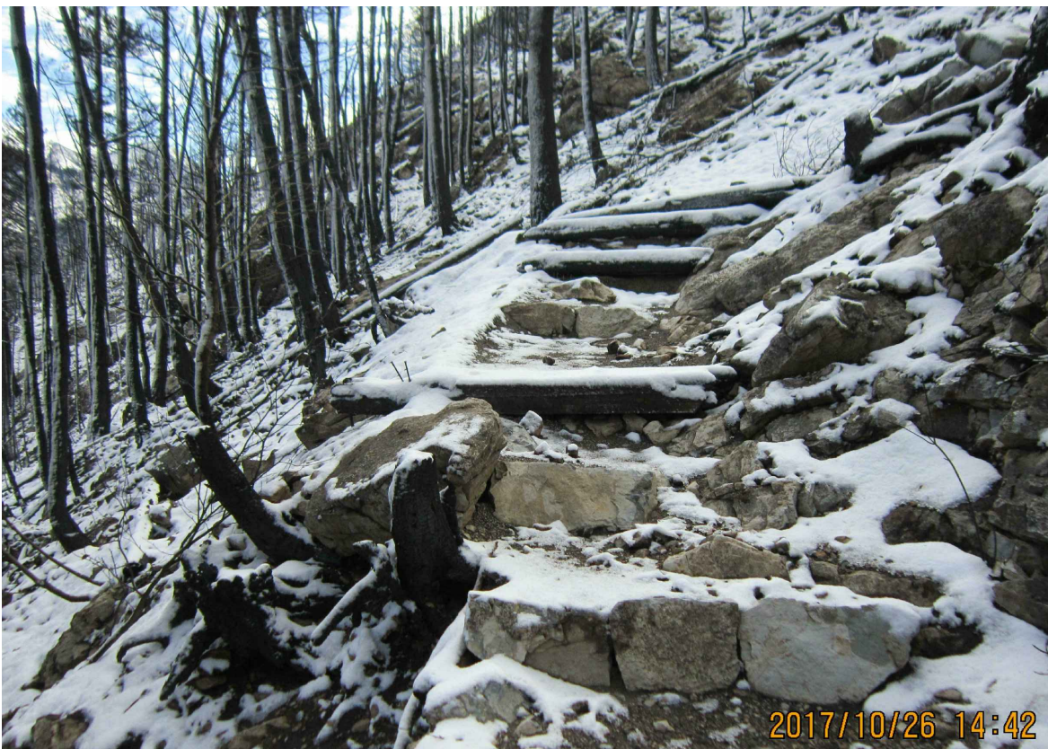
TRAIL AFTER SWITCHBACK AREA - GRADE AND PREPARE TRAIL FOR NEW ROCK WATER BAR STEPS. INSTALL ROCK EDGING AS REQUIRED.
