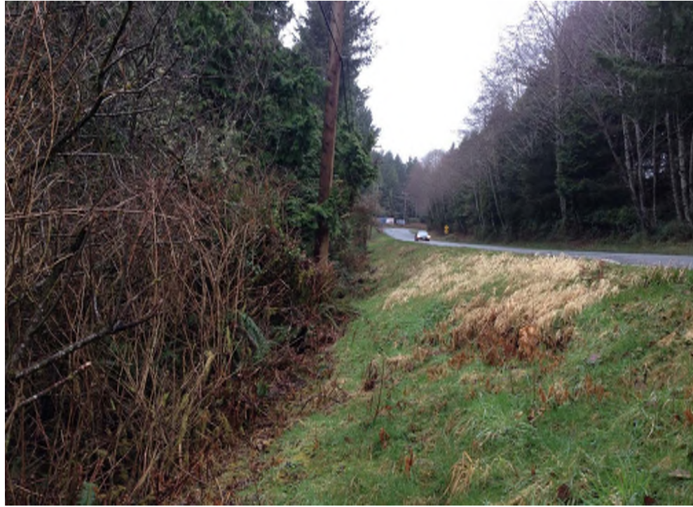
Photo 5: Road embankment slope south of BH14-01 (11 February 2014)
