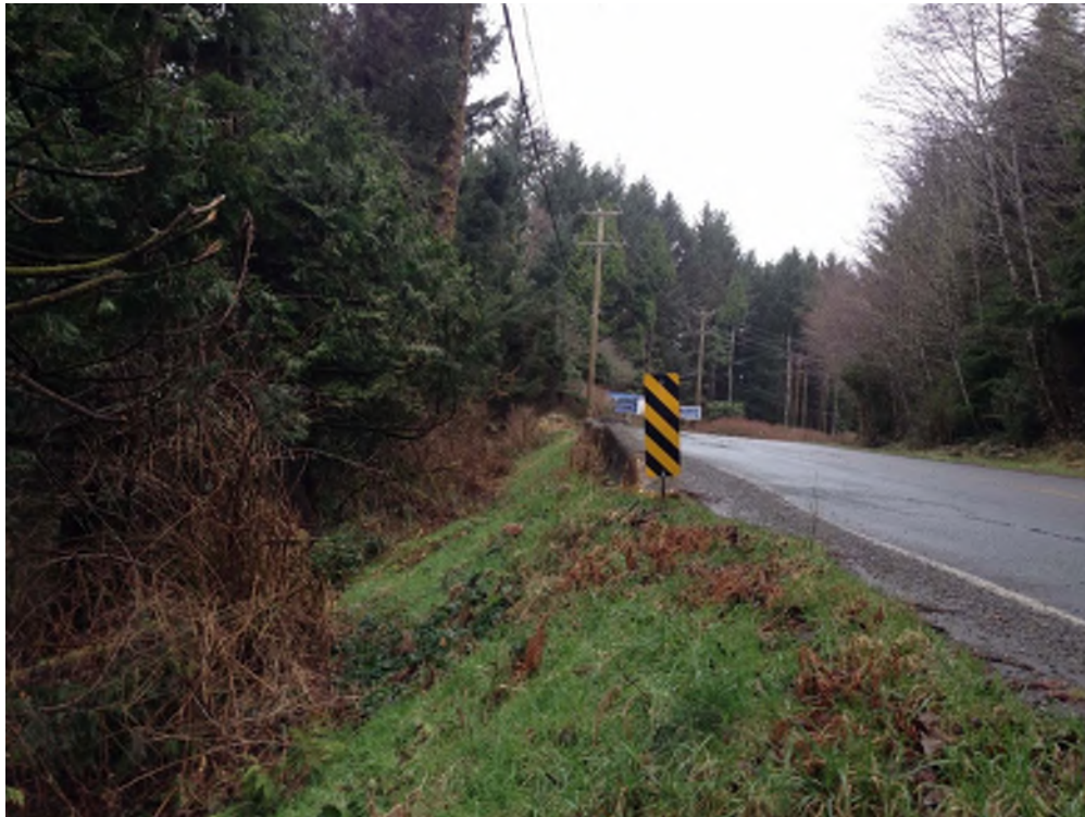
Photo 3: Road embankment slope south of BH14-01 (11 February 2014)
