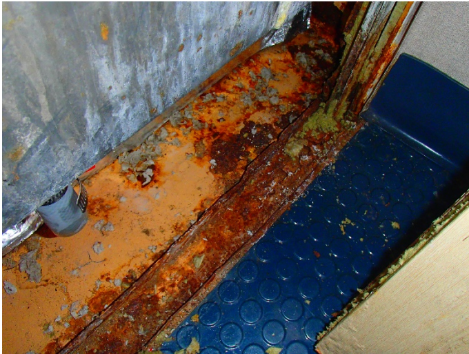
Figure 31: Corroded tracking & deck below sliding window
