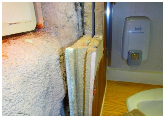
Figure 29: Typical 50mm (2'') Joiner panel
