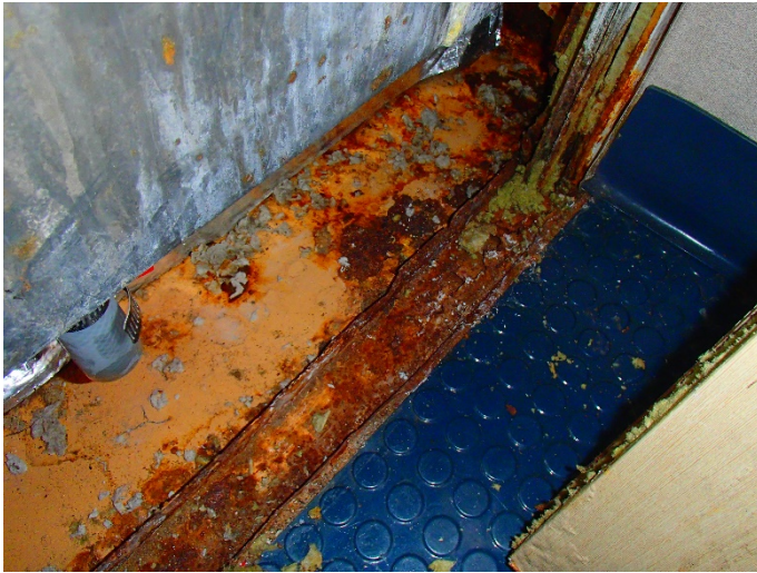
Figure 31: Corroded tracking & deck below sliding window
