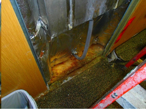
Figure33: Flexible hose connection under reservoir
