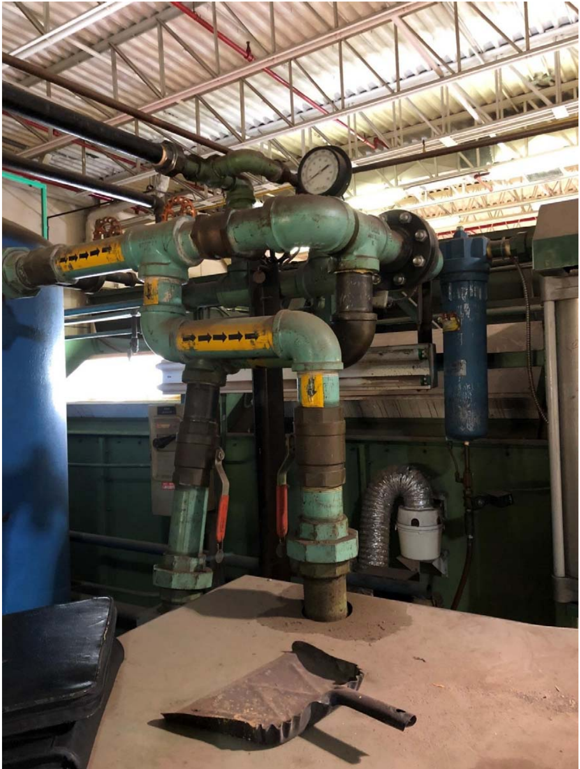
Figure 2: Unlabeled view of flange tie in with more of Air Receiver Tank visible
