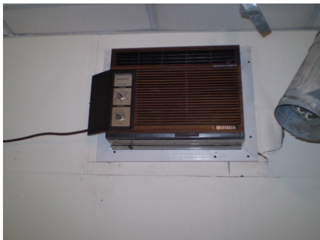
Photograph 45: Potential ODS containing air conditioning unit located in the portable located to the east of the Friar Tuck building.
