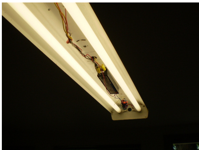
Photograph 3: Mercury-containing fluorescent light fixture.
