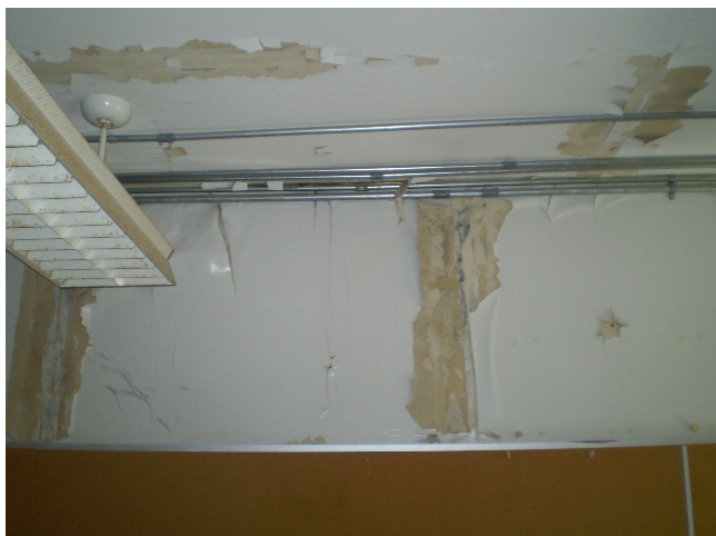
Photograph 19: Cracked and peeling paint in the southern portion of the cooper dome.
