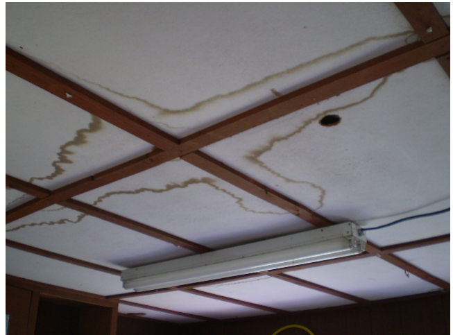
Photograph 18: Water staining observed in the camp craft building.
