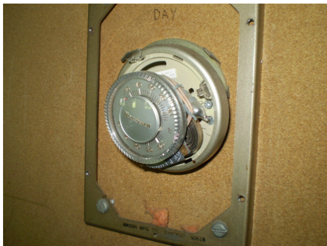
Photograph 2: Mercury-containing thermostat located in the Arts and Crafts building.
