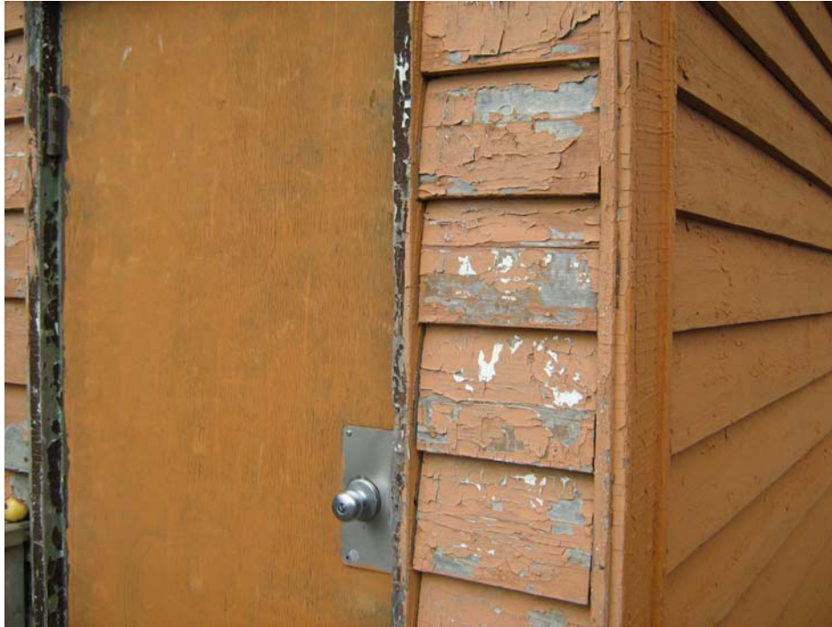
Photograph No. 3: Location of lead-based paint sample 614110-CS3 on --- of program building
