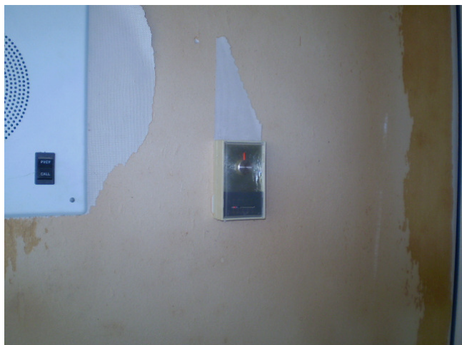
Photograph 44: Potential mercury-containing thermostat located in the Friar Tuck building.
