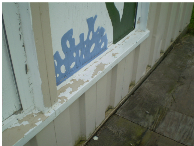
Photograph 46: Cracking and peeling paint located on the window sill of the portable to the east of the Friar Tuck building.
