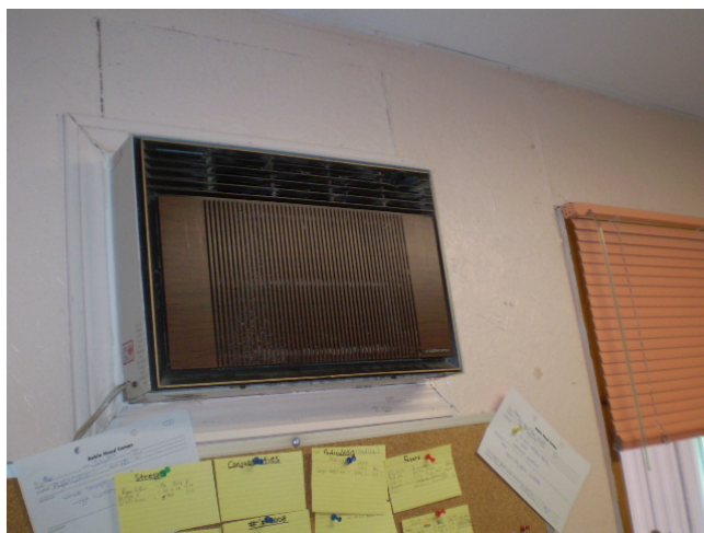
Photograph 4: Window mounted air conditioning (potential ODS) unit located in the main office.
