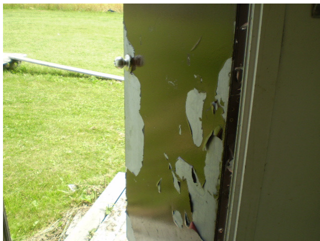
Photograph 20: Cracked and peeling door paint of the sports building.
