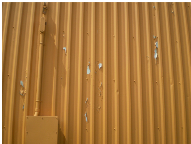
Photograph 47: Cracked and peeling exterior paint located on the Cooper Dome building.
