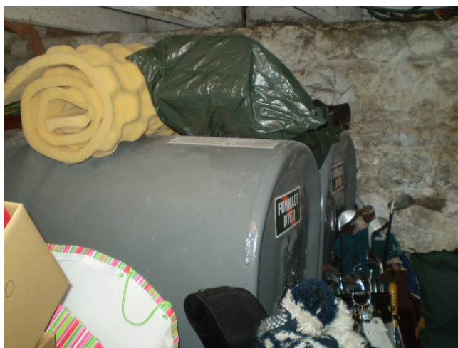
Photograph 6: Two ASTs located in the basement level of the south house.
