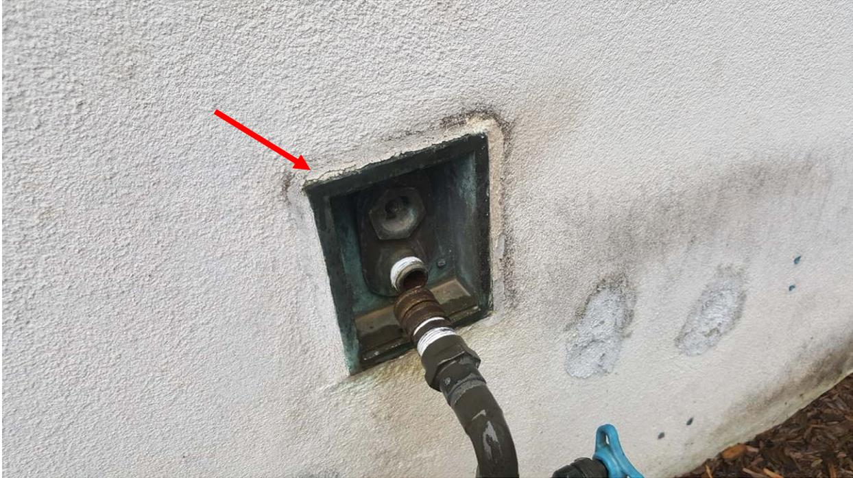
**Photo 2:** Non-friable white joint caulking located on exterior taps and outlets was found to contain 1% Chrysotile asbestos (DST Sample 31268-05B).
