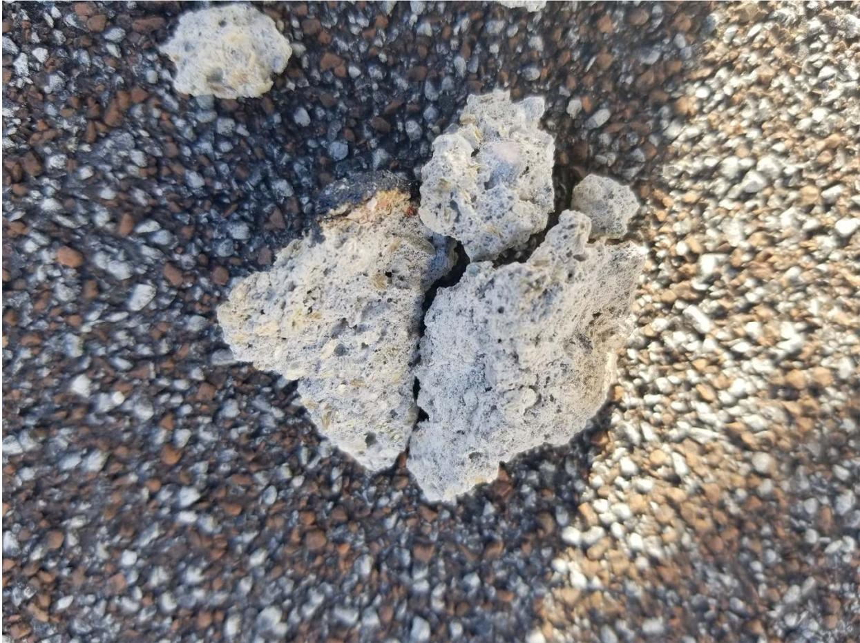
**Photo 5:** Non-friable cementitious roof leveling compound, located under existing roofing materials from Block 1 was confirmed to contain 1% Tremolite asbestos (DST Sample 31268-15A).
