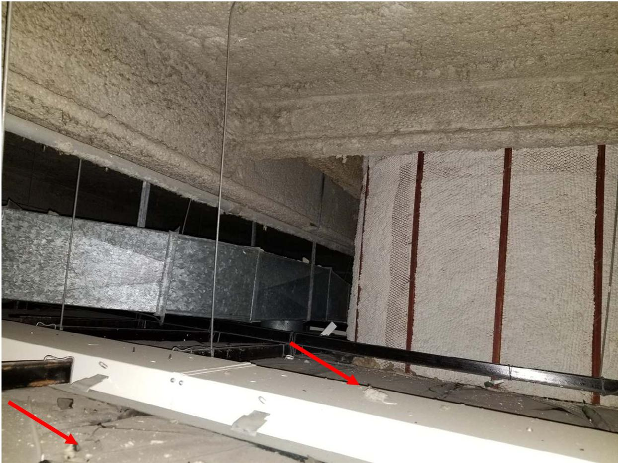
**Photo 4:** Asbestos-containing fireproof debris was observed on the suspended ceiling throughout Room E123.
