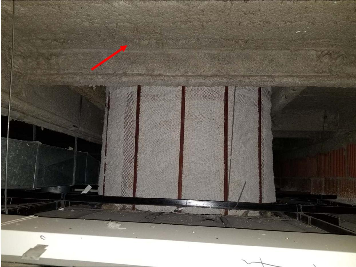
**Photo 3:** Friable spray on fireproofing, located on the deck above the suspended ceiling of Room E123 was confirmed to contain 65% Amosite asbestos (DST Sample 31268-13A).
