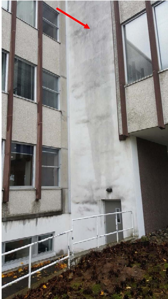
**Photograph 1:** Non-friable textured exterior cladding (both white and grey layers), located on the exterior of the building contain 1% Chrysotile asbestos respectively. (DST Sample 31268-01A).
