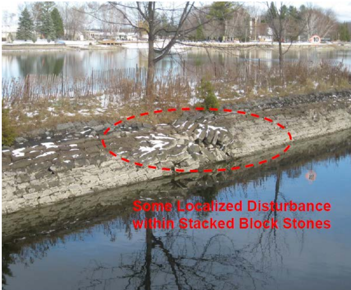
Figure 1. Slumped area of stacked stone.
