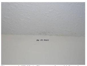
Photograph HMS 6: Close-up of mould Sample PN-R3-M001. Bathroom ceiling in Residence 3 (BU F/353).
