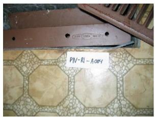
Photograph HMS 4: Close-up of asbestos Sample PN-R1-A004. Sheet flooring in Residence 1 (BU F/373 or F/375).
