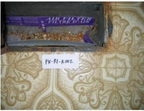
Photograph HMS 2: Close-up of asbestos Sample PN-R1-A002. Sheet flooring in Residence 1 (BU F/373 or F/375).
