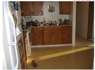
Photograph HMS 1: Asbestos Sample PN-R1-A002. Sheet flooring in Residence 1 (BU F/373 or F/375).
