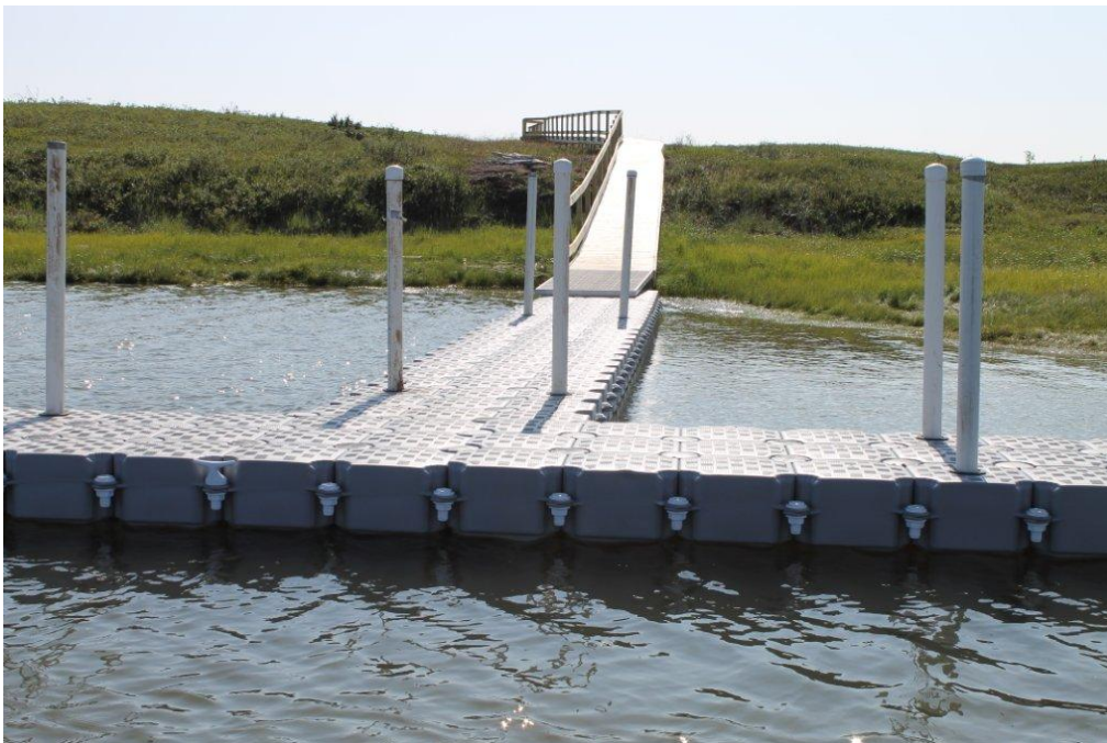
Photo 2: Boardwalk and dock
