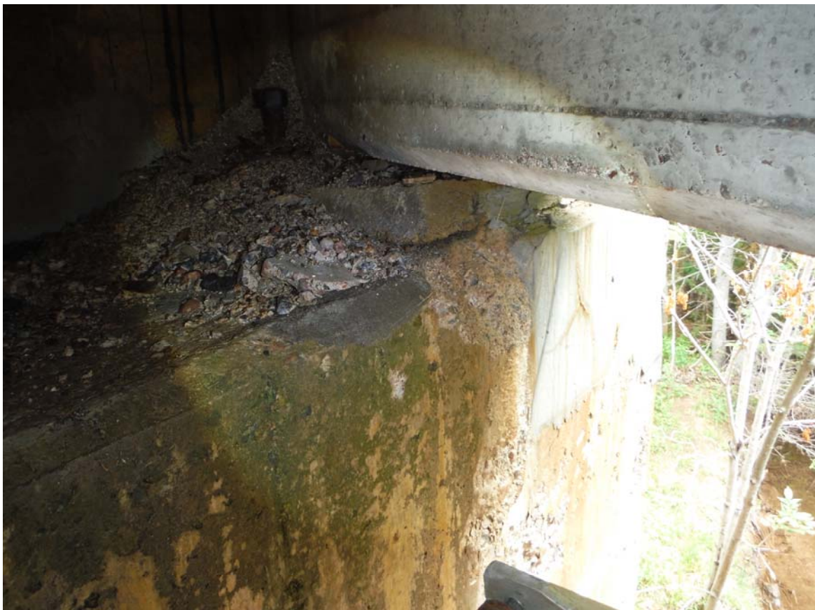
East Abutment Bearings – Medium spall beneath bearing block of South most girder (Poor). Note debris.
