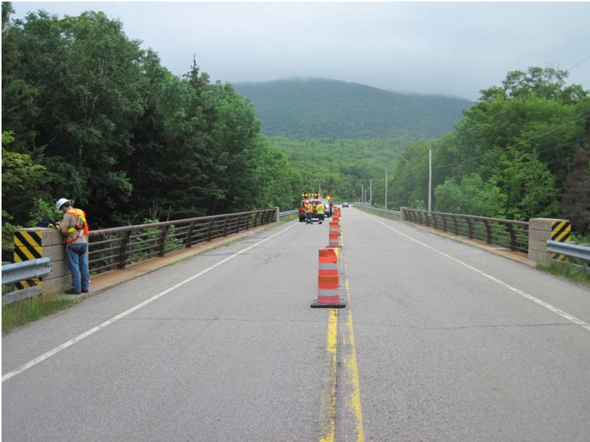
View of East approach, looking West. Note medium transverse crack (Fair) and light wheel track rutting (Good).
