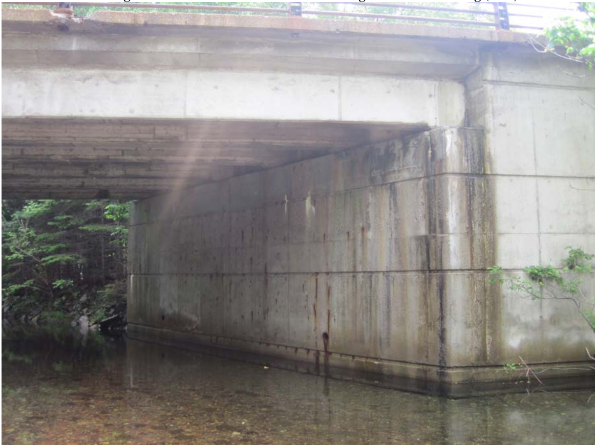
NW Wingwall – Active water run-off from bearings with dark staining (Fair)
