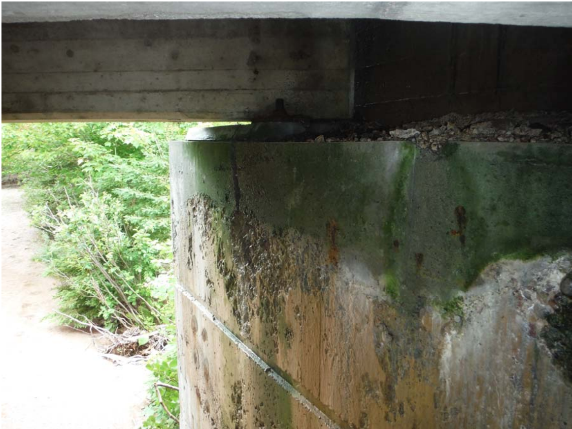
West Abutment Wall – Local area of severe scaling (Poor) below repair to bearing area
