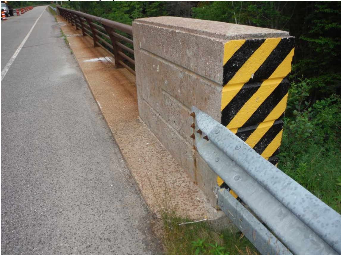
Deck Wearing Surface – Signs of water ponding at North side curb of deck. Appears worst at mid-span due to long-term deflection of concrete beams and re-asphalting.
