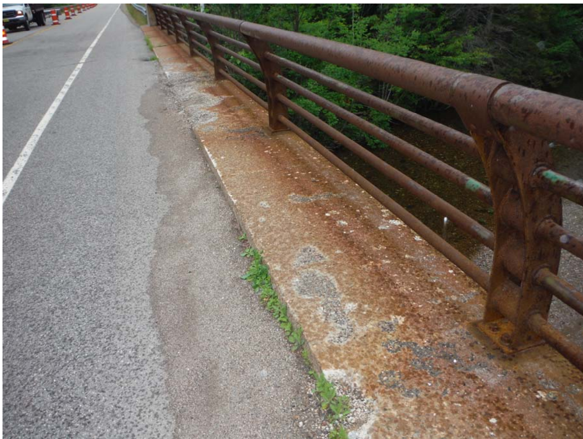
Curb, North side – Medium Disintegration near mid-span of bridge (Fair), likely caused by water ponding and frost action. Rust staining of curb caused by run-off from rails.
