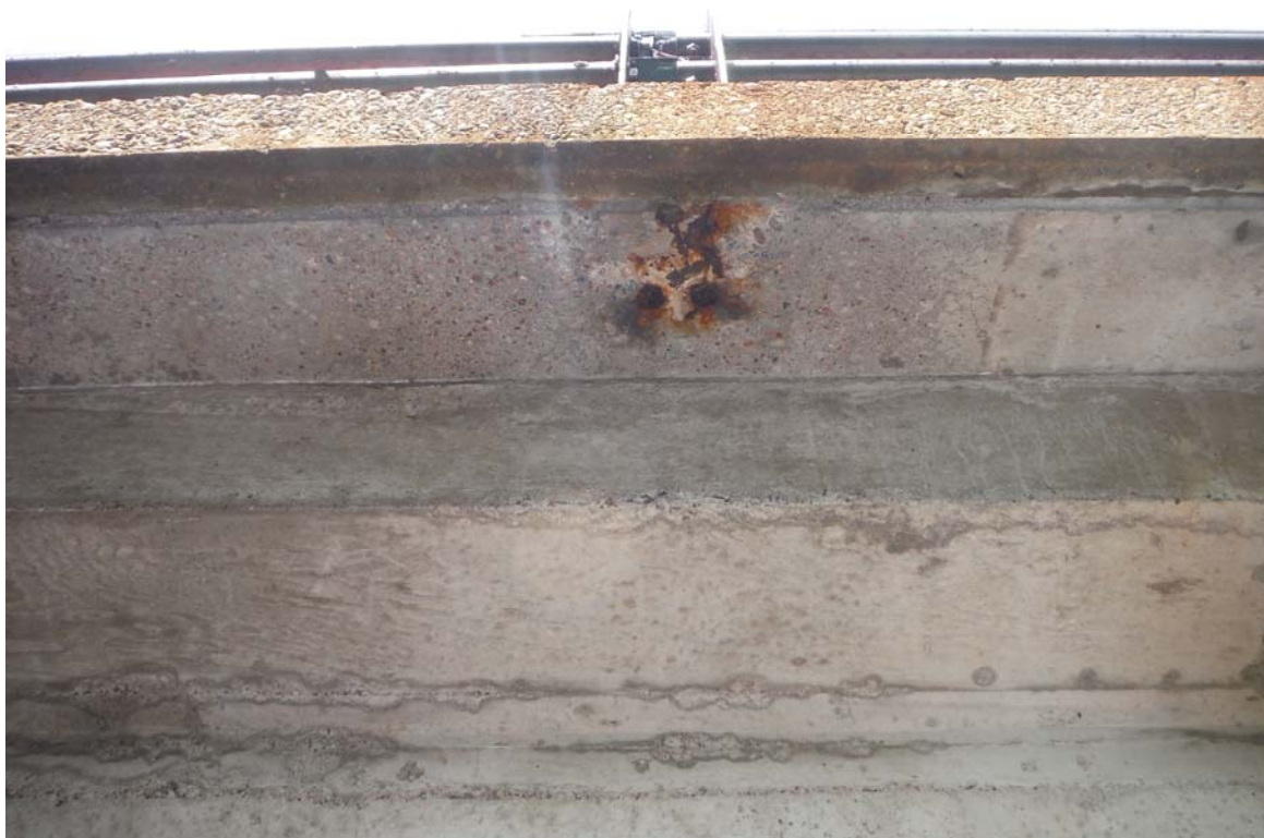
Railings– Typical severe corrosion of anchor bolt heads (Poor). Light spalls in concrete
