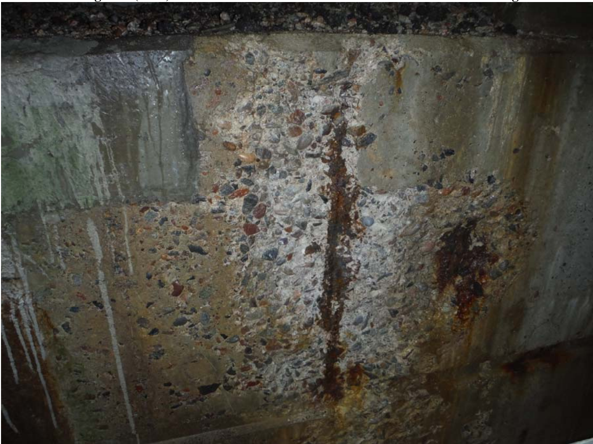
East Abutment Wall – Local area of spalling (Poor) with medium corrosion of reinforcing steel (Poor)
