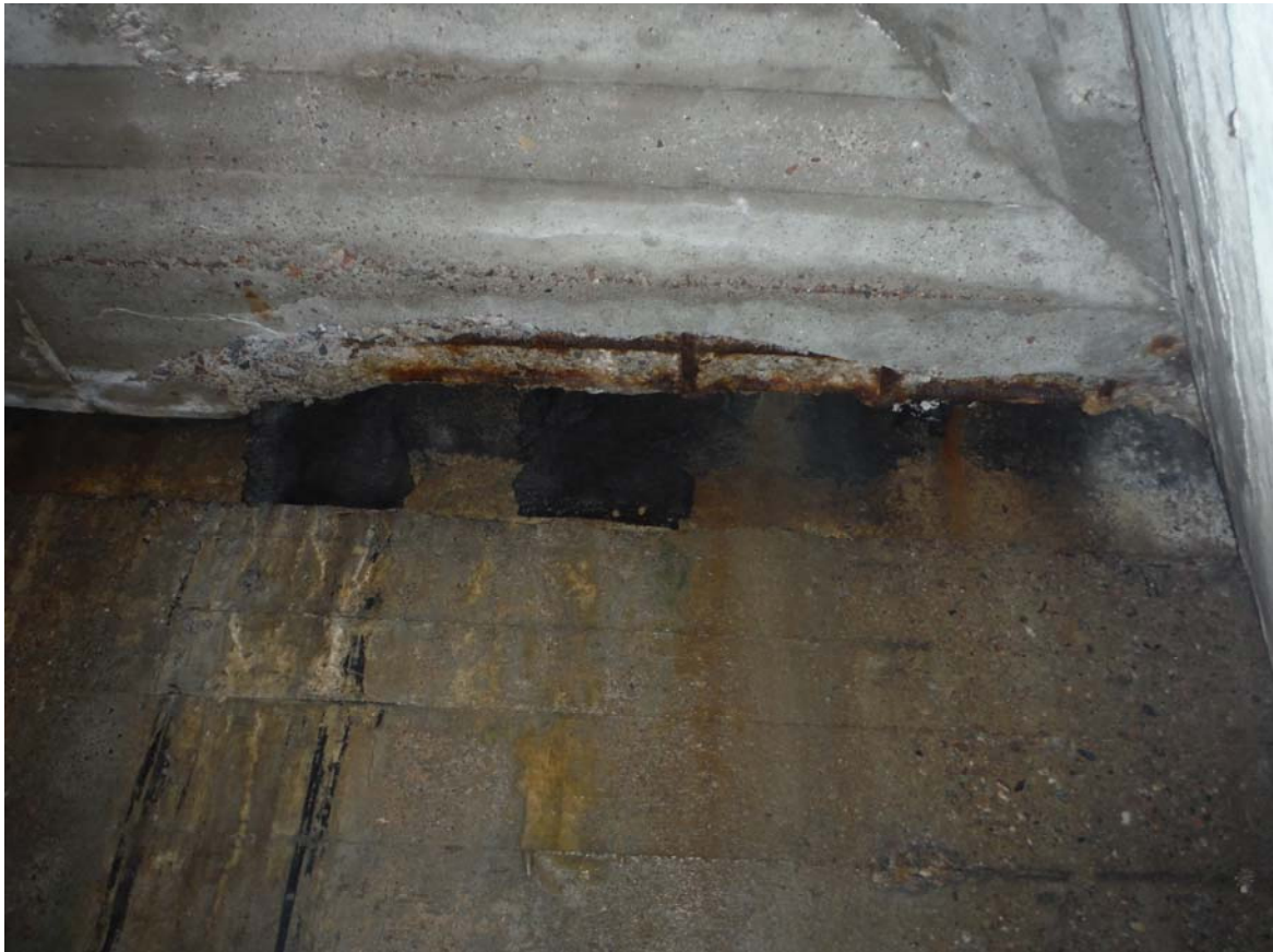
Deck Soffit – Severe spall in soffit of thickened deck edge at East abutment (Poor)
