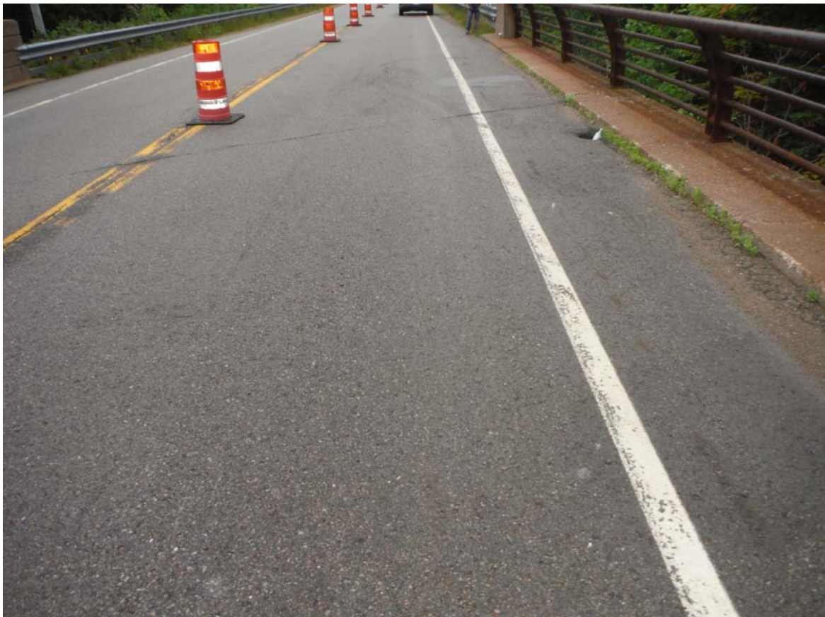
View of East approach, looking East. Diagonal crack directly above expansion joint.
