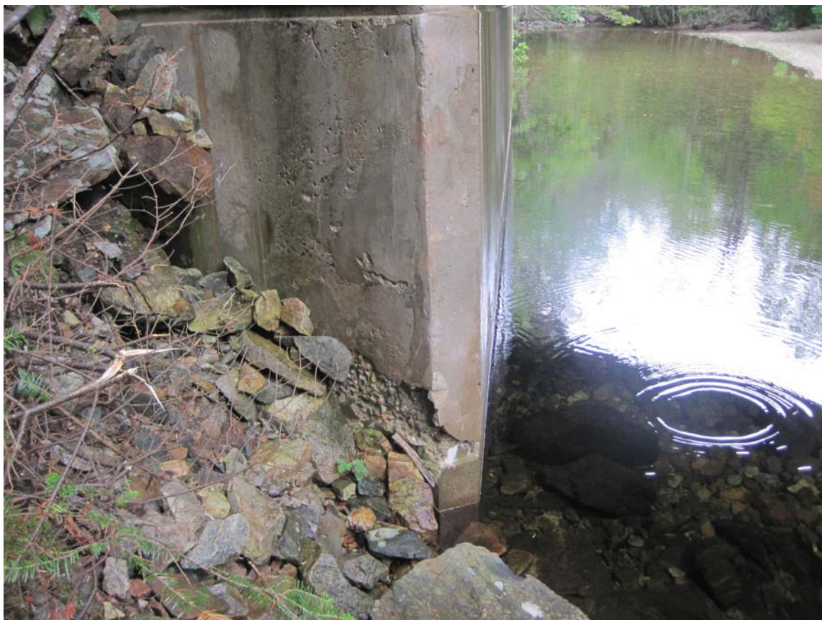
SW Wingwall – Medium spall likely caused by ice flow (Poor)
