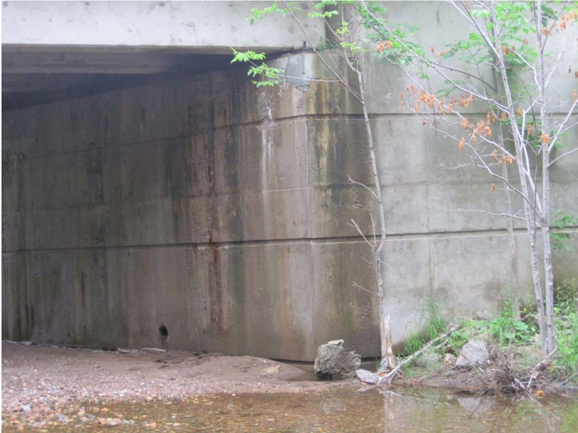
SE Wingwall - Active water run-off from bearings with dark staining (Fair)
