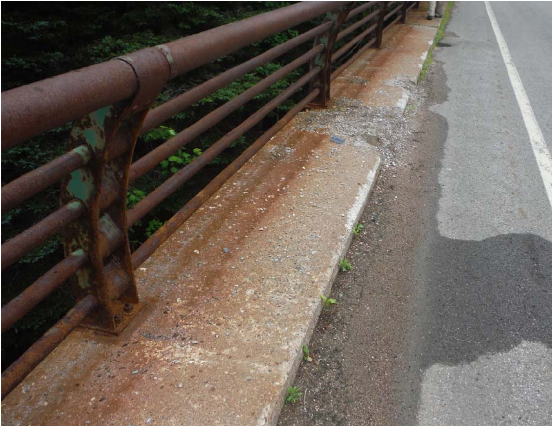
Coating system of railing – Paint system is fully compromised likely due to weathering and continued polymerization (Poor). Medium corrosion of railings and posts.
