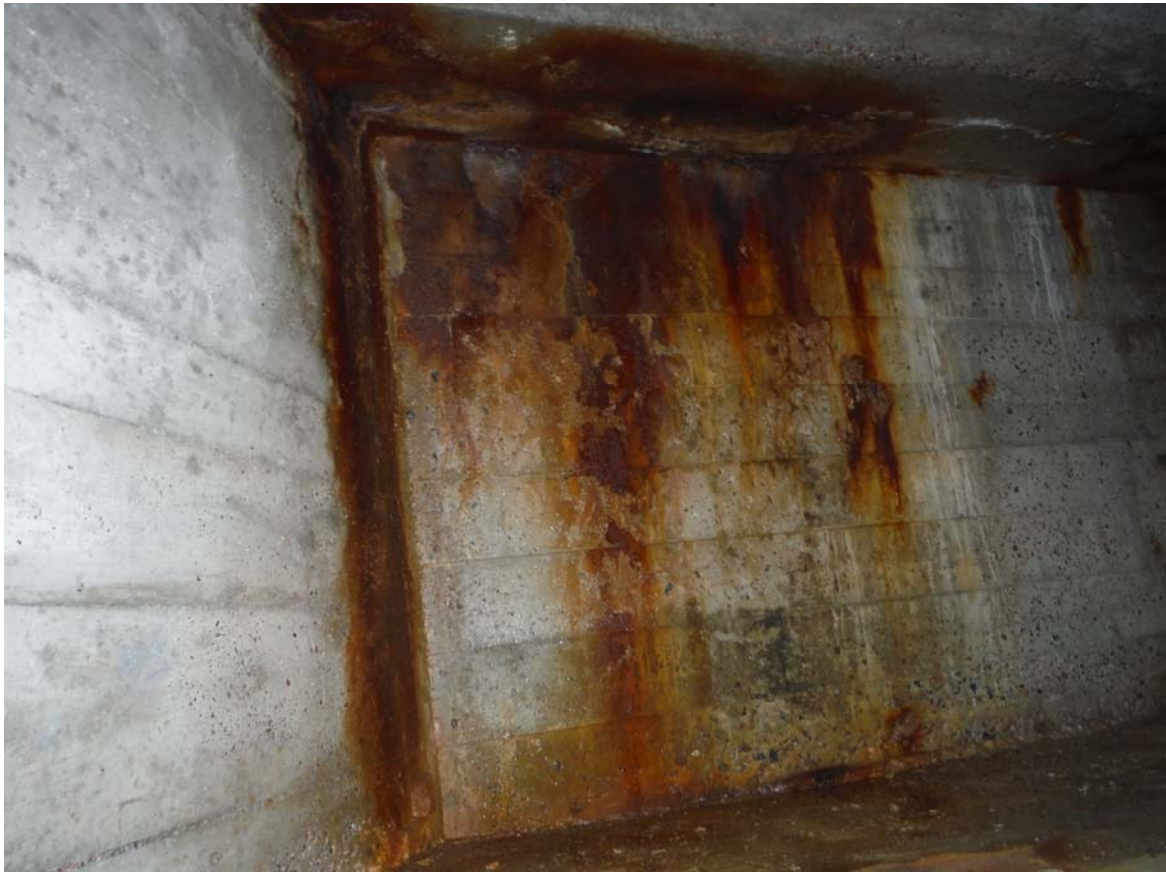
West Ballast Wall – Medium corrosion of reinforcing (Poor) with active wet area
