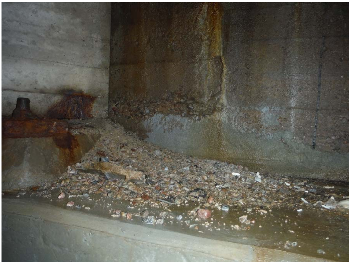
3 rd beam from North – Light spalling at bottom of East end of girder (Poor). Debris is from disintegration of deck soffit directly above beam.
