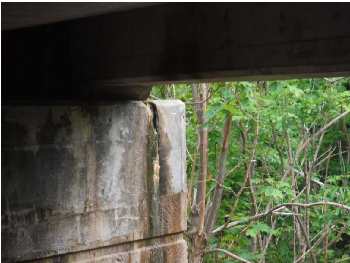
West Abutment Wall – Wide crack (Poor) with spalled portion and deposits caused by run-off from deck
