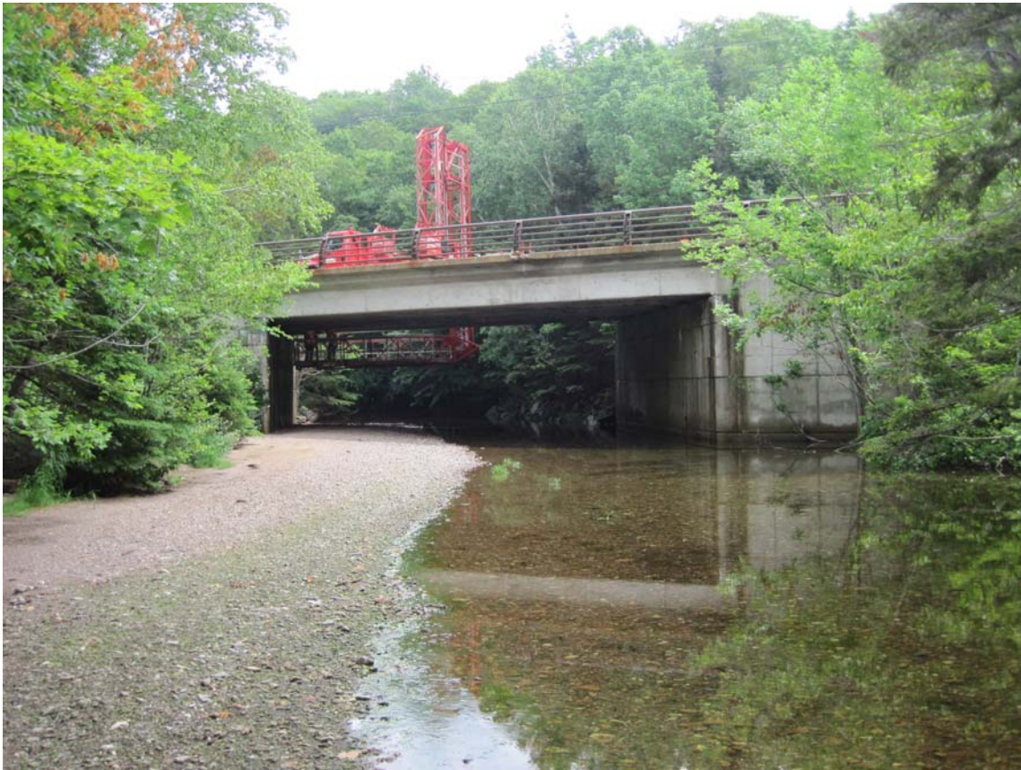
Waterway – Looking downstream (towards South). Aggradation in front of the East abutment and degradation at West abutment.
