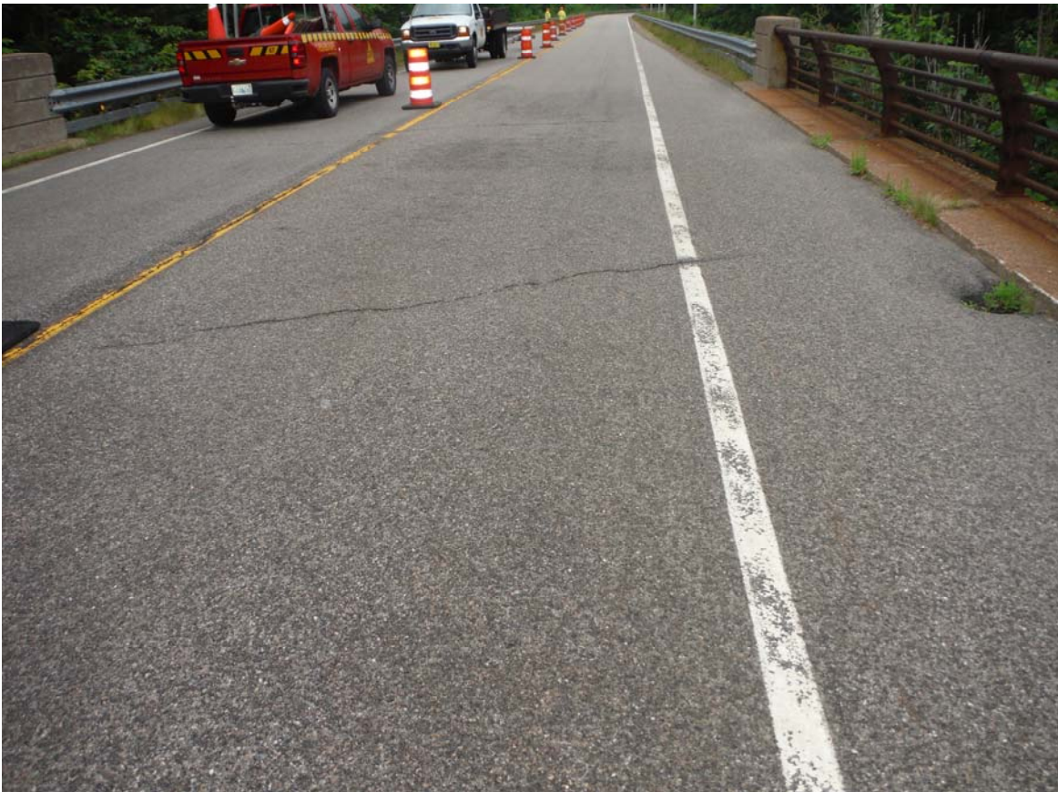
View of West approach, looking West. Diagonal crack directly above construction joint at fixed bearings.
