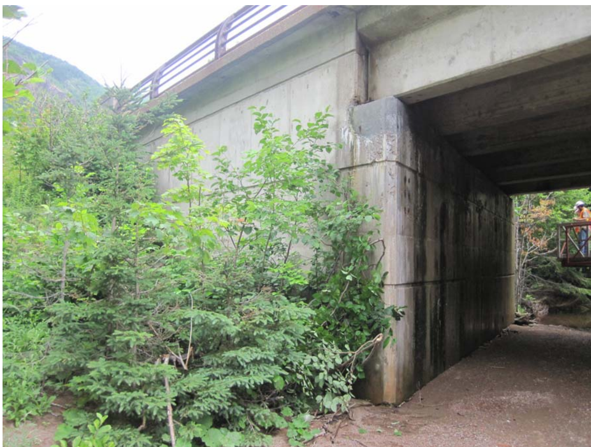
NE Wingwall – Active water run-off from bearings. Cracking with efflorescence below previous repair. (Fair)
