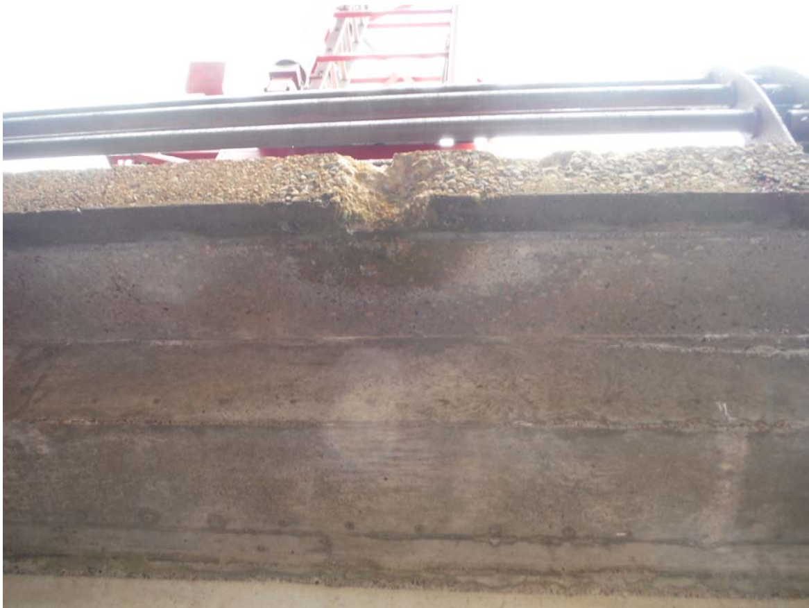
Deck Soffit/Curb – Severe scaling and disintegration of South side deck fascia (Poor)
