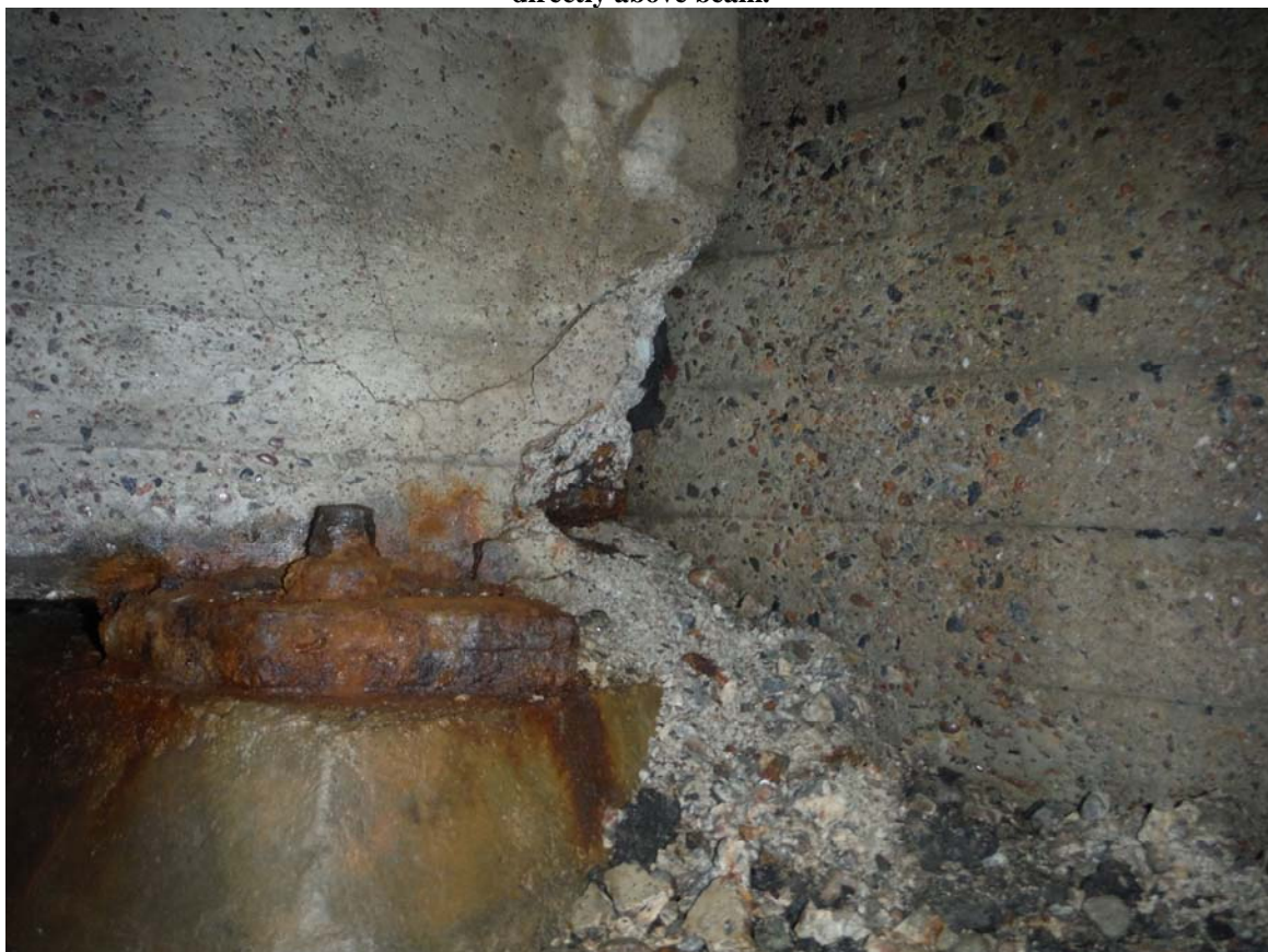
4 th beam from North – Severe disintegration of bottom end of beam at East abutment (Poor)
