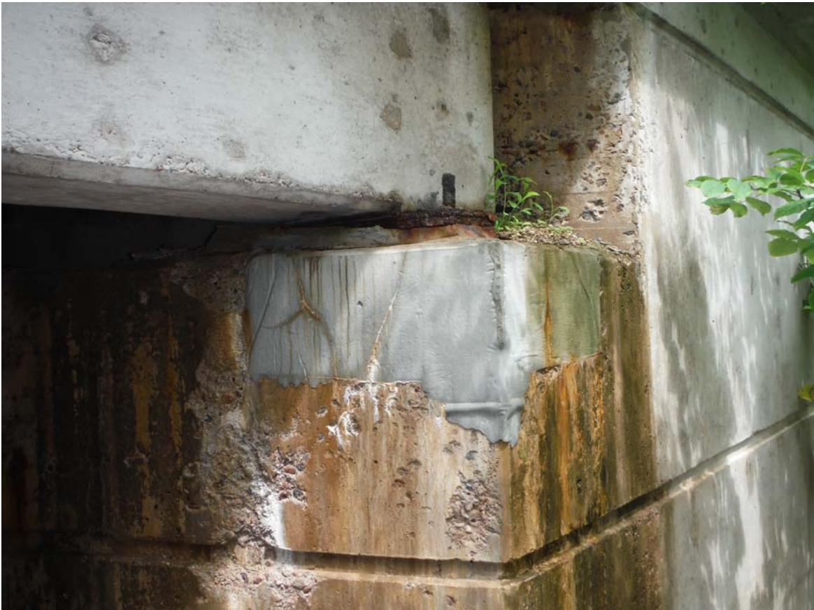
East Abutment Bearings – Medium cracks with leachate deposits through repair to bearing of South most girder (Fair). Missing nut at anchor bolt (Poor).
