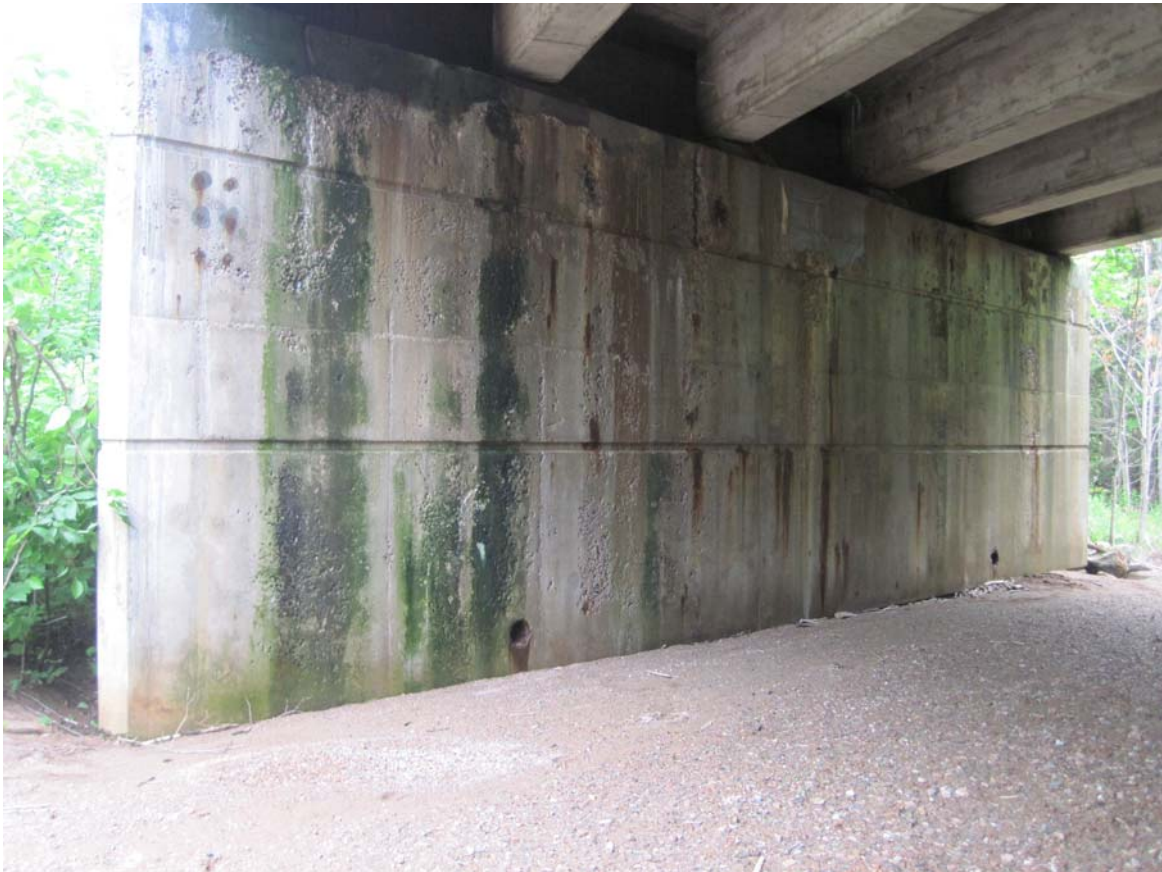
East Abutment Wall – Areas of medium scaling (Fair) with local spalls below bearings with medium corrosion of reinforcing steel (Poor). Note rust stains and indication of water run-off from bridge deck.
