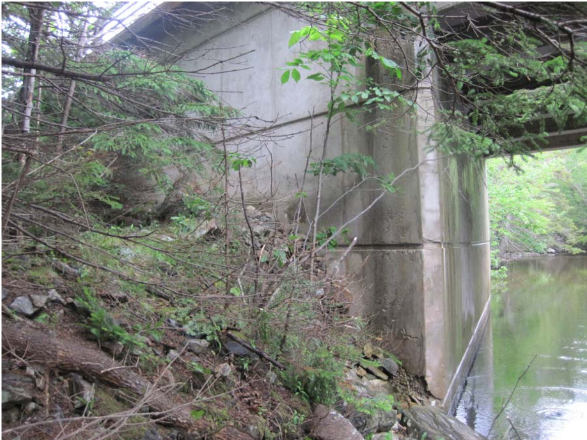
SW Wingwall – Active water run-off from bearings with dark staining (Fair)
