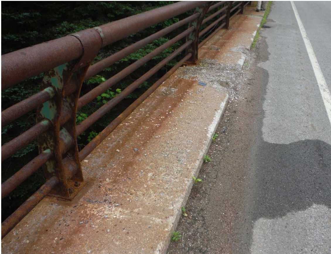
Curb, South side – Medium Disintegration near mid-span of bridge (Fair), likely caused by water ponding and frost action. Abrasions at exposed corner of curb, likely caused by snow plow.
