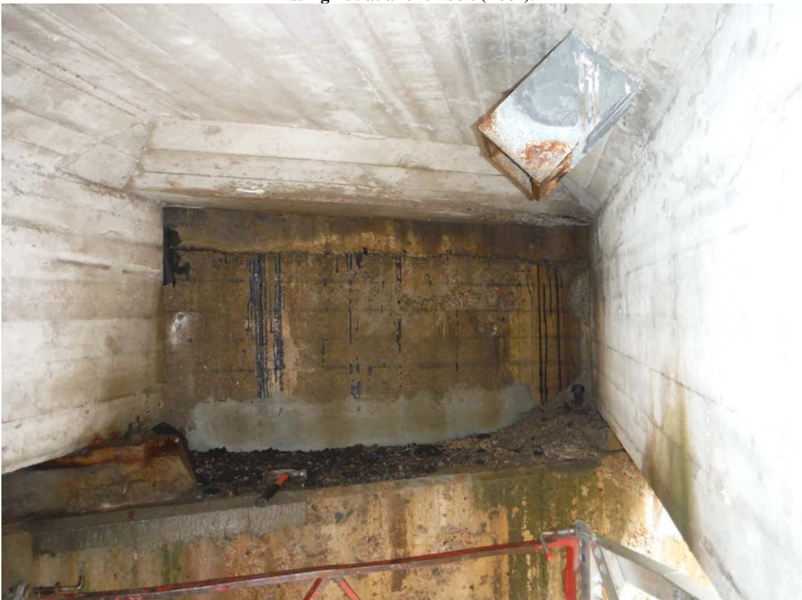
East Abutment Bearings – Proximity of deck drain to bearings. Accumulation of debris on top of abutment wall
