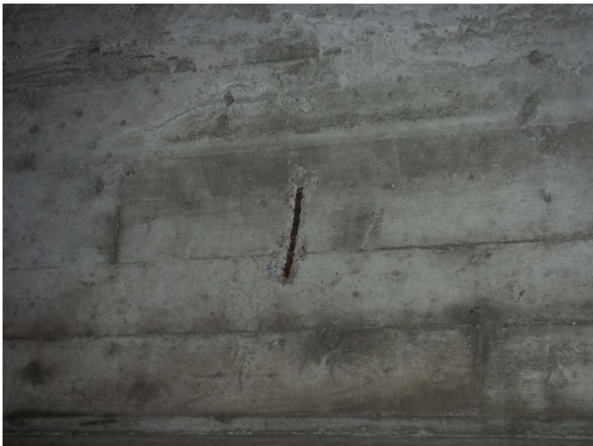
2 nd beam from North – Light spalling on vertical face with medium corrosion of reinforcement (Poor)
