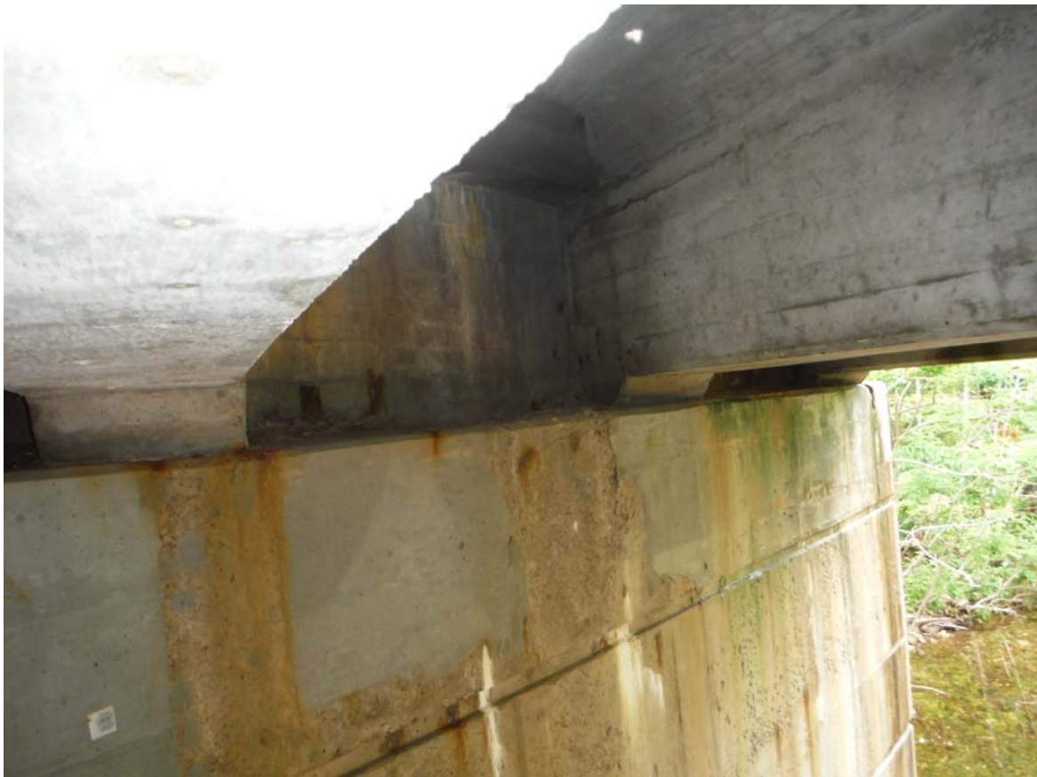
West Abutment – Fixed bearings condition provided by anchors bolt dowels
