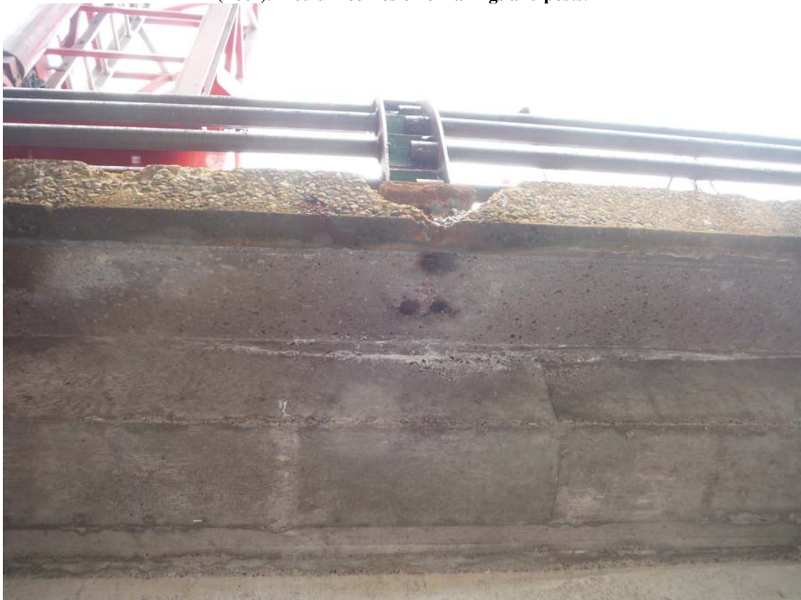
Deck Soffit/Curb – Spalling and severe disintegration at South side fascia (Poor). Railing compromised
