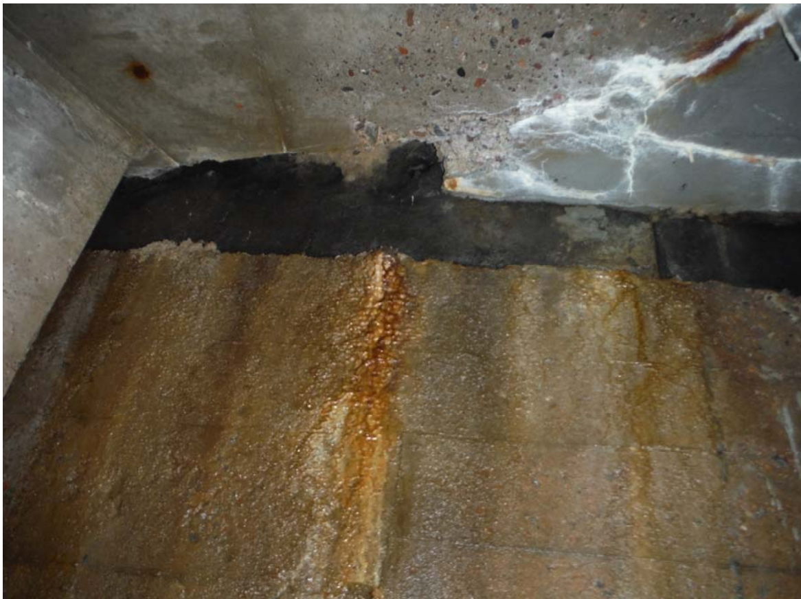
East Ballast Wall – Active wet area with leachate deposits on soffit (Poor)
