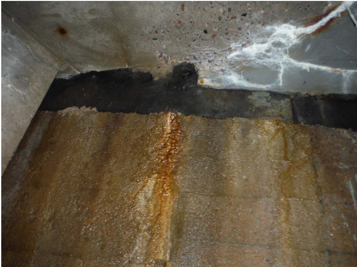
Deck Soffit – Severe spall in soffit of thickened deck edge at East abutment (Poor). Wide cracks with leaching at previously repaired area due to deterioration of old concrete.
