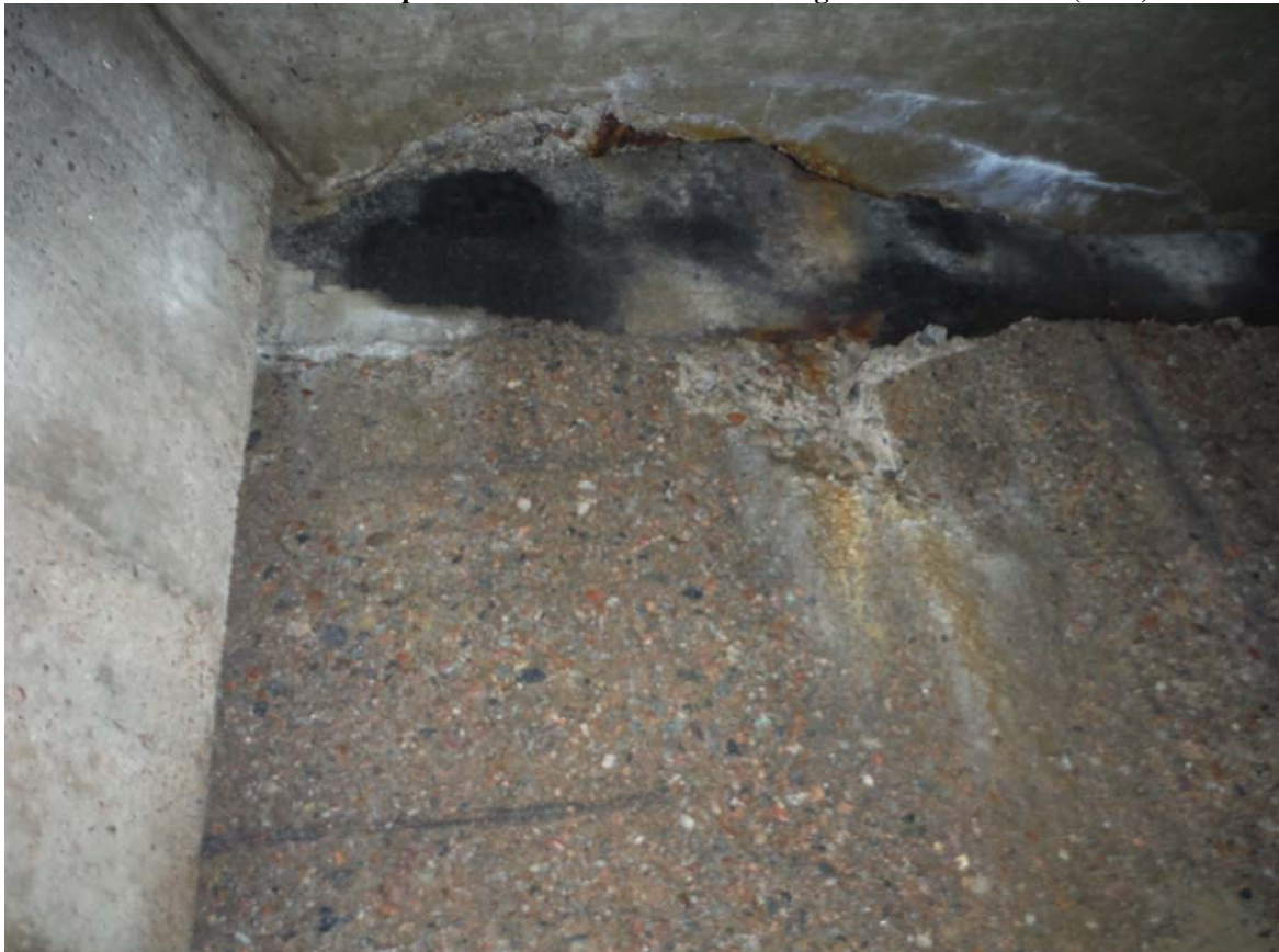
Deck Soffit – Severe spall in soffit of thickened deck edge at East abutment (Poor). Bond break paper has likely been dislodged during previous asphaltting.
