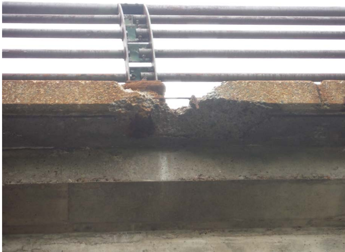
Deck Soffit/Curb – Very severe disintegration at North side deck fascia (Poor). Railing compromised.
