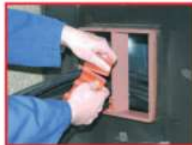
Check diameter of cables, select correct MIM and tear off your single IM if required...
