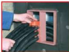
Use FB's or MFB's to fill up space for future installations.
