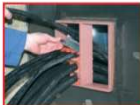
Anchor plates put between the module rows facilitate assembly and increase pressure tightness.
