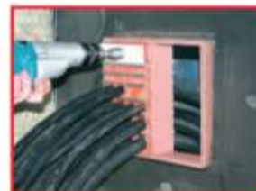
...tighten by ratchet handle or drilling machine.
