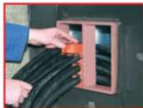
Use FB's or MFB's to fill up space for future installations.
