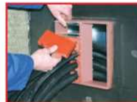
Put in last Anchor plate before inserting the last module row. Use also Fix Anchor if required.
