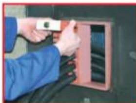
Push Wedge K-120 into the remaining space and...
