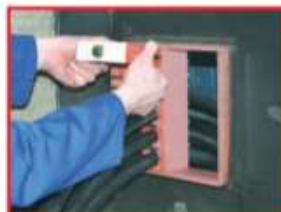
Push Wedge K-120 into the remaining space and...
