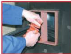
Check diameter of cables, select correct MIM and tear off your single IM if required...
