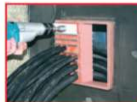
...tighten by ratchet handle or drilling machine.
