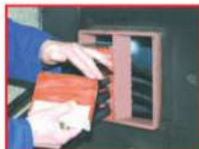
Grease Wedge Compression K-120 with bst Lubricant (grease also inner sides of wedges)
