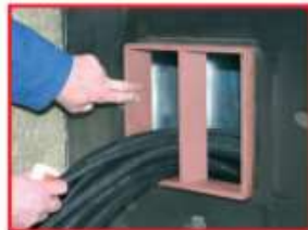
Grease inner surfaces of frame with bst Lubricant
