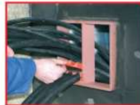
...or use original MIM and put it between the cables row by row.
