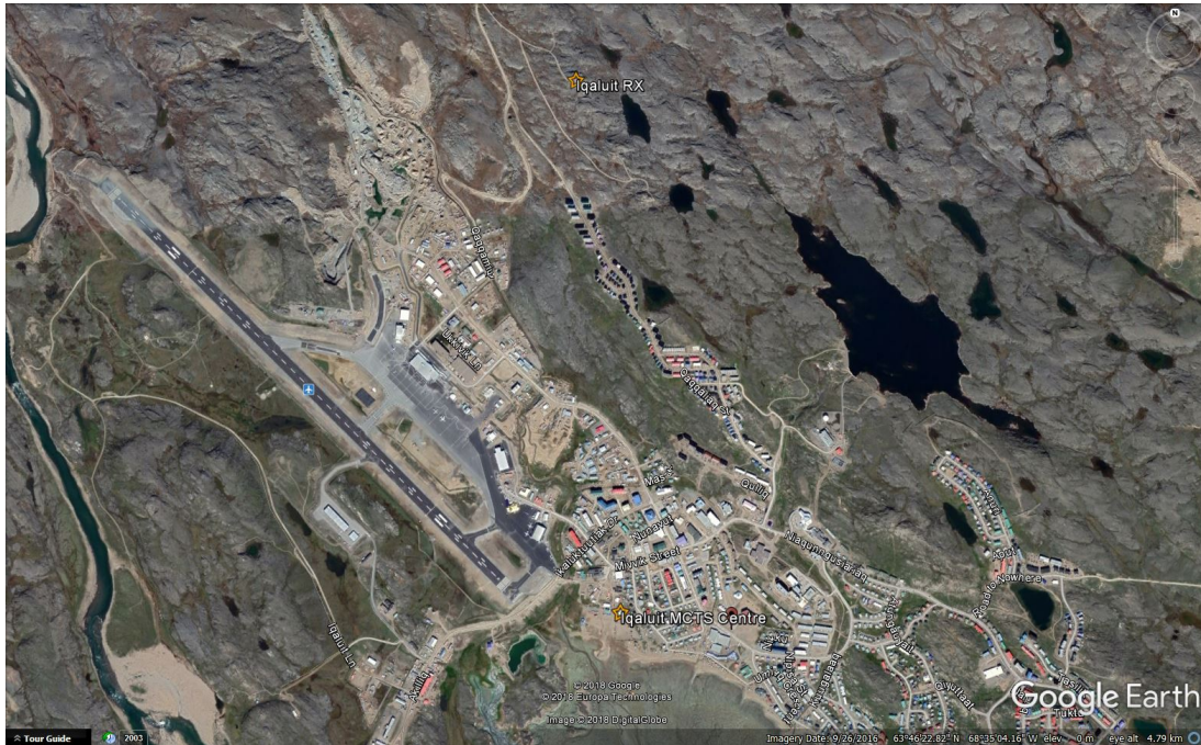
Figure 1: City Overview, Iqaluit, NU Note location of project site and staging location
