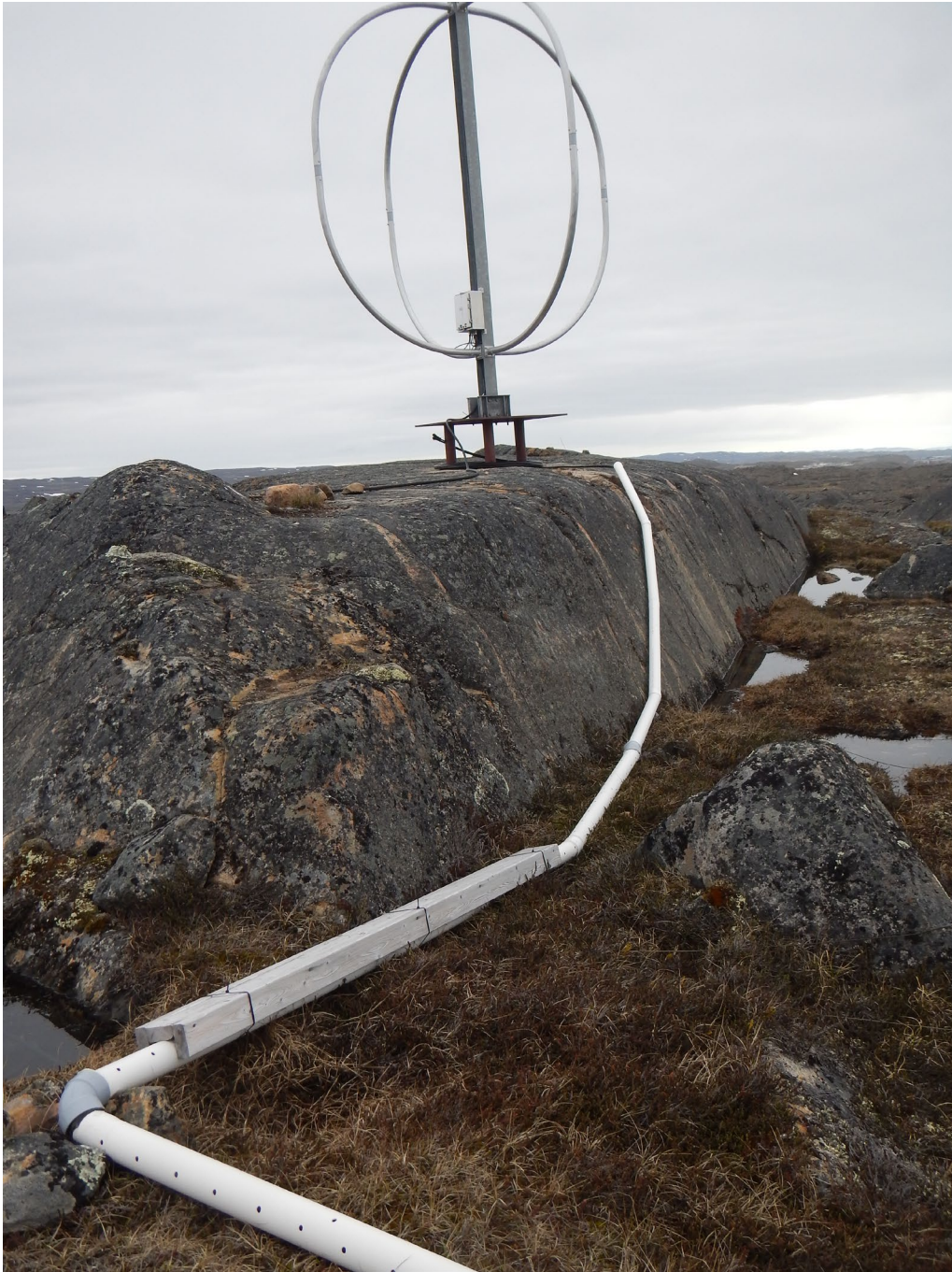
Figure 5: Existing conduit, note drain holes
